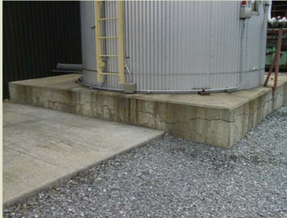
Concrete foundation of a storage tank in Hurt, Virginia constructed in 1993 (left). Close-up view of ASR-distressed concrete (right). Coarse aggregate is a granitic gneiss. Photo sent by Nick Scaglione, Concrete Research and Testing, LLC.
