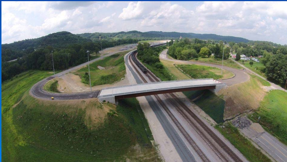
Prichard Intermodal Facility (TIGER III), Source: West Virginia DOT
