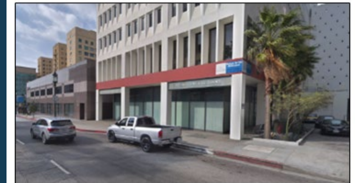
Recommendation 1A.1 Convert White Zone to Yellow Commercial Loading Zone (F) Source: Google Streetview
