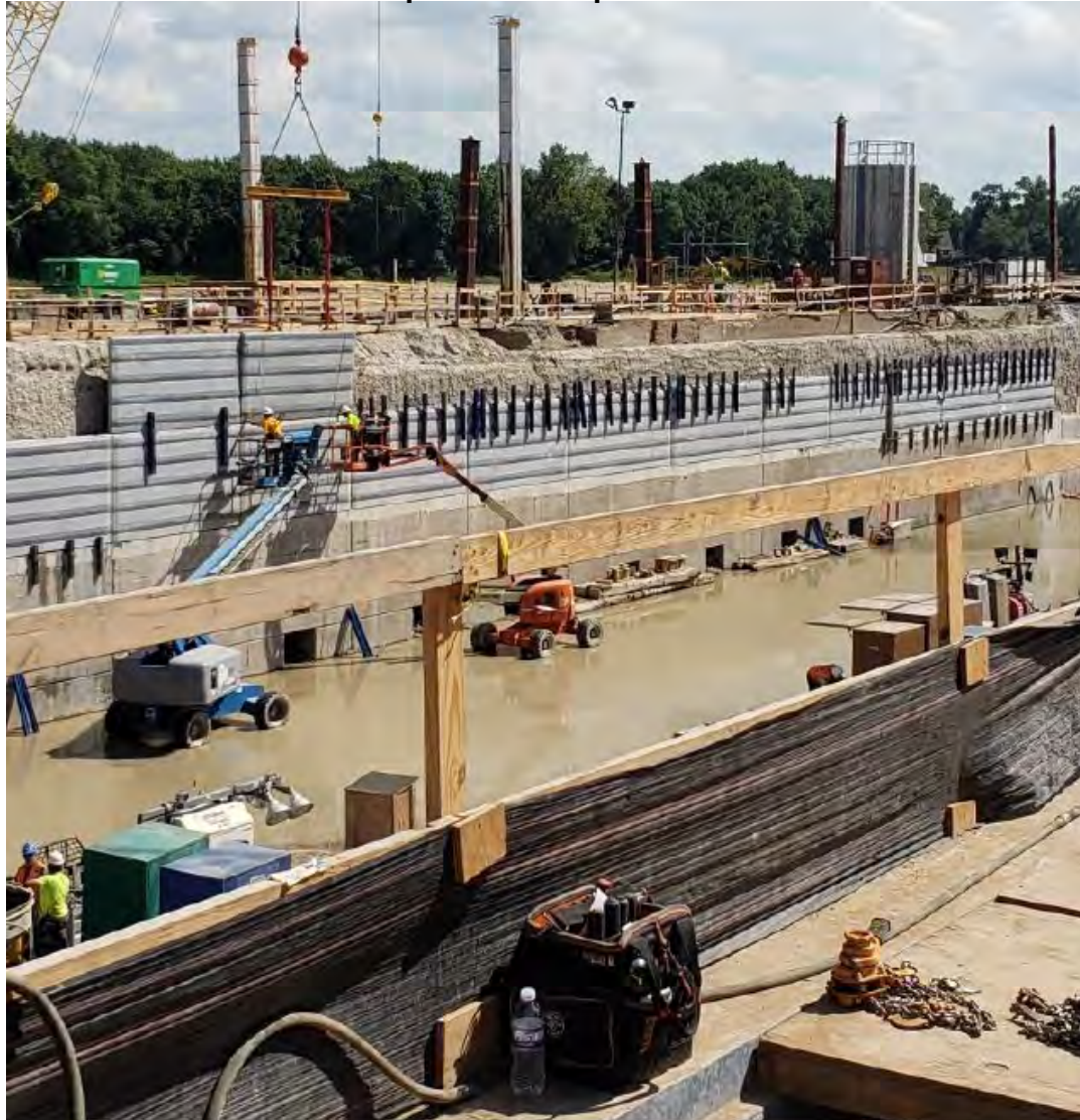
Vertical concrete pre-cast panel installation
