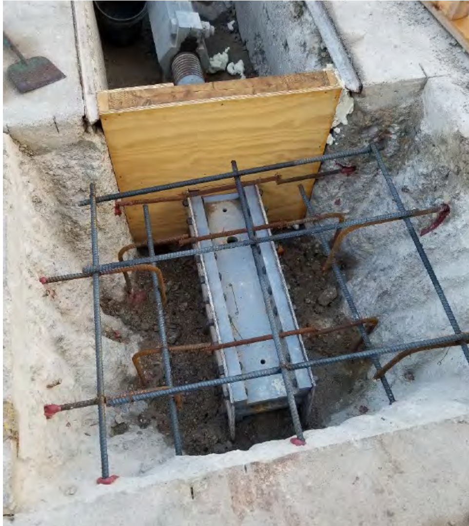
Miter gate anchorage repairs
