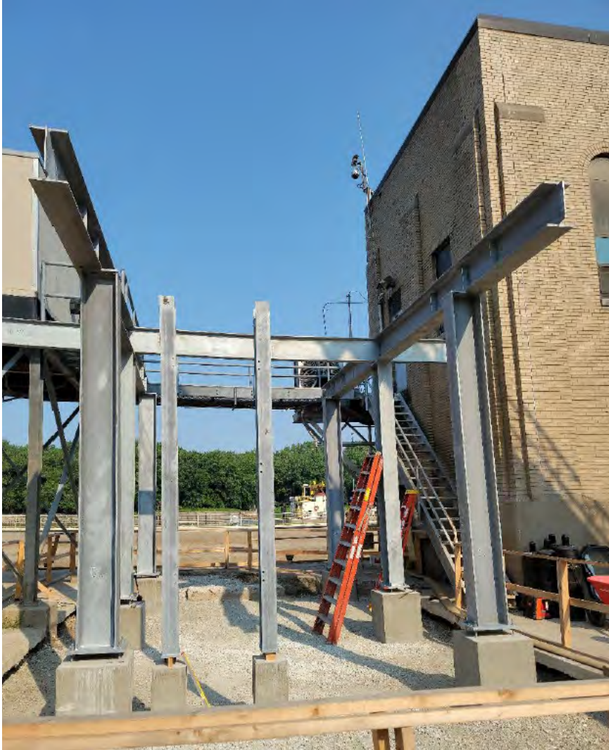
Elevated compressor platform
