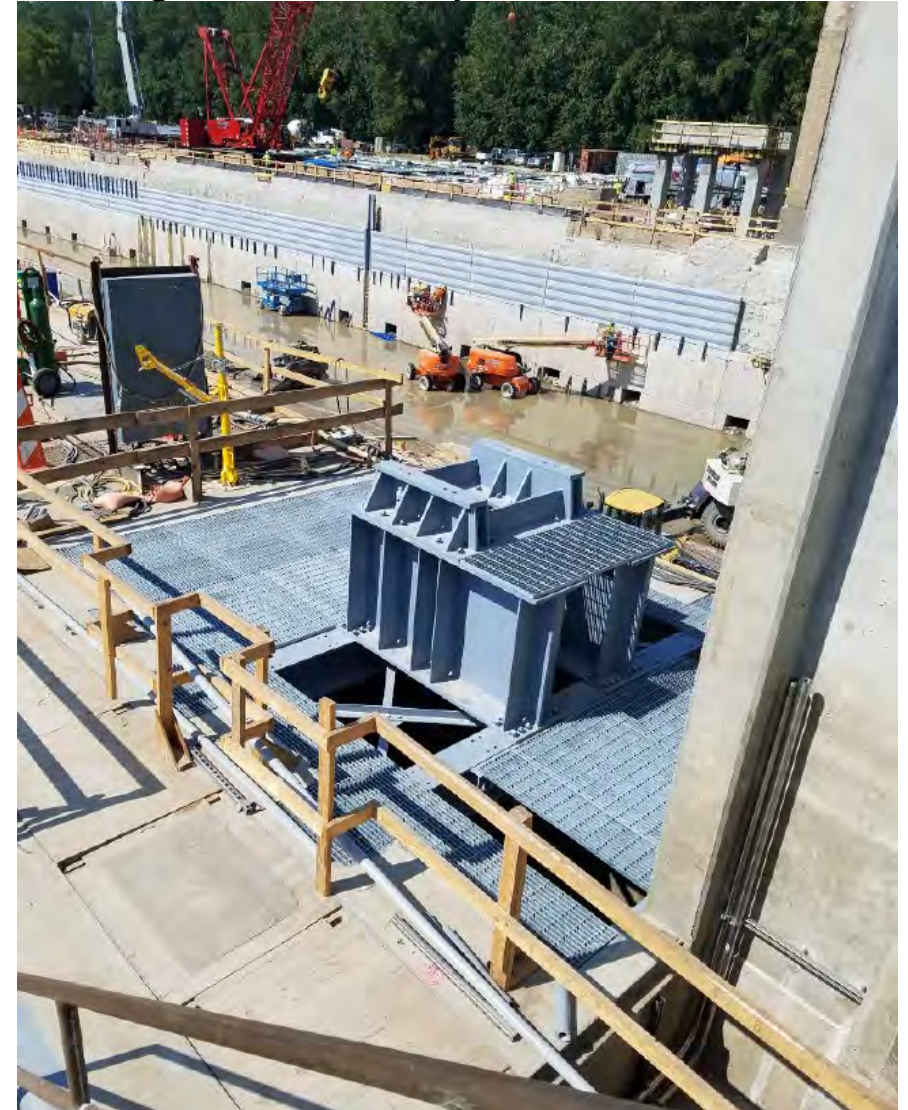
New gate machinery base
