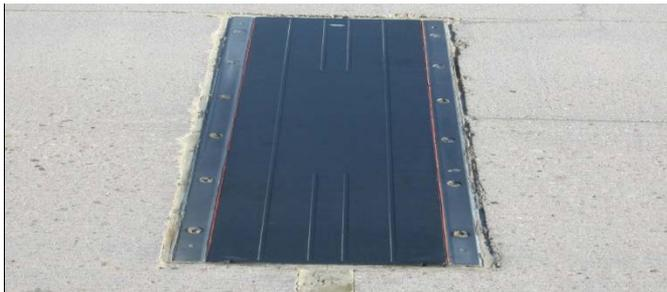
*Figure 7 – Bending Plate Installation*
