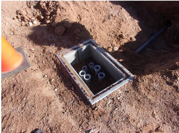
Figure 2 – Junction Box (lid cover removed)
