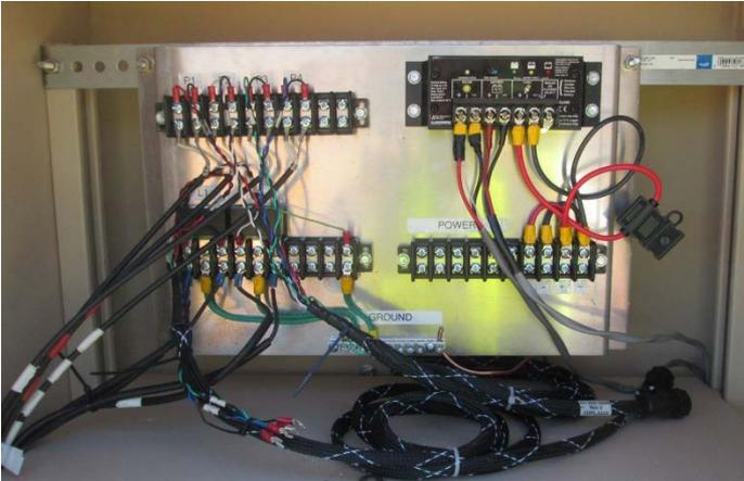
*Figure 48 – Terminal Panel Labels and Connections*
