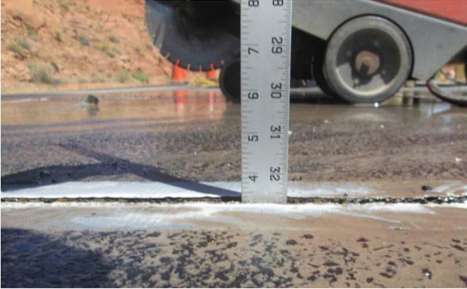
*Figure 44 – Sensor Slot Depth Check*
