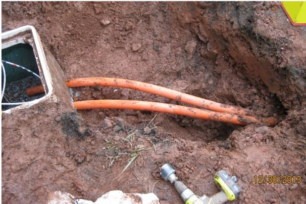
*Figure 18 – Bore Operation Conduit*
