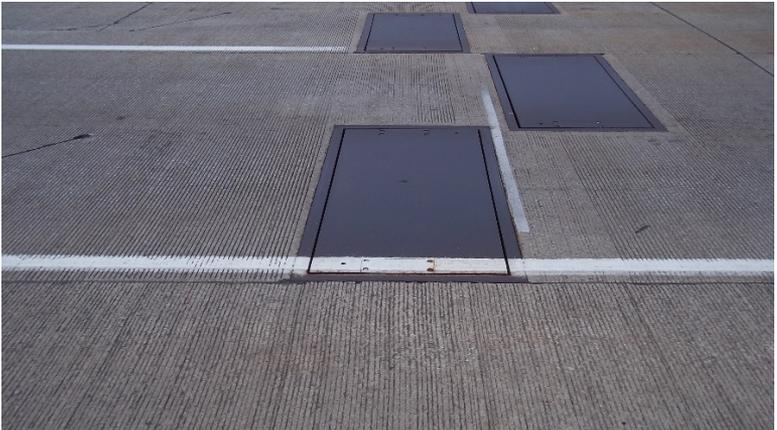
*Figure 9 – Load Cell Installation (Staggered Configuration)*
