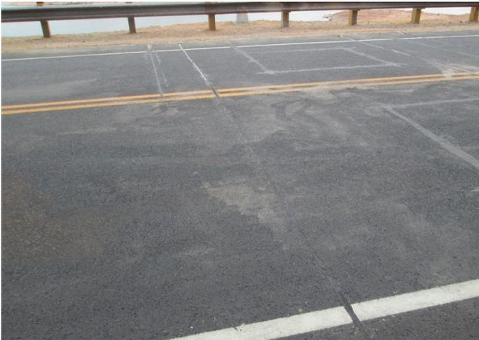
*Figure 46 – Completed Polymer Piezo Sensor Installation*
