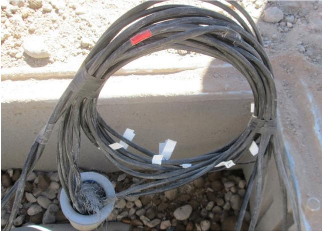
*Figure 47 – Sensor Lead Labeling and Service Loops in Pull Box*
