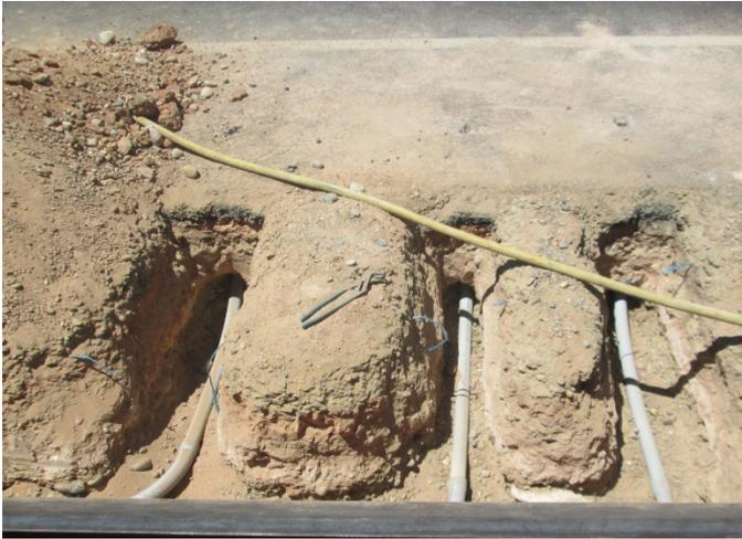
*Figure 33 – Sensor Conduits from Exit Hole to Pull Box*
