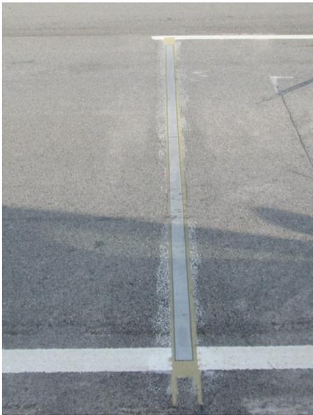
*Figure 42 – Completed Quartz Piezo Installation*
