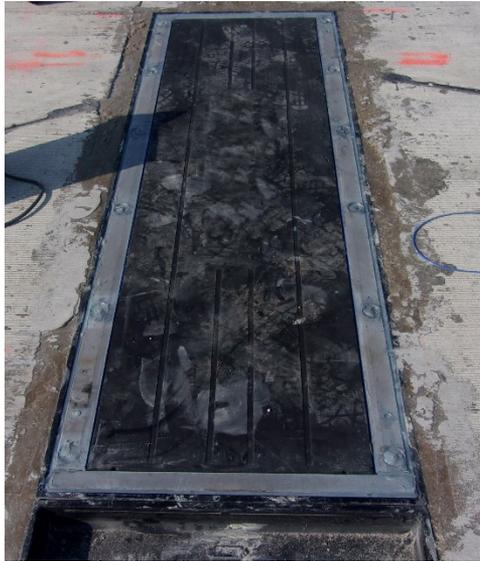
*Figure 41 – Completed Bending Plate Installation*
