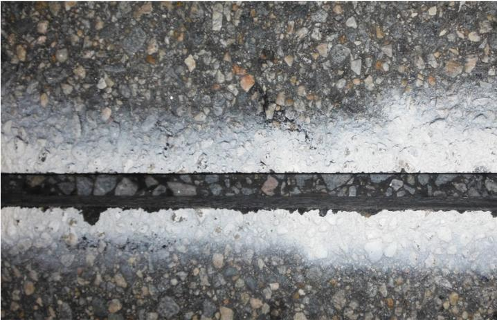
*Figure 45 – Piezo Slot Clean and Dry Check*
