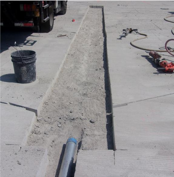
*Figure 40 – Excavated Bending Plate Pit (In-Line Configuration)*
