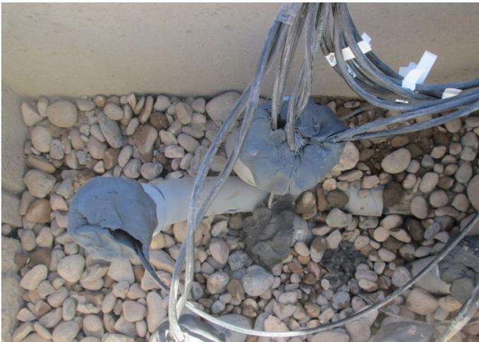
*Figure 34 – Pull Box Conduit Sealed with Duct Seal*
