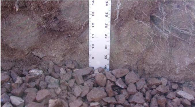
*Figure 36 – Drainage Gravel Depth Check*
