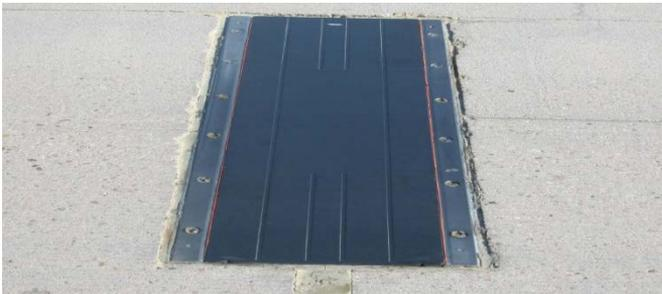
*Figure 5 – Bending Plate Installation*
