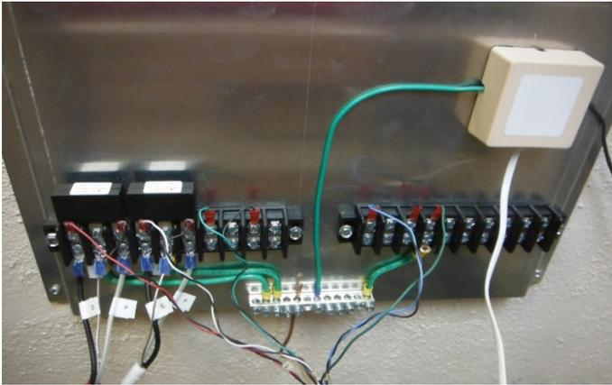
*Figure 29 – Sensor and Telephone Surge Arrester Devices*
