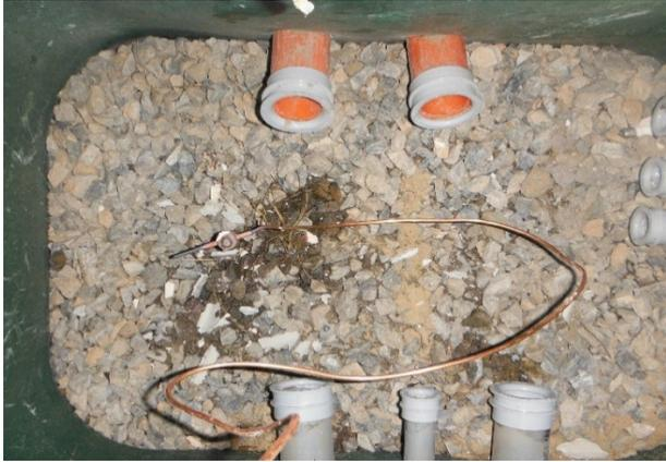
*Figure 30 – Grounding Rod with Cadweld™*
