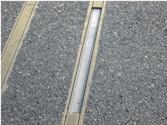
*Figure 19 – WIM Sensor Observed During Inspection*
