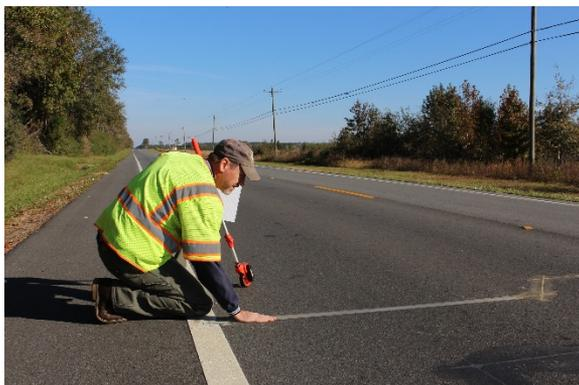
*Figure 9 – WIM Sensor Inspection*
