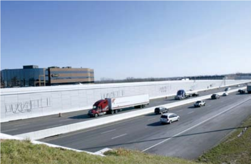
A wall along I-75 incorporates scale images of the Wright Brothers' historic flight. The length and elevation of the flight match the original 1903 milestone.
