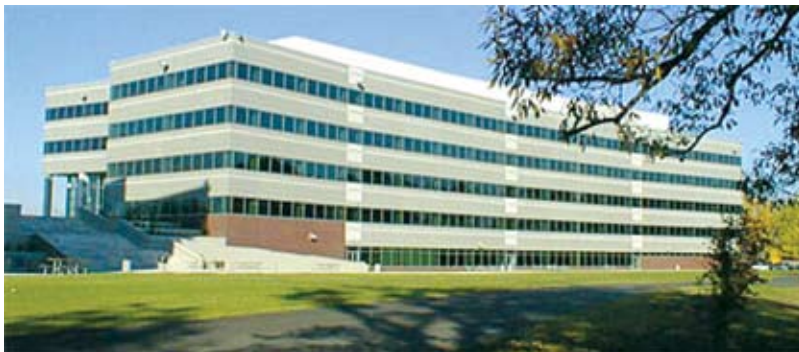
Central Office Hilltop Complex, Columbus, Ohio.
