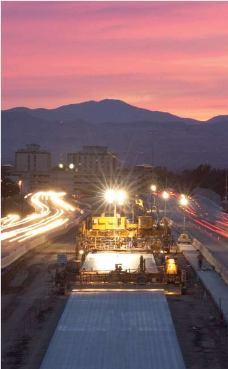
Concrete paving on I-25 at University Boulevard in Denver.
