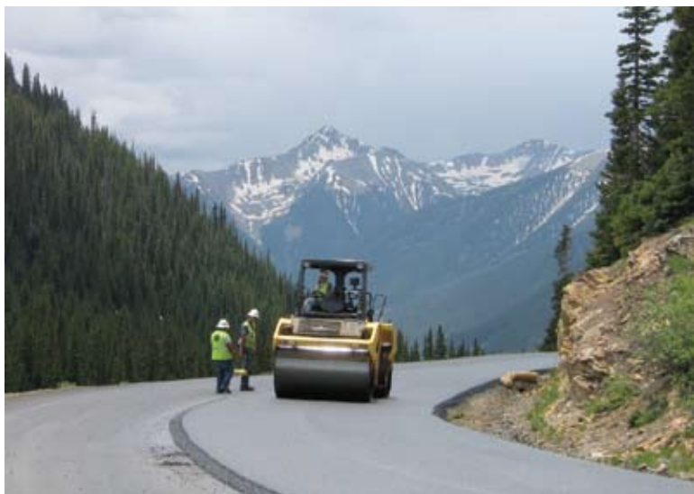
Photo courtesy of Denis Donnelly, Colorado Asphalt Paving Association
