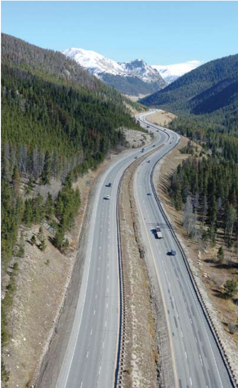
Aerial photo of I-70 near Shrine Pass.
