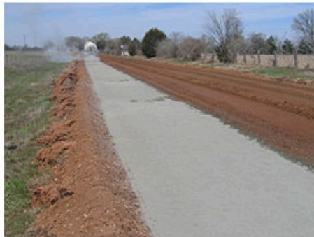
Figure 26. Full-Depth Reclamation (FDR): Recycle Old Roads into Smooth Roadways
