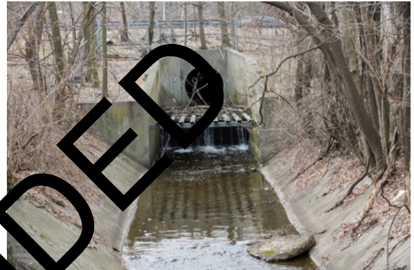
Figure 10-10: Accumulated debris on culvert rack (I-80 Milepost 57.3 Structure #1610177). (NJDOT)
