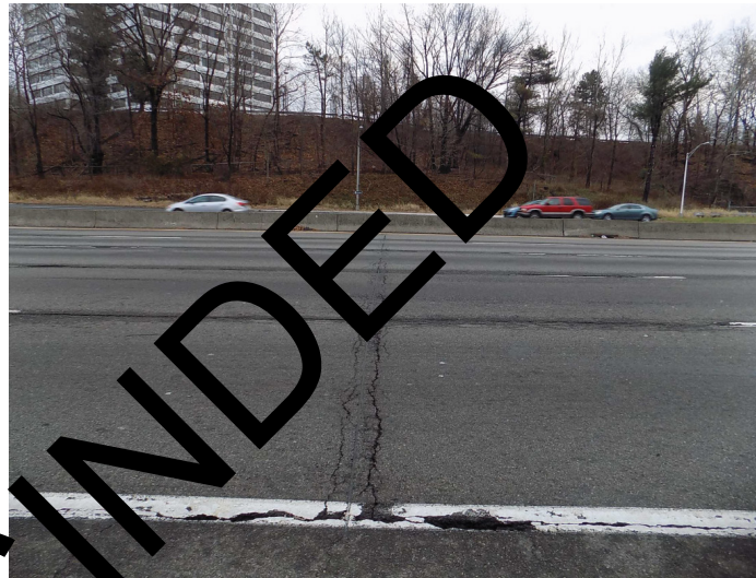
Figure 8-3. Example of pavement deterioration (NJDOT, 2019).
