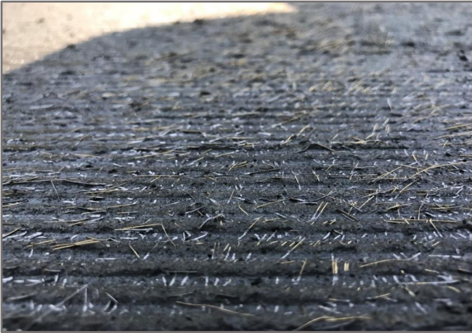
Figure 8 – Exposed steel fibers in UHPC deck overlay after grinding © 2018 DelDOT
