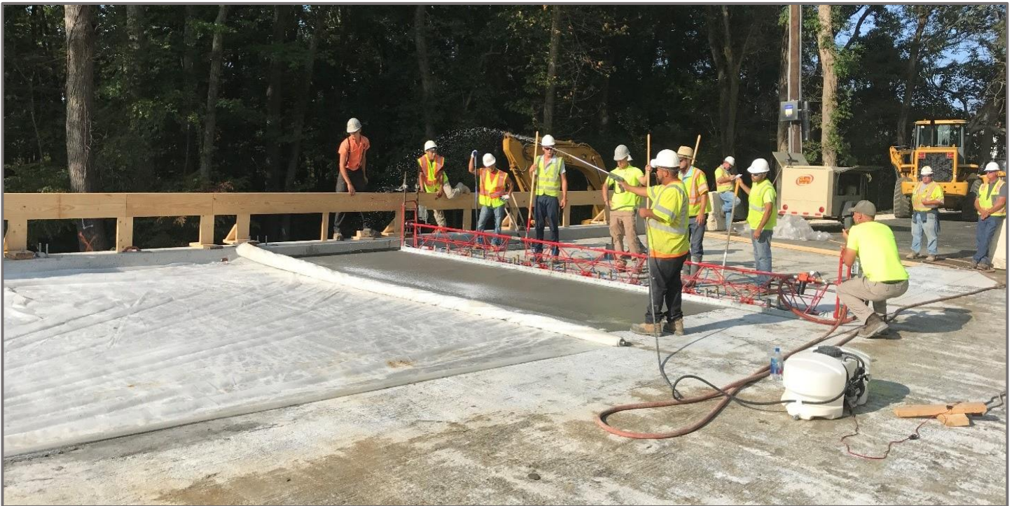
Figure 7 - UHPC deck overlay placement © 2018 DelDOT
