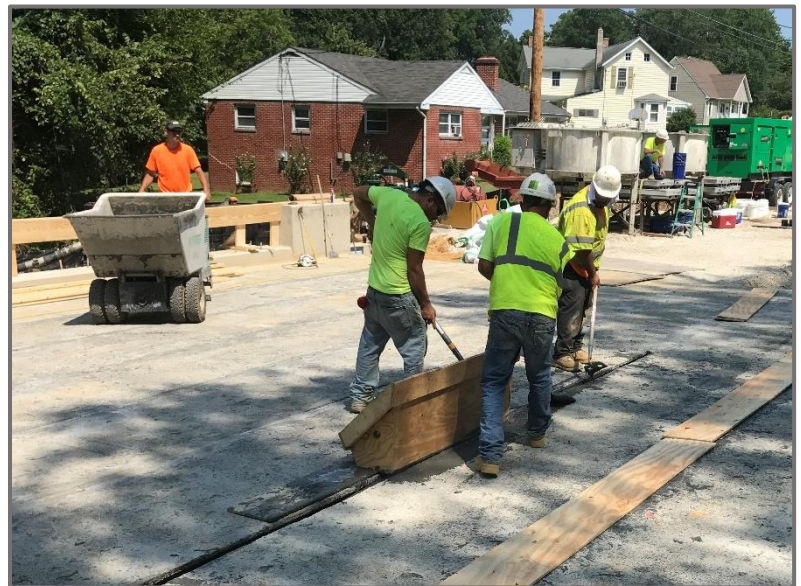
Figure 6 - Placement of UHPC in longitudinal box beam connections © 2018 DelDOT
