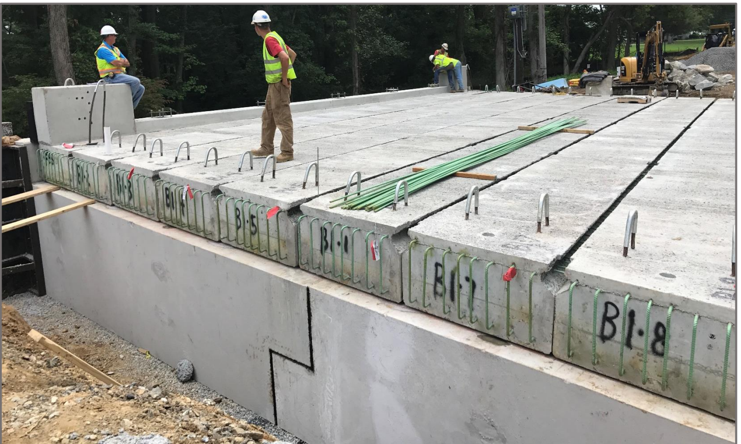
Figure 5 – The bridge after setting box beams in place, showing precast abutment wall joint, unfilled box beam longitudinal UHPC shear keys, and box beam rebar to connect to UHPC end diaphragm © 2018 DelDOT
