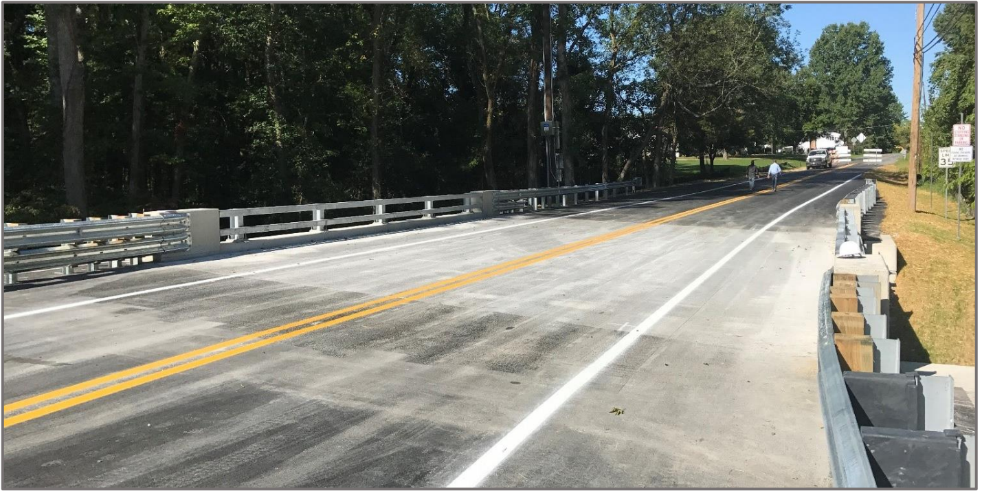
Figure 9 - UHPC deck overlay final riding surface © 2018 DelDOT
