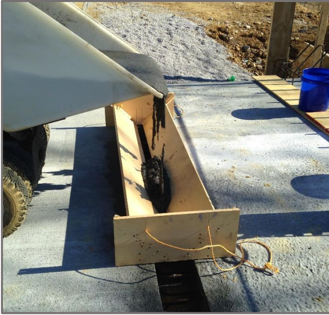
Figure 8 - Placement of UHPC in NEXT D beam connections using troughs © 2018 SCDOT
