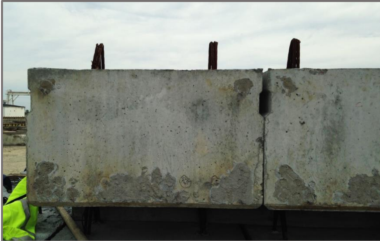
Figure 4 - Interior hollow-core beams with minimum 0.75-inch shear key joint openings © 2018 SCDOT
