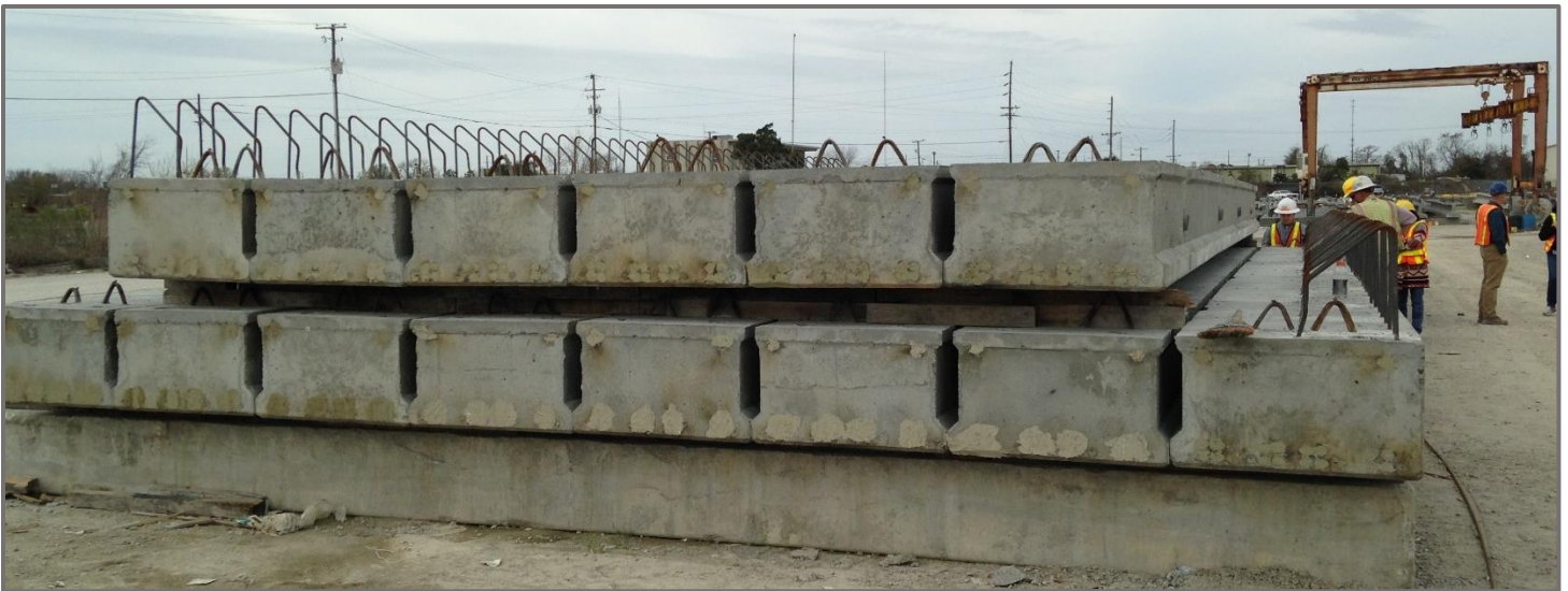
Figure 7 - Solid-slab beams with shear keys staged prior to construction © 2018 SCDOT
