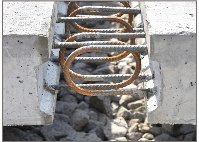
Figure 10 – NEXT D beam connection, note lack of surface roughening inside the connection © 2018 SCDOT
