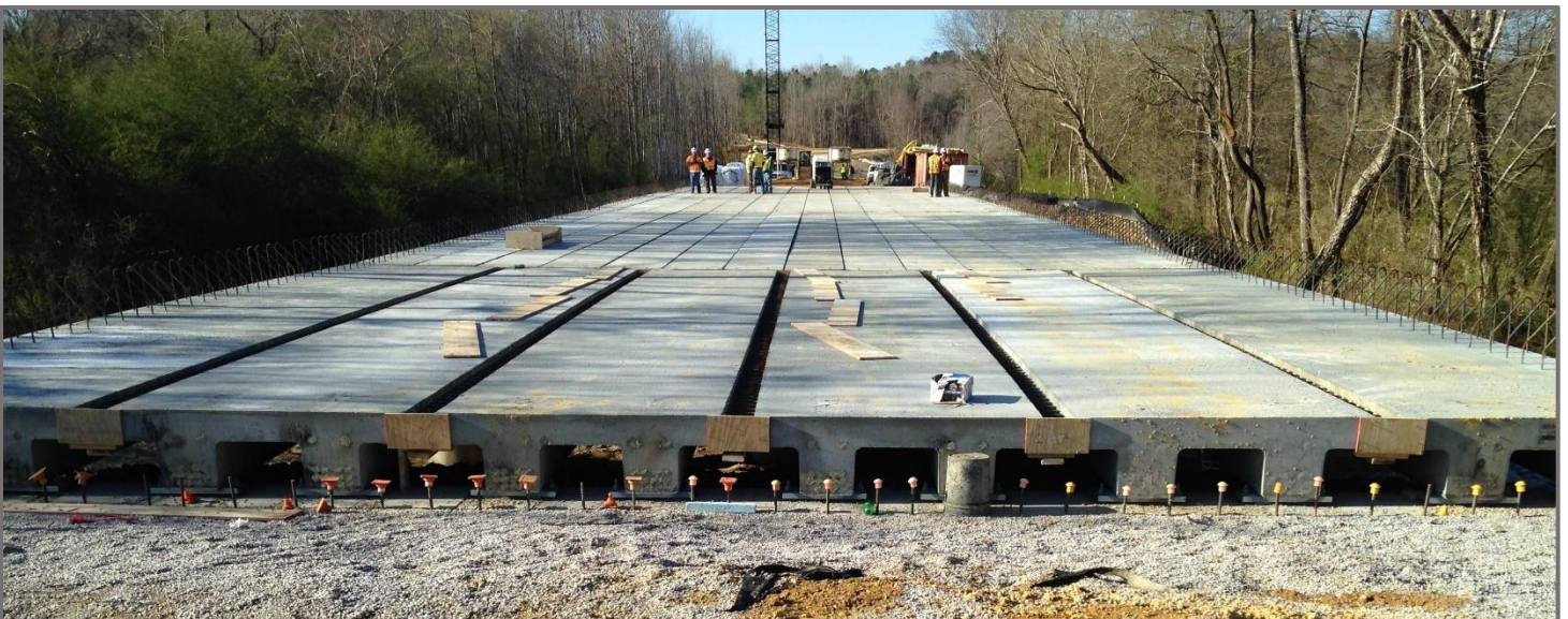
Figure 1 - Hanging Rock Creek Bridge during construction, with NEXT D beams in the foreground span © 2018 SCDOT
