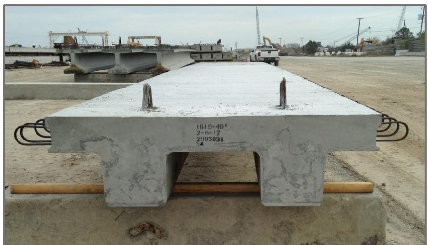
Figure 2 - Interior modified NEXT D beam © 2018 SCDOT
