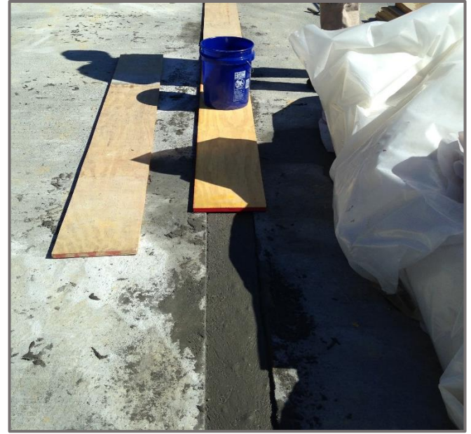
Figure 9 - Placement of UHPC, using chimney system and top formwork to control head pressure © 2018 SCDOT
