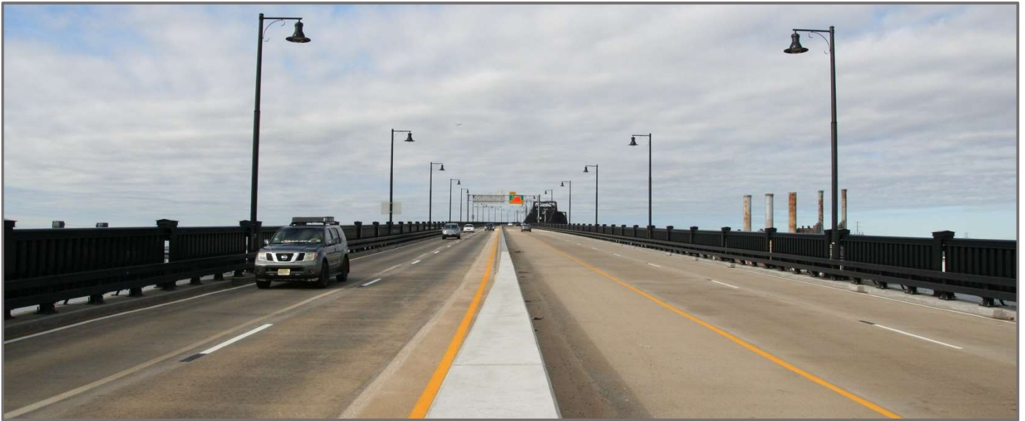
Figure 9 - Completed deck replacement © 2018 WSP USA
