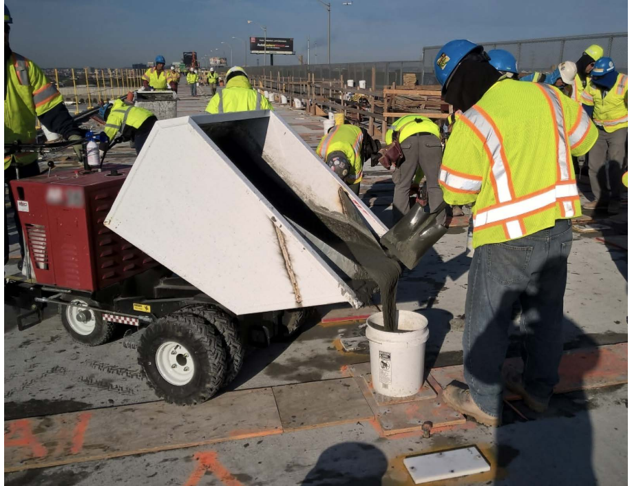
Figure 8 - Placing UHPC using motorized buggy © 2018 WSP USA
