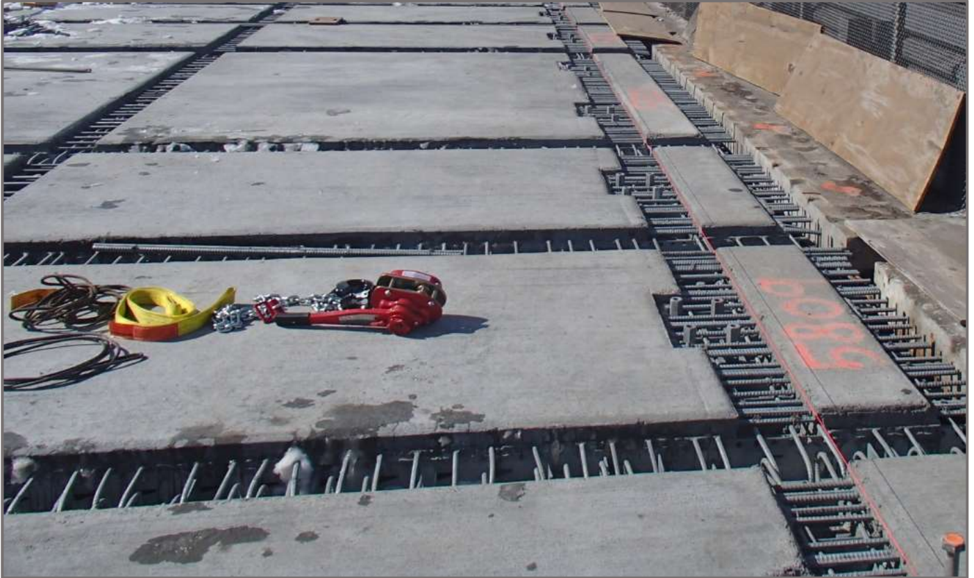
Figure 5 - Precast composite steel grid deck panels prior to UHPC placement, showing limited space between northbound deck panels and existing southbound deck on the right side of photograph © 2018 WSP USA
