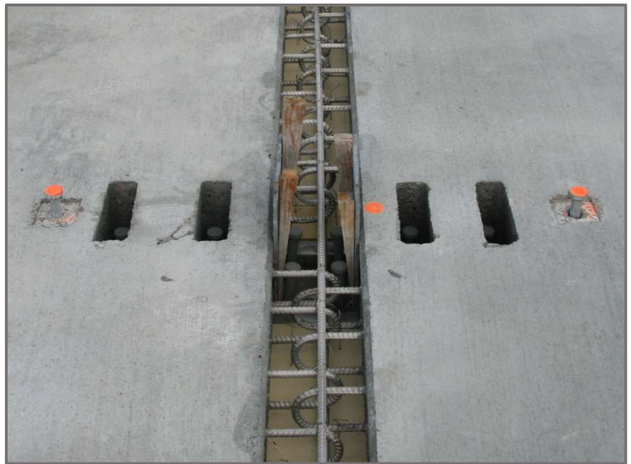
Figure 4 - Transverse connection between precast full-depth concrete deck panels prior to UHPC placement © 2018 WSP USA
