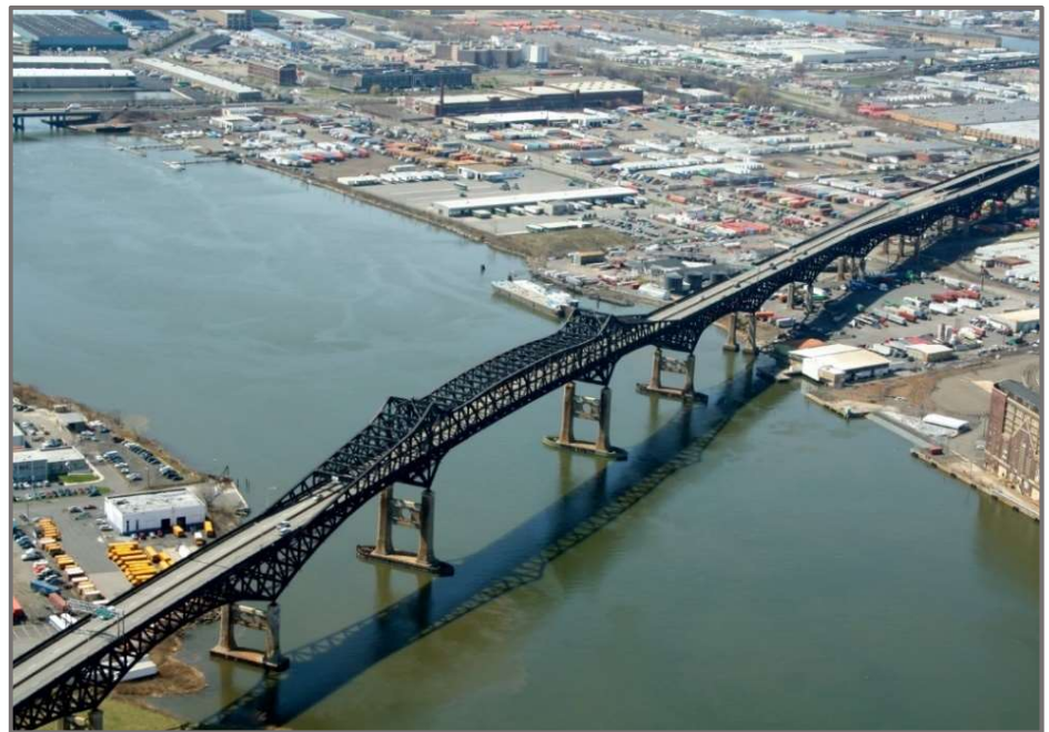
Figure 1 - Partial aerial view of the Pulaski Skyway © 2018 WSP USA
