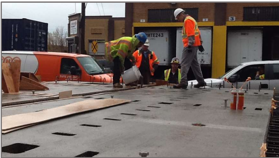
Figure 7 - Pouring of UHPC into demonstration deck panel joint © 2018 WSP USA
