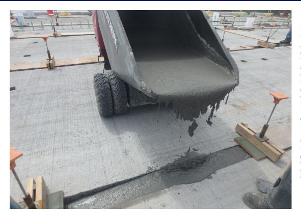
The UHPC connections were placed during July 2016. The UHPC mix was combined with chilled water, a superplasticizer liquid, and steel fibers onsite using two horizontal shaft mixers. The contractor added ice to the water to keep the mix temperature below 80°F. The contractor also used soaker hoses in the formwork overnight, and a hand-held sprayer just prior to the pour, to ensure that the connection interfaces had a saturated surface dry (SSD) condition.
