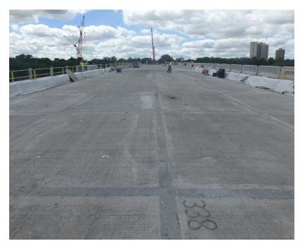
Fully cured connections were ground flush with surrounding deck panels through the use of typical construction equipment.
