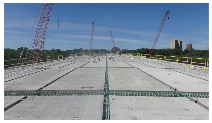
Deck panel placement was completed within tight tolerances on a 2 percent transverse grade. The deck reinforcement was typical to conventional deck design, but included short, straight rebar lap splices in the connections. Using UHPC allowed for shorter lap lengths between panel reinforcement, with the largest connection being 9 inches wide.
