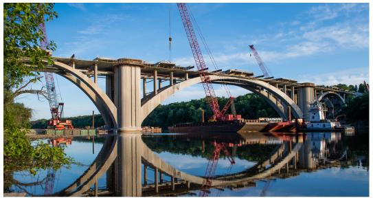
The Franklin Avenue Bridge is a historic crossing in downtown Minneapolis, MN, heavily used by drivers, pedestrians, and cyclists. Hennepin County used UHPC connections between precast deck panels to help accelerate the bridge's rehabilitation in 2016.
