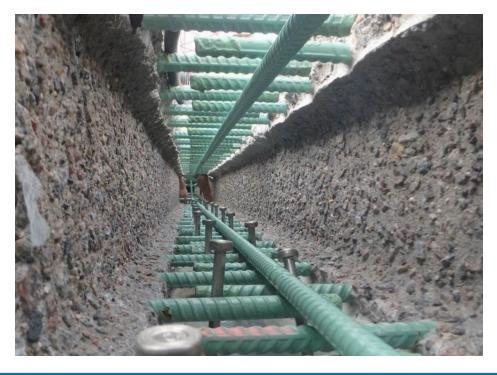
Joining the panels with UHPC achieved a full-moment connection by bonding to the exposed aggregate deck panel key-ways and splicing the reinforcing bars. The contractor understood that attaining an exposed aggregate finish with a minimum 1/4" amplitude was necessary to facilitate interface bond and avoid the potential for leakage.
