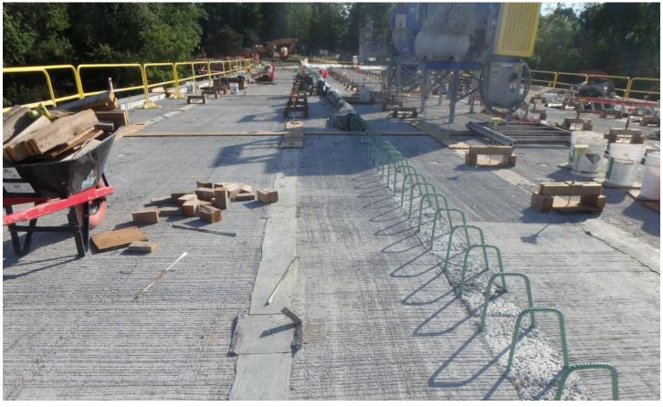
Forming accommodated removal of the top form to check that an SSD condition was met. Five-gallon buckets with a hole in the bottom were used as "chimneys" at the high points of the connections. This allowed the UHPC to flow into the connections after the top form was placed to ensure they were completely filled.
