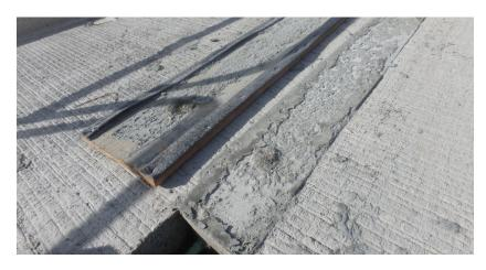
The UHPC connections were overfilled by 1/4", which allowed for removing air pockets and any other anomalies through surface grinding. A total of 350 cubic yards of field-cast UHPC was used to connect the precast panels.
