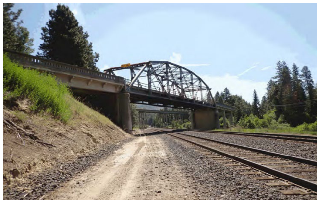
Photo Source: Local Highway Technical Assistance Council, Idaho
