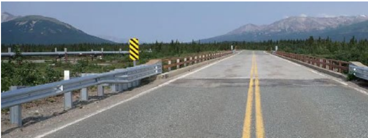
Source all photos: Alaska DOT&PF
