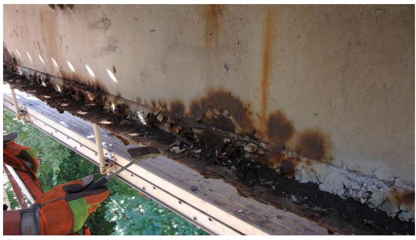
Closed captioned video with narration available: Inspector removing debris and laminar rust from a floorbeam
