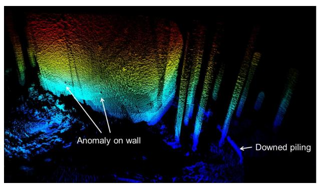
Figure 59. Image. 3D view of base of pier 3.
