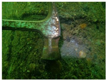
Figure 50. Photo. Typical cold joint after cleaning.
