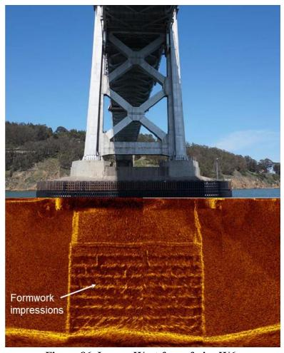
Figure 86. Image. West face of pier W6.
