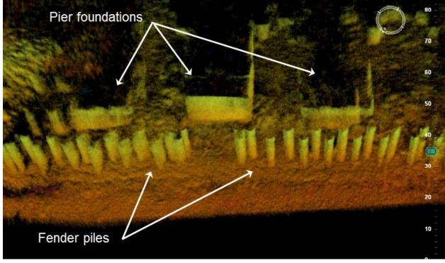
Figure 94. Image. Close-up of the south channel pier (Third Street Bridge).
