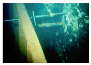
Figure 7-1 Commercial Rigid Form for Pier Repair Underwater
