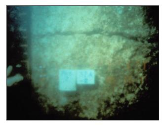
Figure 3-8 Cracked Concrete Member
