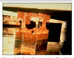
Figure 3-1 Steel Deterioration Resulting from Corrosion
