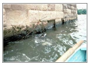
Figure 3-3 Deteriorated Masonry
