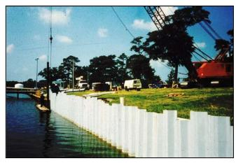
Figure 4-9 Polymer Sheet Pile Wall
