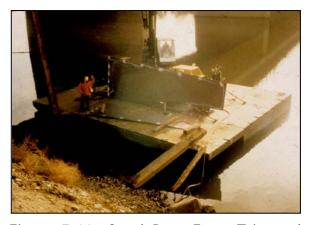
Figure 7-11 Steel Pate Form Trimmed to Fit Stream Bed
