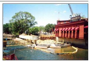
Figure 5-8 Bridge Pier with Dike Constructed of Soil, Traffic Barriers, and an Impervious Membrane
