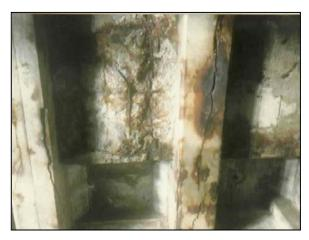
Figure 3-6 Cracks Along Reinforcing Bars
