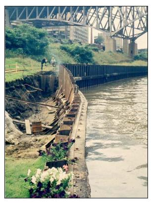
Figure 8-30 Sheet Pile Wall Failure
