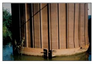
Figure 8-32 Reinforcing Band Placed on Sheet Pile Cell
