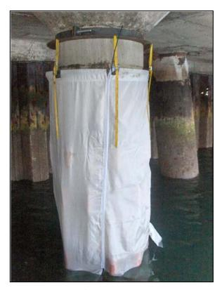
Figure 8-16 Fabric Form Installation
