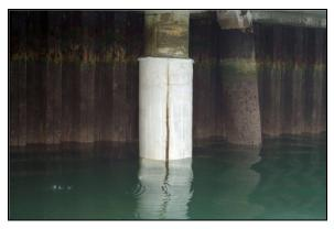
Figure 8-19 Completed Fabric Form Jacket
