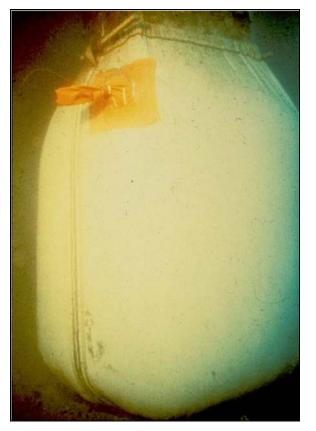
Figure 8-20 Completed Underwater Fabric Form Repair
