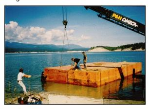
Figure 6-4 Sectional Barges Being Assembled
