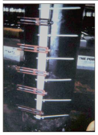
Figure 8-10 Pile Wrap Attachment
