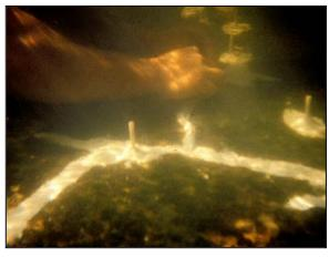
Figure 7-7 Injection of Resin through Port
