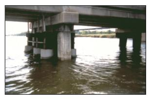
Figure 8-4 Supplemental Pile Bents (Crutch Bent)
