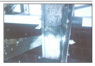
Figure 8-7 Pile Replacement Using Splice Plates
