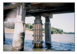
Figure 8-22 Completed Composite Jacket (Back Pile) and Jacket Read to by Pumped (Middle Pile). The Stiffening System is in Place on the Middle Pile Due to the Flexibility of the Fiberglass Jacket Form.
