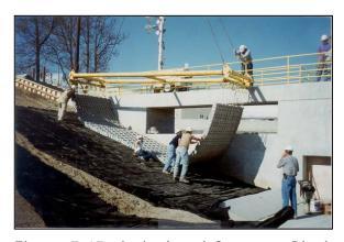
Figure 7-15 Articulated Concrete Block System Being Installed
