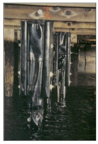
Figure 8-11 Wrap Installation at Pile Splice
