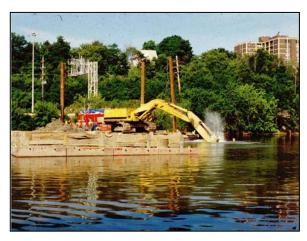
Figure 6-14 Hydraulic Excavator Performing Underwater Excavation
