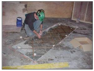
Figure 9-10 Galvanic Sacrificial Embedded Anodes Along Edge of Repair
