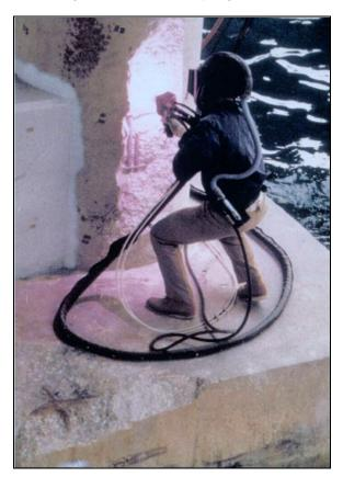
Figure 9-8 Application of Sprayed Zinc
