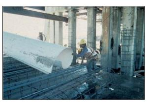
Figure 8-21 Semi-rigid Stay-in-Place Form; Note Also the Reinforcing Cages Sit Awaiting Forms
