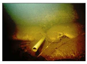
Figure 7-10 Grout Bag and Inlet Pipe
