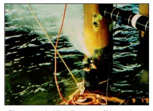
Figure 6-12 High Pressure Water Jet
