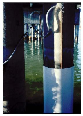
Figure 8-24 Epoxy Placement Pipes in Form
