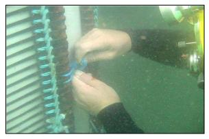
Figure 8-17 Stiffening System Being Secured in Place
