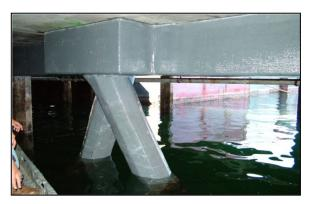
Figure 8-29 FRP Strengthening of Concrete Piles and Pile Cap
