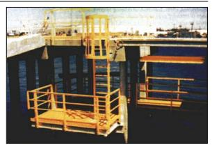
Figure 4-10 Platform Built of Fiber Reinforced Plastic Members and Decking
