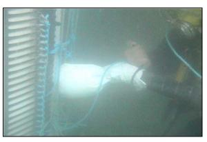
Figure 8-18 Pumping Grout into Form
