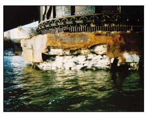
Figure 7-4 Bagged Concrete Emergency Repairs to Swing Pier
