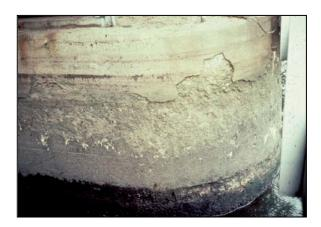
Figure 3-5 Deteriorated Concrete
