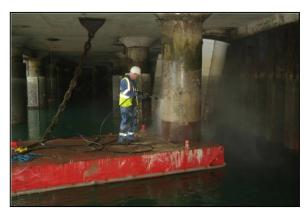
Figure 8-14 High Pressure Water Cleaning Prior to Pile Jacket Installation
