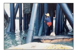
Figure 8-9 Pile Wrap Installation
