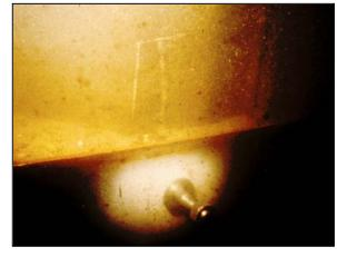
Figure 7-2 Permanent Steel Plate Form Secured with Expansion Anchor
