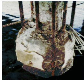
Figure 3-10 Concrete Pile During Repair
