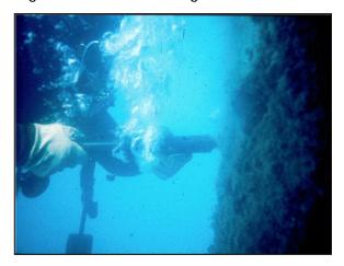
Figure 6-6 Pneumatic Needle Gun
