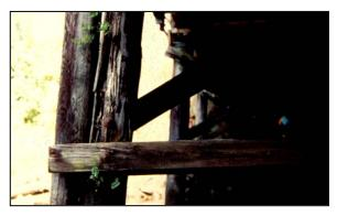
Figure 8-2 New Pile Driven Outside of Damaged Pile
