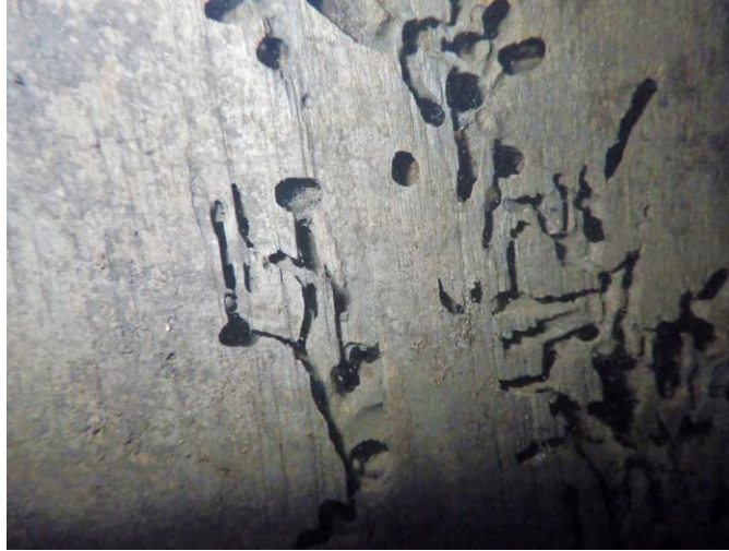
Figure 35. Photo. Marine borer damage in timber pile. (Source FHWA).
