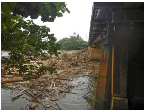
Figure 91. Photo. Heavy timber debris, Hawaii DOT, B.C.09 rating 3. (Source FHWA).
