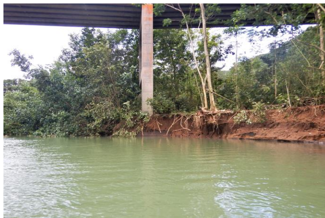
Figure 83. Photo. Channel migration threatening stability of bridge pier. (Source FHWA).
