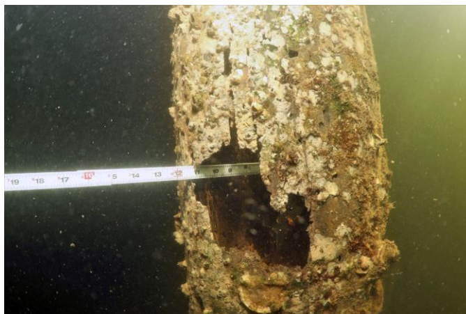
Figure 34. Photo. Timber pile with severe decay. (Source FHWA).
