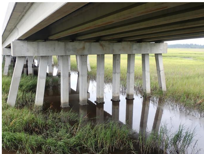
Figure 39. Photo. Example of concrete pile bent. (Source FHWA).
