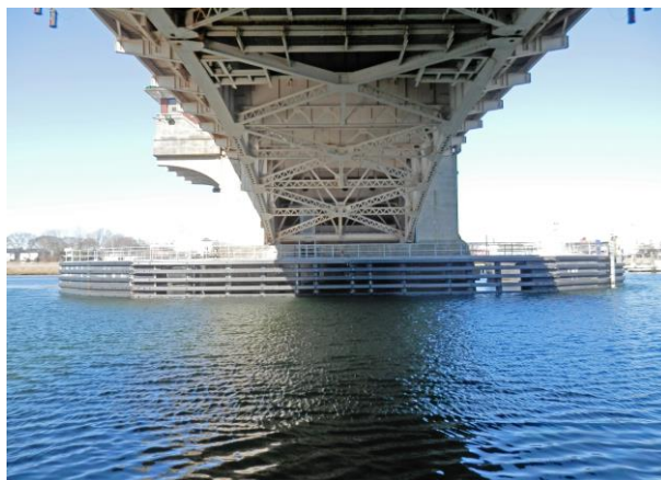
Figure 20. Photo. FRP bridge fender system. (Source FHWA).
