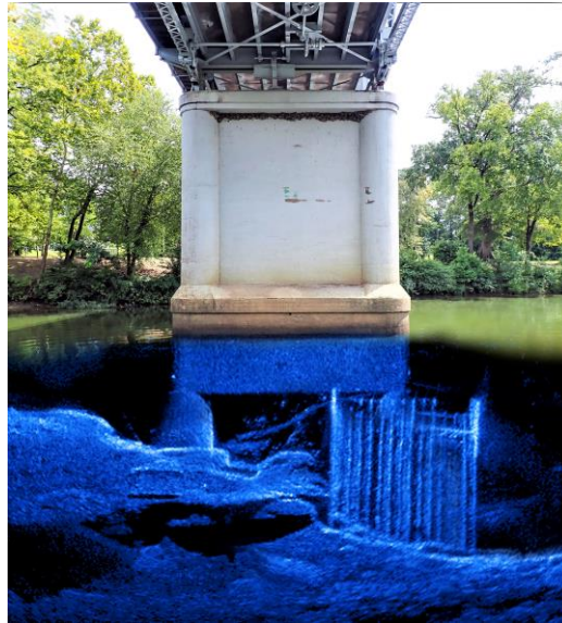
Figure 63. Graphic. Combined acoustic image of pier with debris lodged against footing. (Source FHWA).
