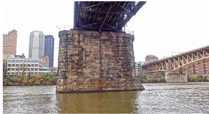
Figure 17. Photo. Example of a masonry bridge pier. (Source FHWA).
