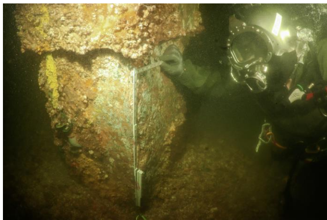
Figure 5. Photo. Level 2 inspection of a concrete pile at channel bottom. (Source FHWA).
