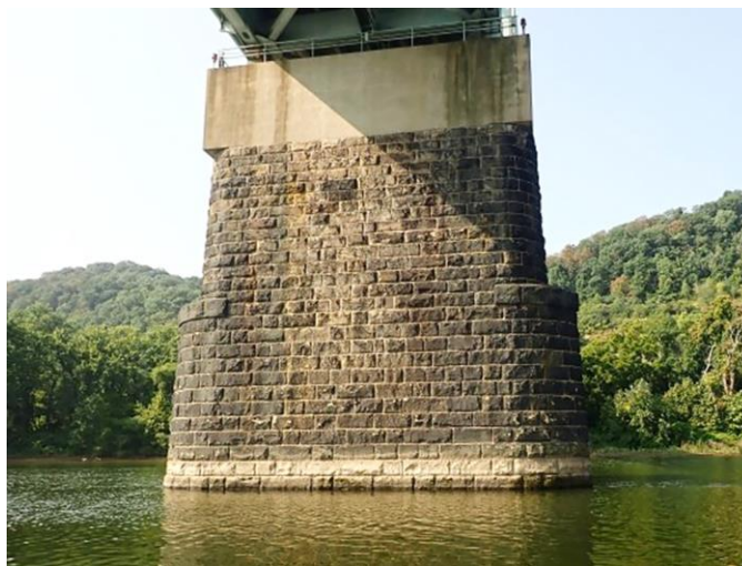
Figure 42. Photo. Example of a masonry pier. (Source FHWA).
