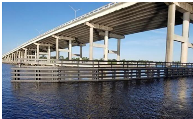
Figure 53. Photo. Example of a fender system. (Source FHWA).
