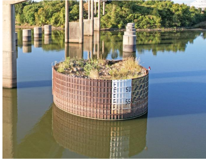
Figure 52. Photo. Example of a steel sheet pile dolphin cell. (Source FHWA).
