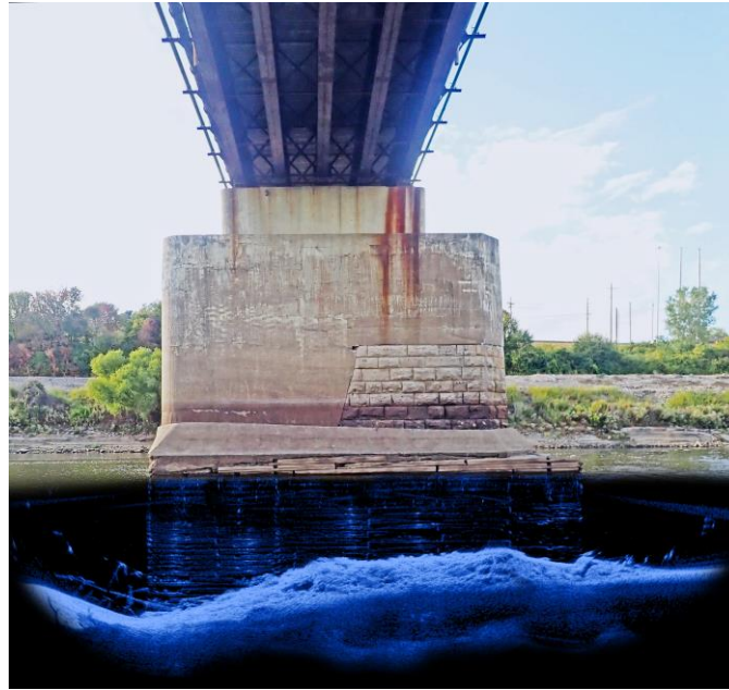
Figure 102. Graphic. 2D image of scour on a bridge pier. (Source FHWA).
