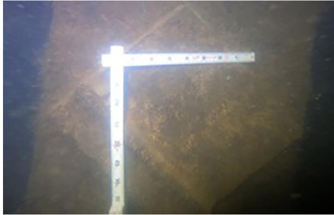
Figure 32. Photo. Example of steel pile splice. (Source FHWA).
