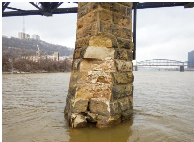
Figure 37. Photo. Vessel impact on bridge pier. (Source FHWA).
