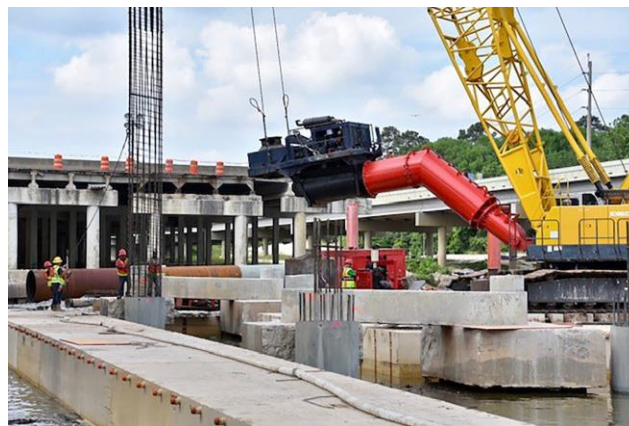
Figure 11. Photo. Construction of a cast-in-place bridge substructure. (Source FHWA).
