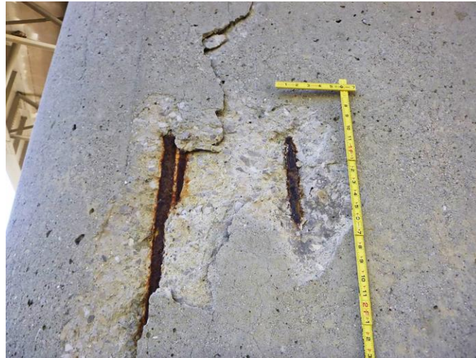
Figure 25. Photo. Surface spall with exposed and corroded reinforcing steel. (Source FHWA).
