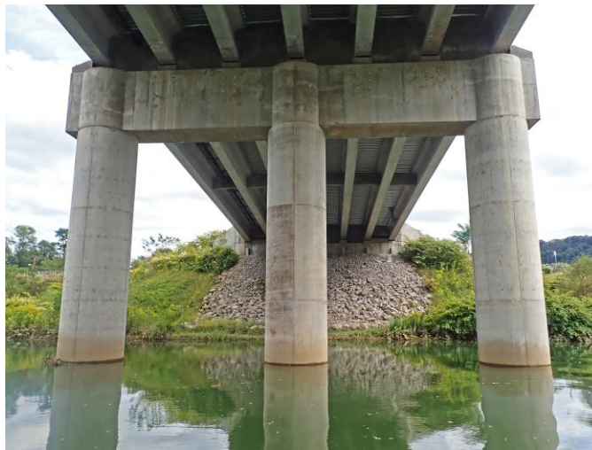
Figure 44. Photo. Example of a multi-column pier. (Source FHWA).
