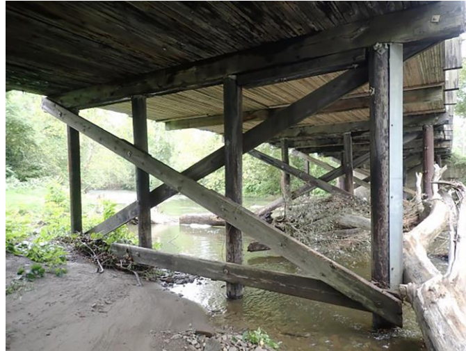
Figure 18. Photo. Example of timber pile bent, coded as T03. (Source FHWA).
