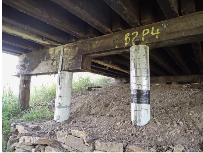
Figure 80. Photo. Timber pile bent with wrapped piles. (Source FHWA).
