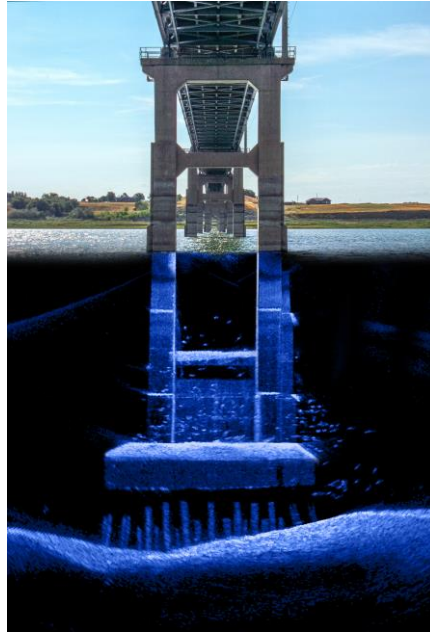
Figure 14. Graphic. Bridge pier supported by steel H-piles. (Source FHWA).
