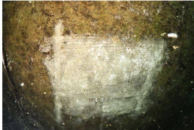
Figure 7. Photo. Example of 1-sq-ft level 2 cleaning on a reinforced concrete (RC) pier wall. (Source FHWA).
