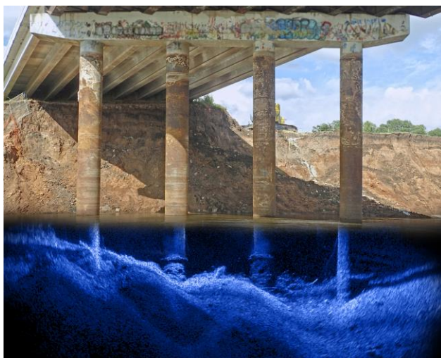
Figure 67. Graphic. Combined acoustic image of a drilled shaft bent configuration. (Source FHWA).
