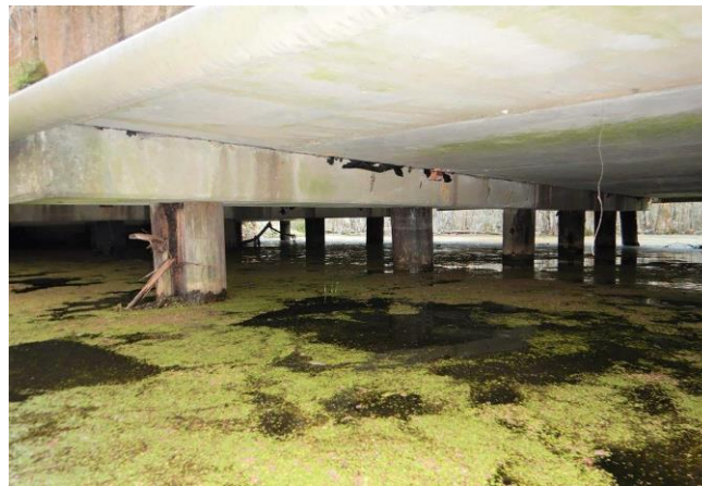
Figure 19. Photo. Timber pile bent with RC cap. (Source FHWA).
