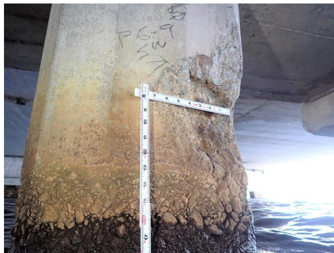
Figure 26. Photo. Spall in splash zone. (Source FHWA).
