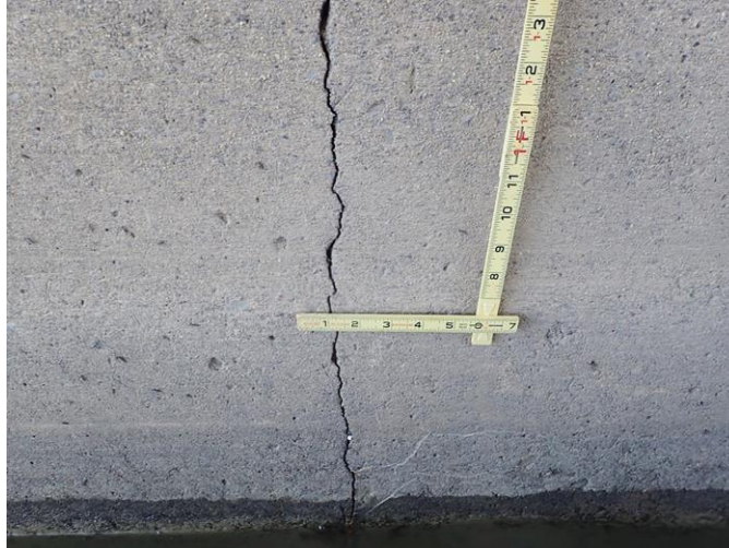
Figure 21. Photo. Shrinkage cracks on RC pier wall. (Source FHWA).
