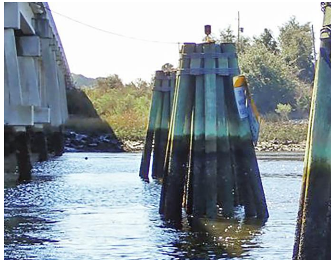
Figure 51. Photo. Example of a timber dolphin. (Source FHWA).
