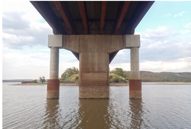
Figure 38. Photo. Widened substructure unit with two different substructure types. (Source FHWA).
