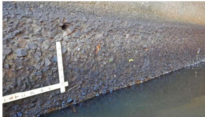
Figure 24. Photo. Scaling of concrete pier at waterline. (Source FHWA).
