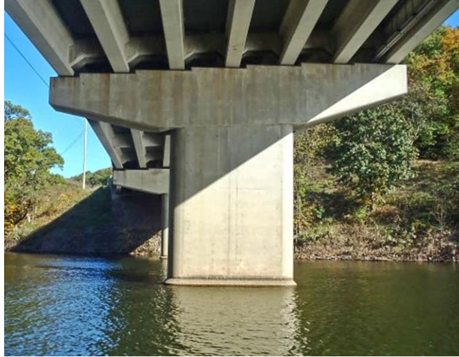
Figure 43. Photo. Example of a single-column hammerhead pier. (Source FHWA).
