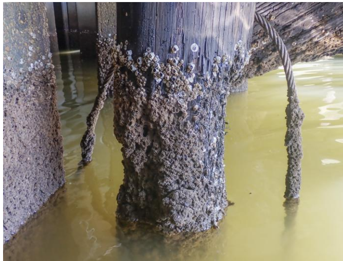
Figure 36. Photo. Example of hourglass shape as a result of marine borer damage. (Source FHWA).
