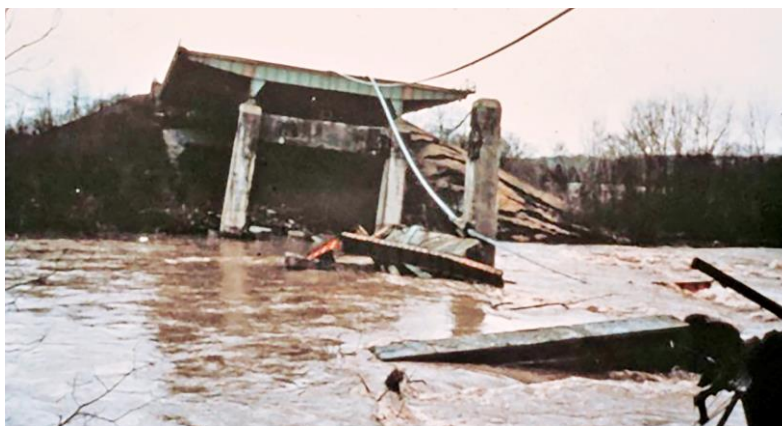
Figure 1. Photo. Schoharie Creek bridge failure (1987). (Source FHWA).
