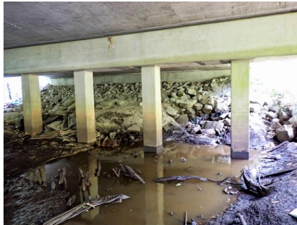
Figure 92. Photo. Displaced riprap with erosion, South Carolina DOT, B.C.10 rating 4. (Source FHWA).
