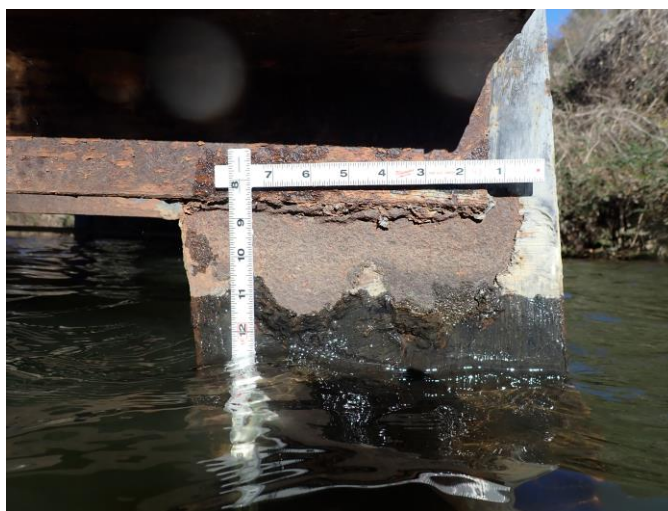
Figure 30. Photo. Galvanic corrosion of steel H-pile. (Source FHWA).
