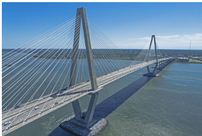
Figure 45. Photo. Cable-stayed bridge with tower pier substructure. (Source FHWA).
