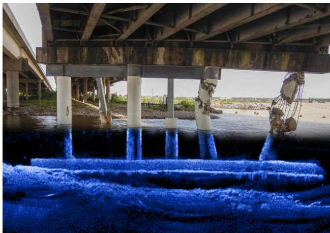
Figure 58. Graphic. Acoustic image of bridge after vessel impact. (Source FHWA).
