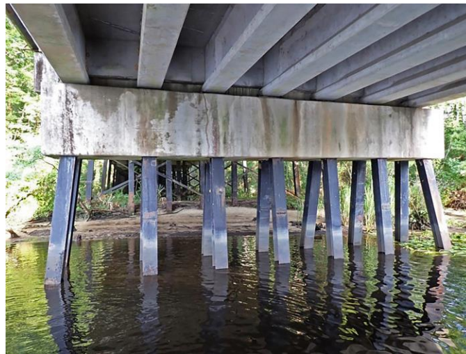
Figure 15. Photo. Example of a steel H-pile bent. (Source FHWA).
