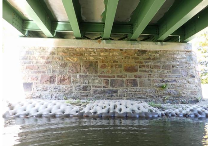
Figure 90. Photo. Mattress installed around bridge pier. (Source FHWA).
