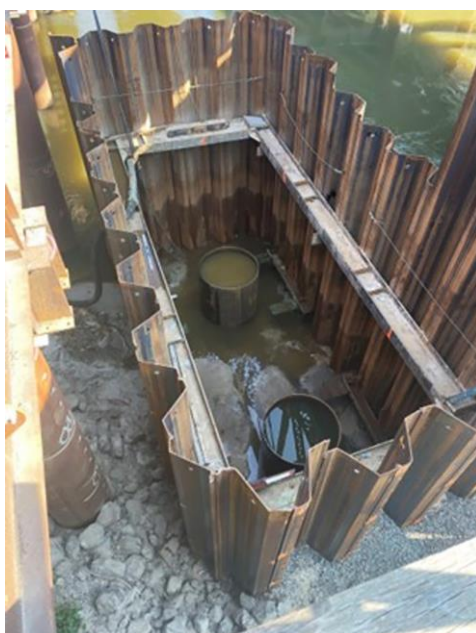
Figure 50. Photo. Cofferdam used to dewater for footing construction. (Source PCL Construction).
