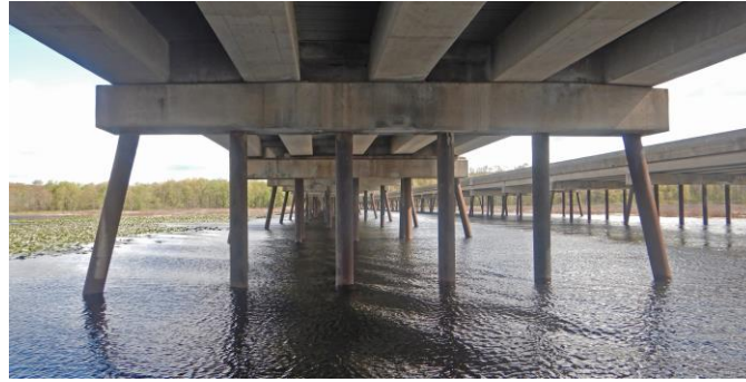
Figure 16. Photo. Example of steel pipe piles. (Source FHWA).
