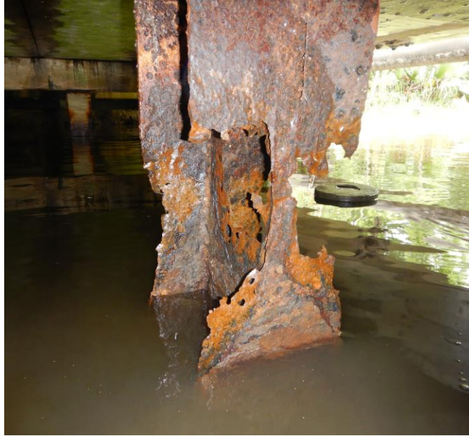
Figure 29. Photo. Example of corrosion on a steel pile. (Source FHWA).
