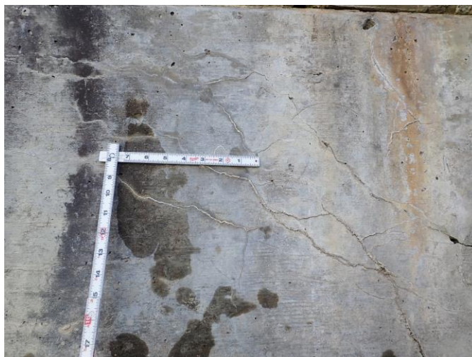
Figure 27. Photo. Example of ASR. (Source FHWA).
