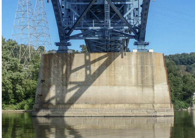
Figure 41. Photo. Example of a pier wall. (Source FHWA).
