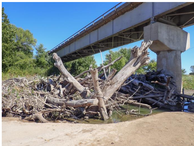
Figure 93. Photo. Timber debris lodged upstream of a bridge pier documented during channel above-water inspection. (Source FHWA).
