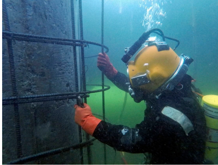
Figure 50. Photo. Reinforcing steel prepared for repair. (Source JF Brennan Company).
