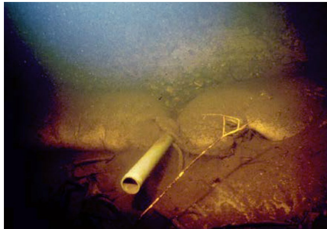
Figure 56. Photo. Grout bags used to repair undermining. (Source FHWA).
