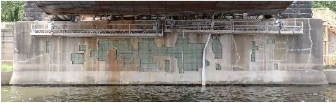
Figure 49. Photo. Concrete repair preparation. (Source FHWA).
