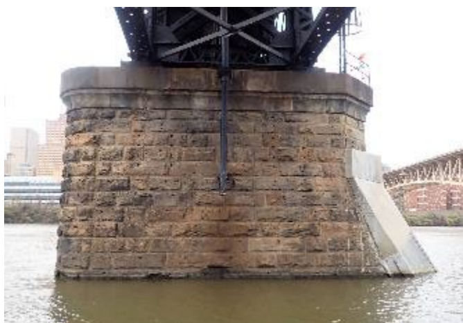
Figure 55. Photo. Concrete masonry repair. (Source FHWA).
