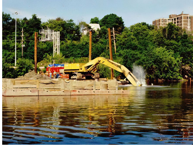
Figure 32. Photo. Excavator mounted on a barge. (Source FHWA).
