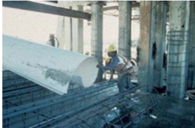
Figure 74. Photo. Concrete pile being strengthened with a structural jacket. (Source FHWA).
