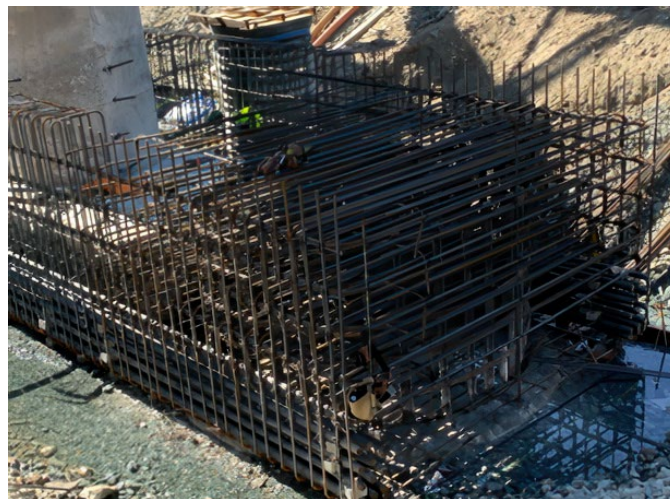
Figure 64. Photo. Reinforcing to extend footing and tie-in new drilled shafts. (Source FHWA).
