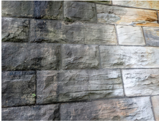
Figure 18. Photo. Mortar securing stones of a masonry substructure. (Source FHWA).
