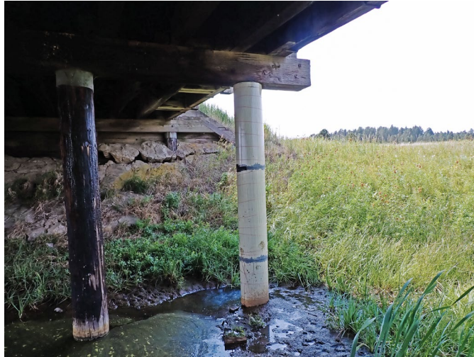
Figure 69. Photo. Timber pile wrap. (Source FHWA).
