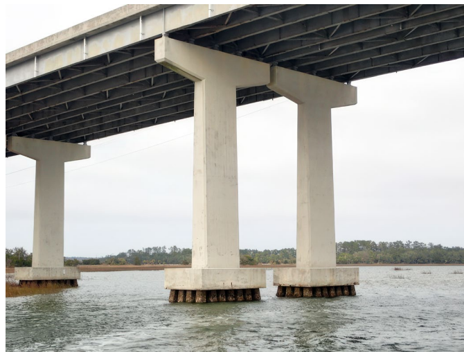
Figure 6. Photo. Pile-supported footings. (Source FHWA).
