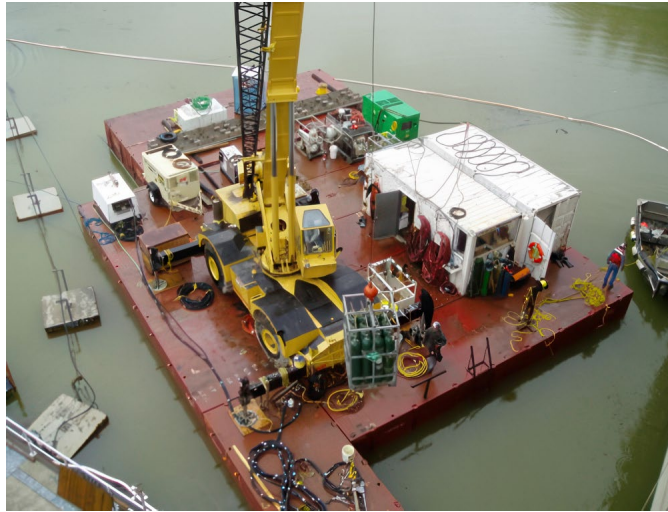
Figure 22. Photo. Marine construction site. (Source Global Diving and Salvage).
