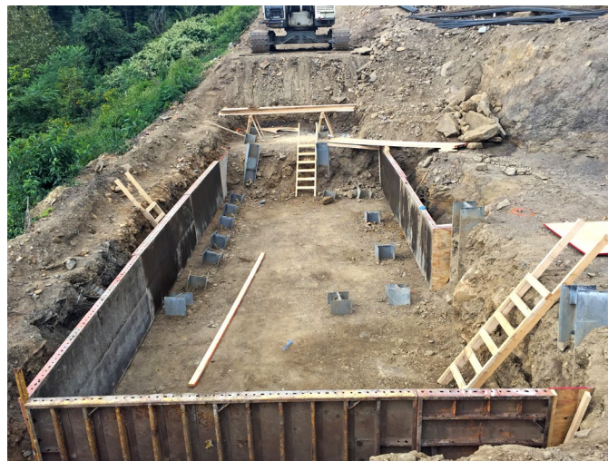
Figure 47. Photo. Rigid formwork. (Source FHWA).
