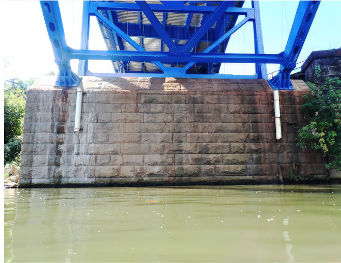
Figure 16. Photo. Stone masonry pier wall. (Source FHWA).
