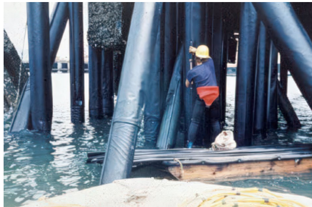
Figure 70. Photo. Steel pile wrap. (Source FHWA).
