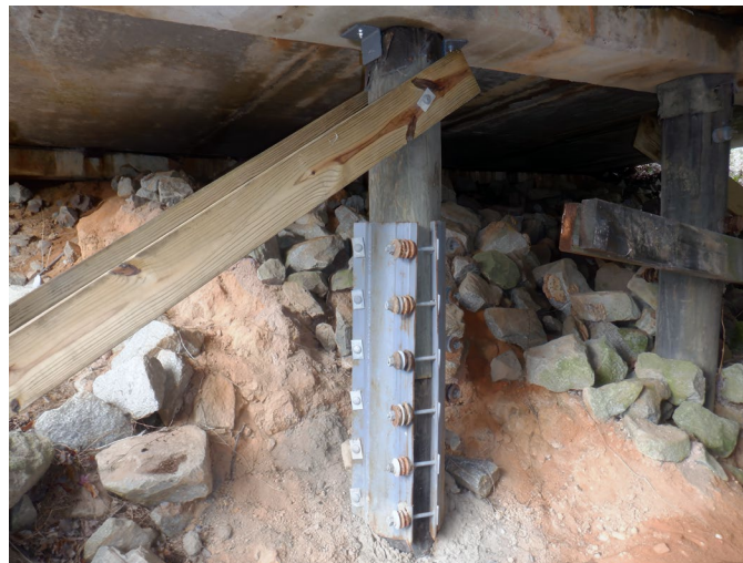
Figure 77. Photo. Fish plates used for partial pile replacement. (Source FHWA).
