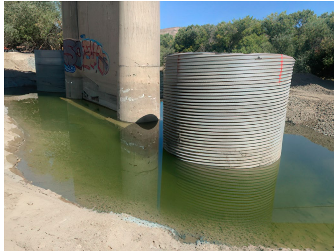
Figure 63. Photo. Drilled shafts were installed to strengthen the existing pier. (Source FHWA).
