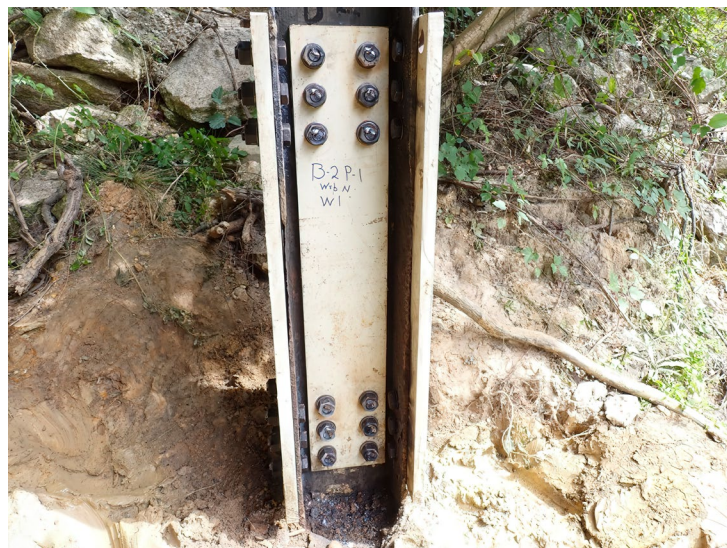
Figure 15. Photo. Field-coated steel plate installed as part of a pile repair. (Source FHWA).
