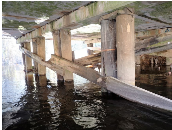
Figure 78. Photo. New timber piles driven adjacent to deteriorated piles. (Source FHWA).
