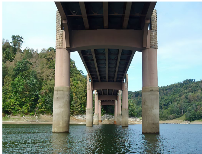
Figure 7. Photo. Drilled shaft bent. (Source FHWA).
