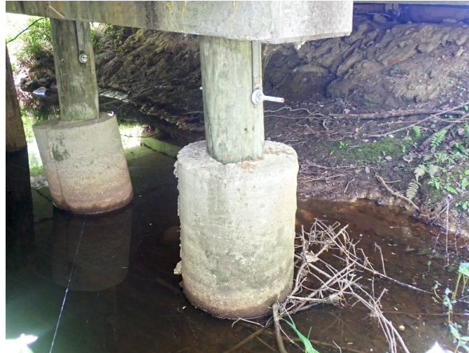
Figure 71. Photo. Concrete pile jacket. (Source FHWA).
