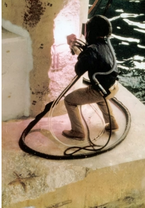
Figure 83. Photo. Sprayed zinc is applied to a bridge substructure. (Source FHWA).
