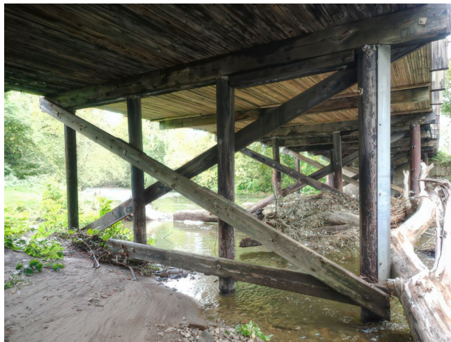
Figure 19. Photo. Timber pile bent. (Source FHWA).
