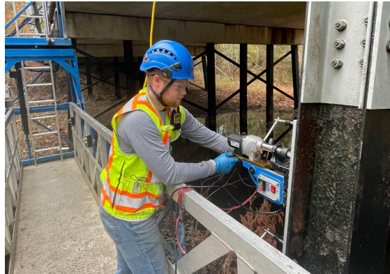
Figure 72. Photo. Electromagnetic drill press used to facilitate repair connections. (Source FHWA).
