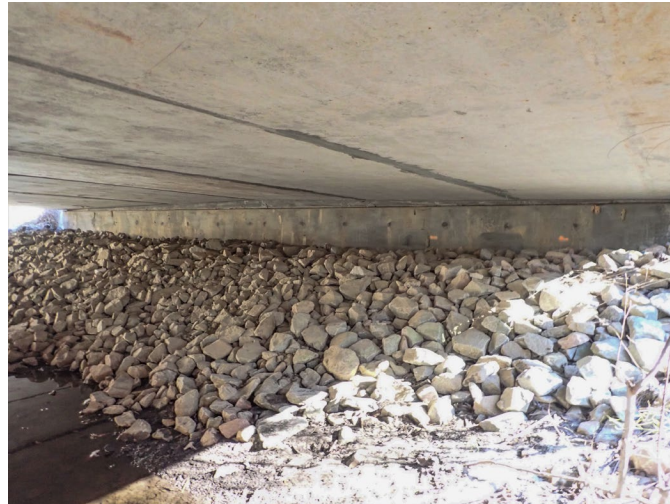
Figure 60. Photo. Riprap along bridge abutment.
