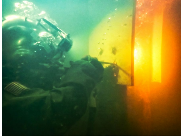
Figure 68. Photo. Diver strengthening a steel pile by attaching a steel plate to the flange. (Source FHWA).
