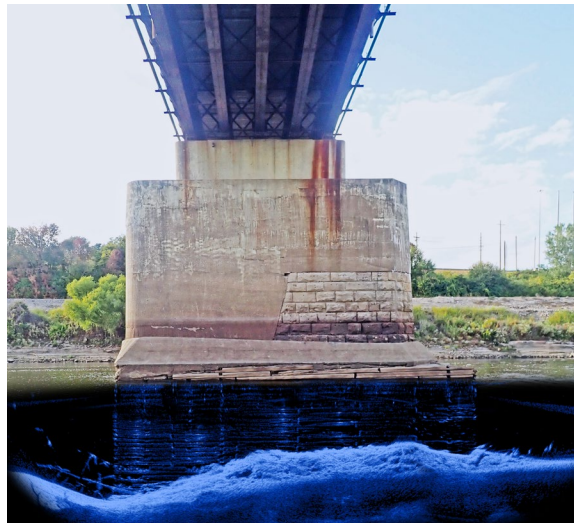
Figure 40. Graphic. Combined 2D acoustic image of a bridge pier. (Source FHWA).
