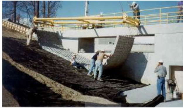
Figure 61. Photo. Articulating concrete block system used as scour countermeasure. (Source FHWA).
