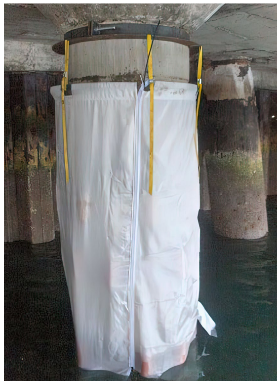
Figure 48. Photo. Flexible formwork installation. (Source FHWA).
