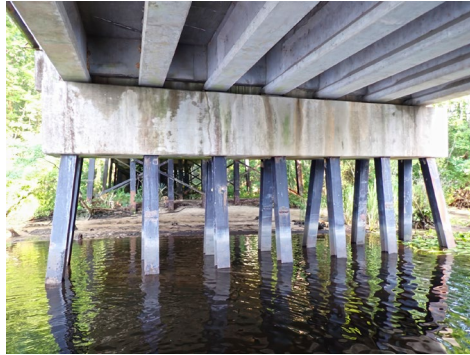
Figure 12. Photo. Steel H-pile bent. (Source FHWA).
