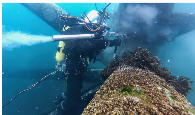
Figure 34. Photo. Diver operating a water blasting system. (Source Global Diving and Salvage).
