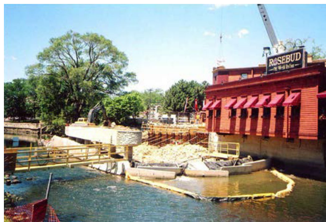
Figure 27. Photo. Dike around construction site. (Source FHWA).
