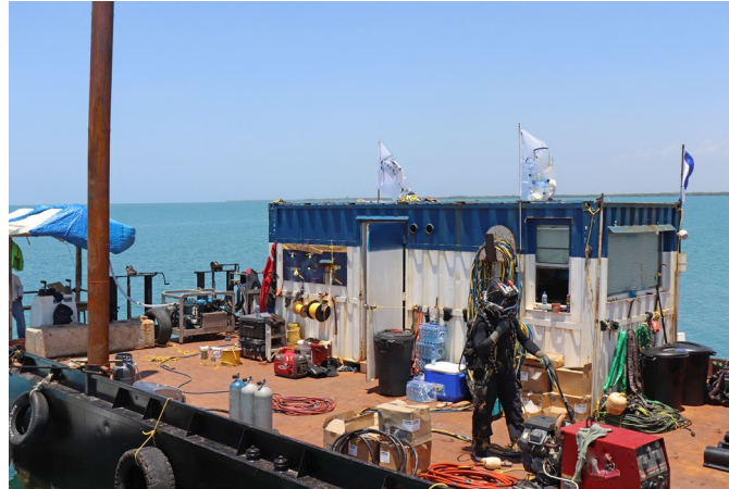
Figure 29. Photo. Dive team and support equipment on a construction site. (Source Global Diving and Salvage).
