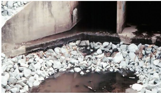
Figure 62. Photo. Riprap used to repair undermining at culvert. (Source FHWA).
