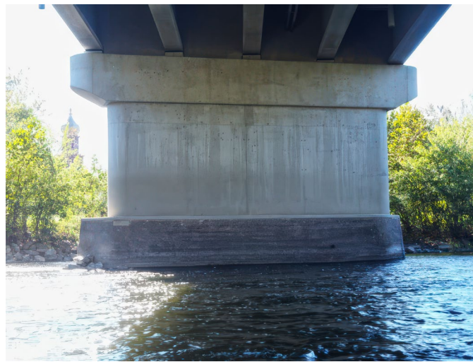
Figure 8. Photo. Reinforced concrete pier wall. (Source FHWA).
