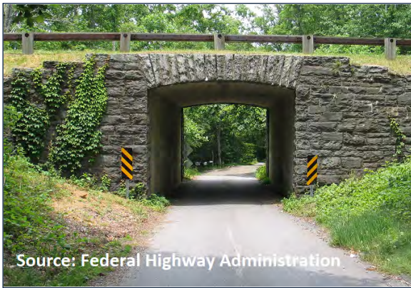
Fig. 9 Example of a non-NBIS bridge
