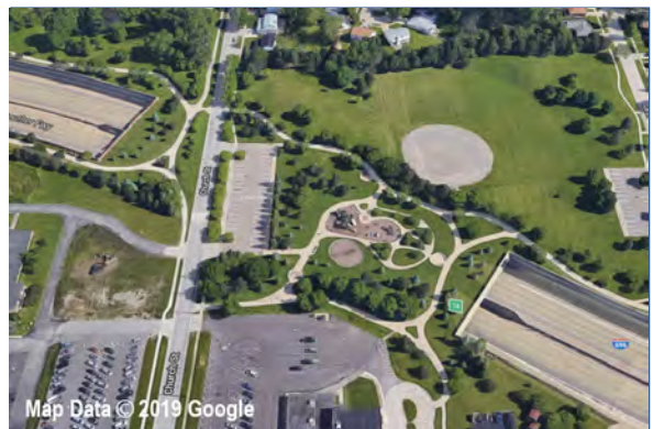
Fig. 16 Structure that may be more suitably classified as a highway tunnel
