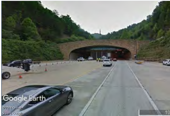
Fig. 1 Tunnel through a mountain
