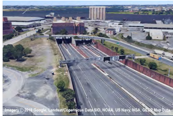
Fig. 2 Tunnel under a waterway
