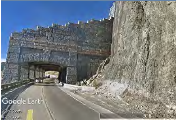
Fig 13. Example of a rock shed
