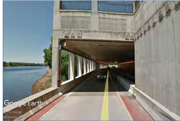
Fig 14. Example of a 3 sided structure
