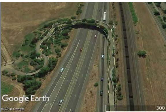
Fig. 11 Example of a pedestrian bridge
