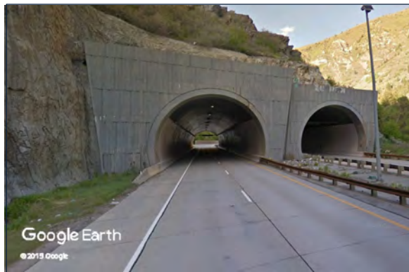
Fig. 3 Bored tunnel with lining
