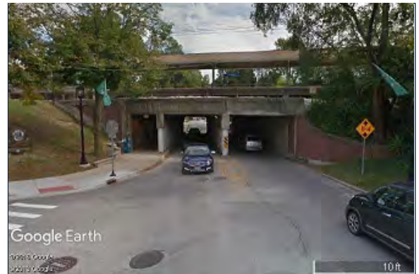
Fig. 8 Example of a railroad bridge
