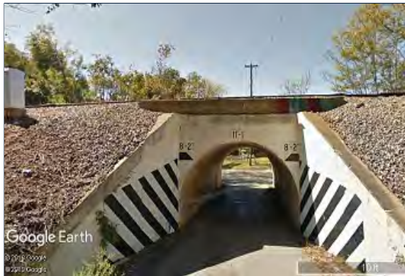
Fig. 7 Example of a railroad bridge
