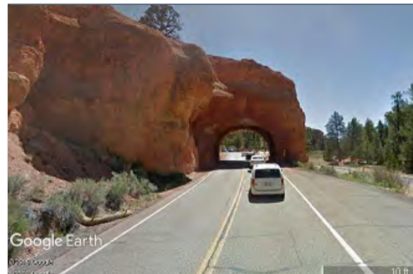
Fig. 4 Bored tunnel without lining
