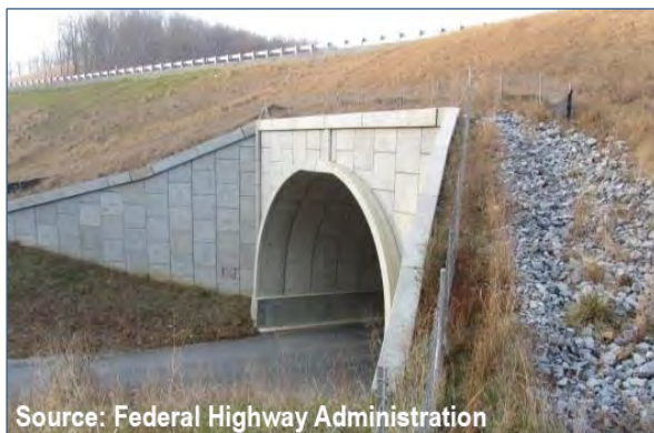
Fig. 17 Structure that can be classified as a highway bridge or highway tunnel
