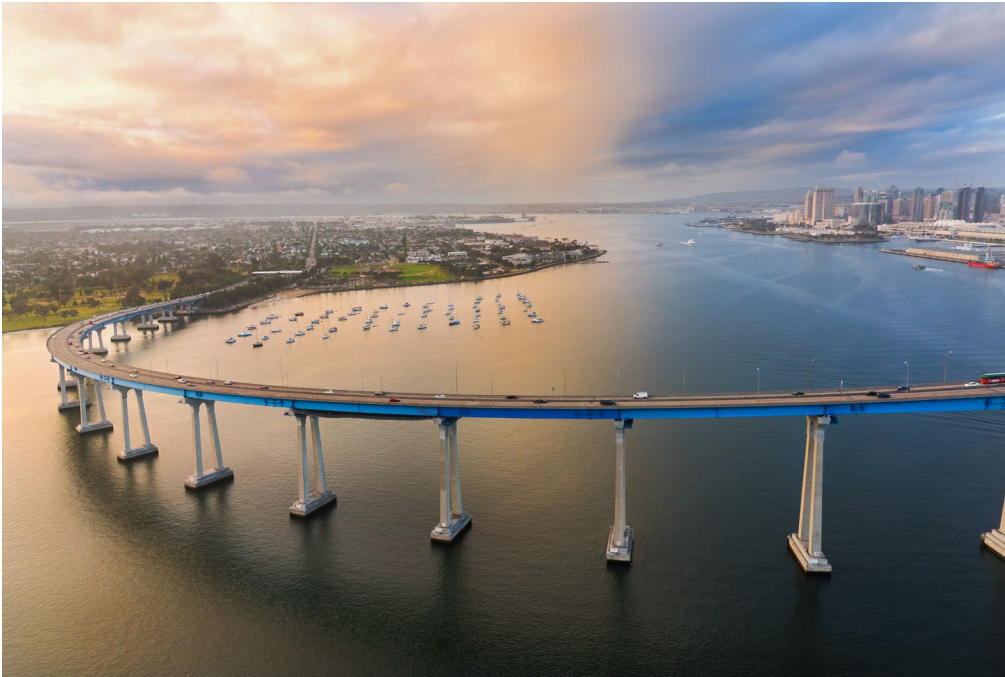
Coronado Bridge San Diego, CA
