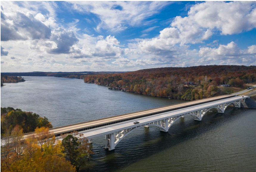
Lake Tillary Bridge, NCDOT
