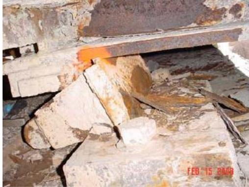
**Figure 2-6** *Photo of failed rocker bearing at Pier 10S of Birmingham Bridge Approach Span showing the rocker tipped over with girder sitting on top of failed bearing (taken from [30]).*
