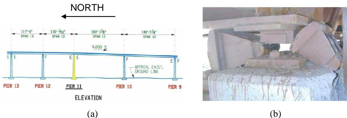
**Figure 2-5** *Dunn Memorial Bridge Interchange Rocker Bearing Failure: (a) Sketch of the bridge elevation from Pier 9 to Pier 13; (b) Photo of the failed rocker bearings at Pier 11 showing them tipped over (taken from [29]).*
