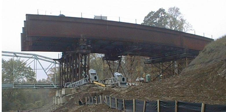
**Figure 2-10** Photo showing the use of temporary supports during erection of a curved steel I-girder bridge. The use of temporary supports help to control the geometry of the structure during steel erection.
