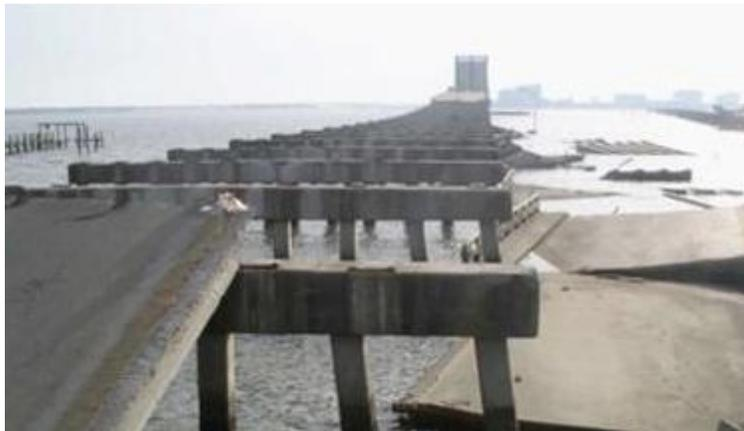
**Figure 3-6** *Photo showing the spans of the US-90 bridge completely unseated and submerged in the water due to storm surge induced loading (taken from [57]).*
