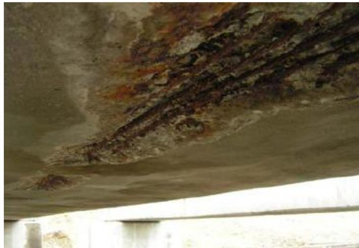
**Figure 3-3** Photo showing results of vehicle impact and subsequent corrosion damage to prestressing strands from a prestressed concrete box beam in Lake View Bridge over I-70 (taken from [43]).
