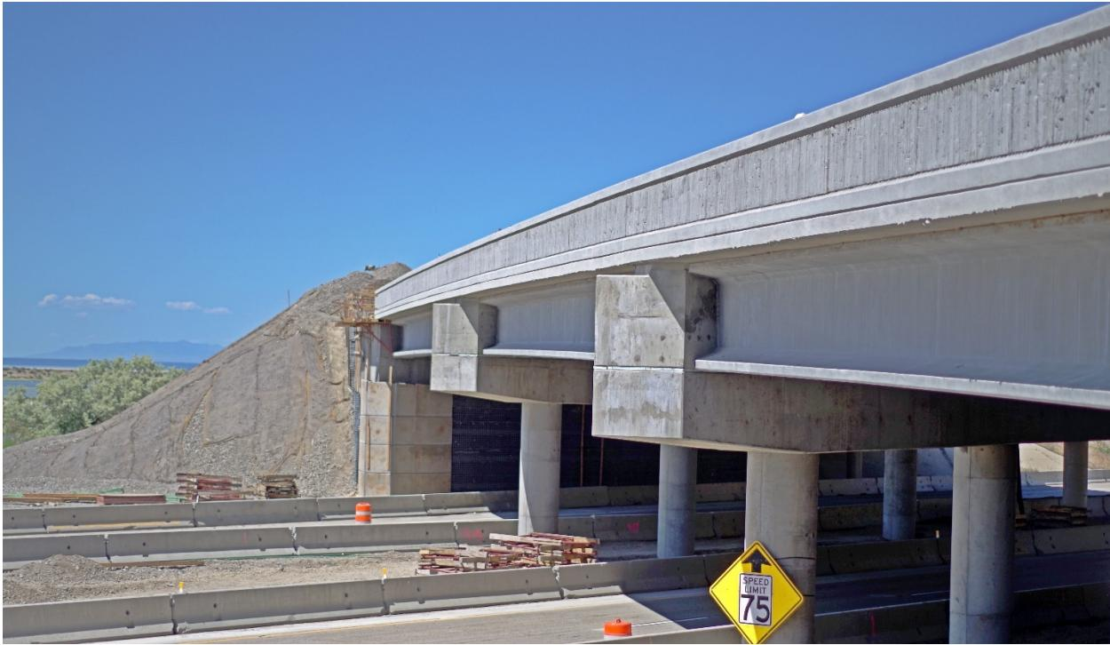
**Figure 20: Photo. The new SR-36 girders were fabricated to accommodate complex geometry.**
