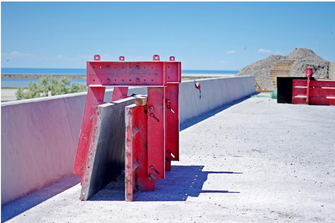
**Figure 59: Photo. Parapet form next to parapet.**
