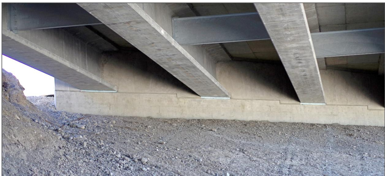
**Figure 55: Photo. Constructed abutment on SR 36 bridge.**
