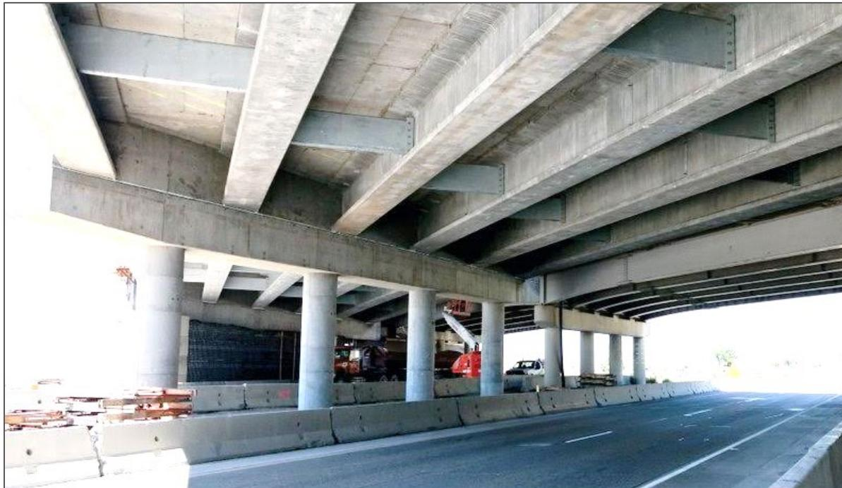
**Figure 57: Photo. Constructed pier from precast concrete bridge.**
