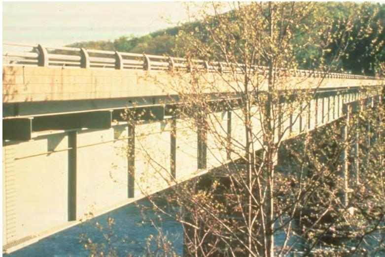
**Figure 6.6.6.2.1-1 Transverse Web Stiffeners on an I-Girder**
