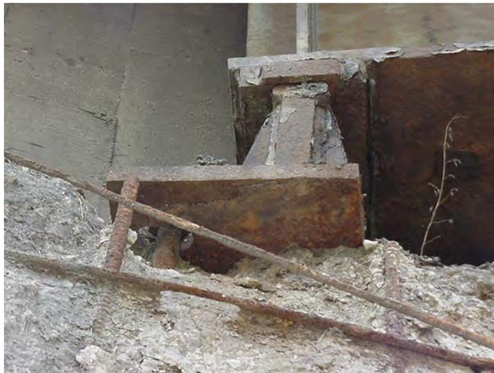
**Figure 6.3.3.3.7-2 Distressed Bearing on a Skewed Support**
