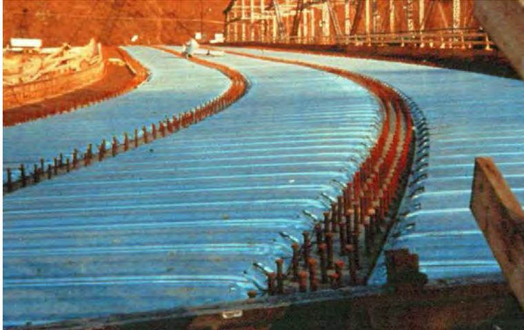
**Figure 6.6.2.1-1 Stud Shear Connectors on Steel Girders**
