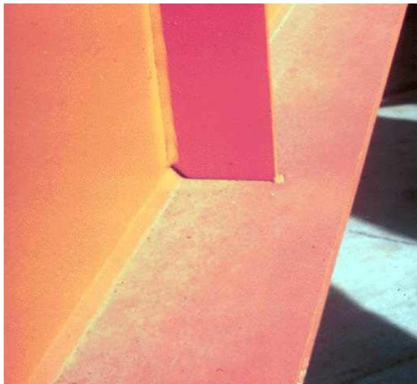
**Figure 6.5.5.2.2.1.2-1 Longitudinal Flange-to-Web Fillet Weld (Fatigue Detail Category B)**
