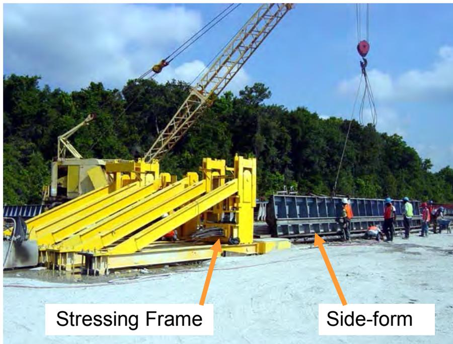
**Figure 5.10.3.1.3-2 Stressing Frame and Side Forms**
