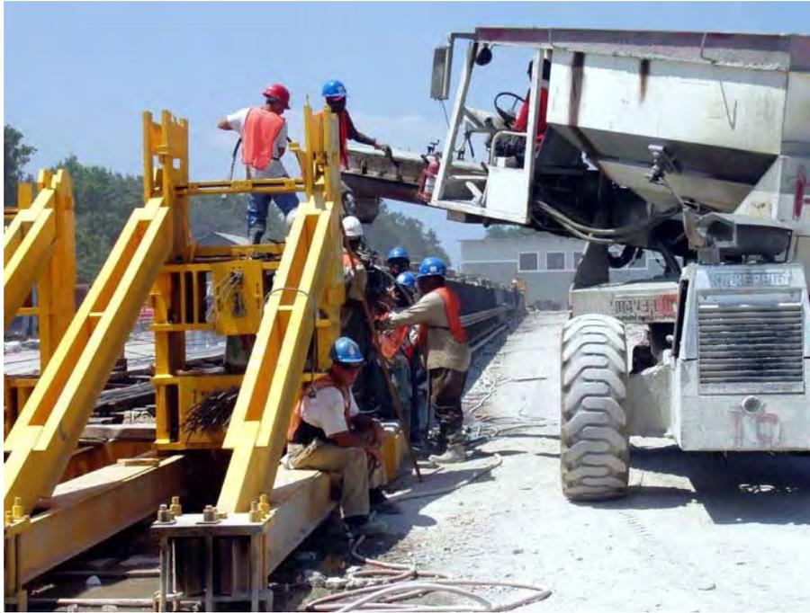
**Figure 5.10.3.1.3-3 Placing and Consolidating Concrete**
