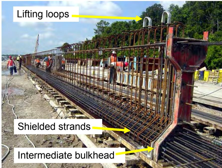
**Figure 5.10.3.1.3-1 Precast I-Girder (Type IV) Fabrication**
