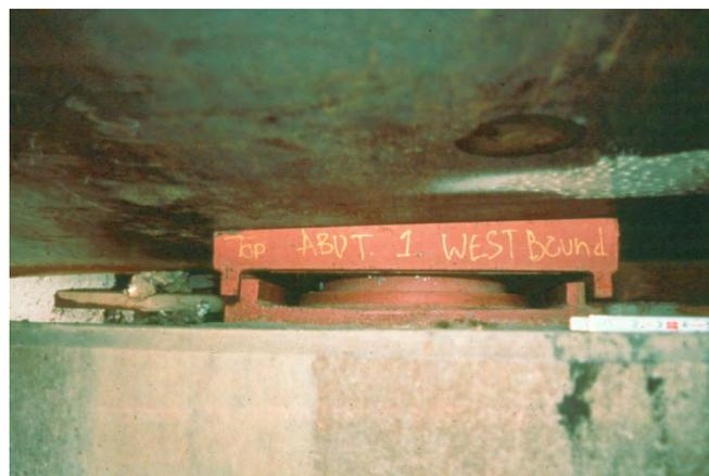
Figure 8.2.1-1 Guided Steel Pot Bearing
