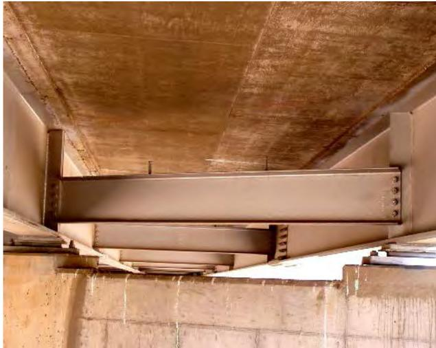
**Figure 6.3.2.9.5.1-4 Diaphragms in an I-Girder Bridge**
