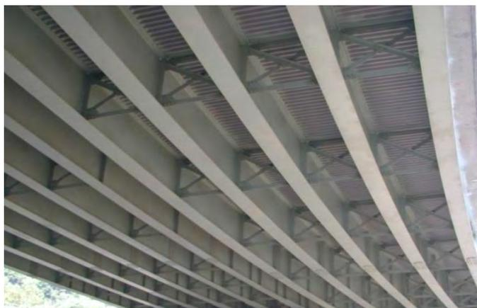
**Figure 6.3.2.9.5.1-2 X-Type Cross-Frames in an I-Girder Bridge**
