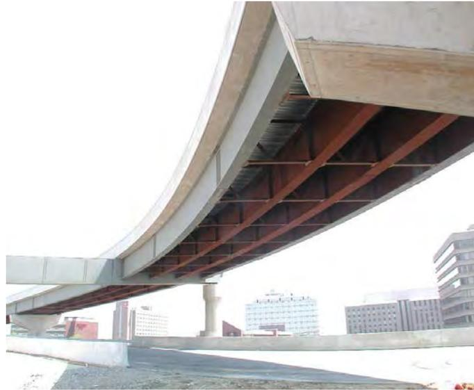
**Figure 6.3.3.3-1 Straddle Beam Supporting a Curved Steel I-Girder Bridge**
