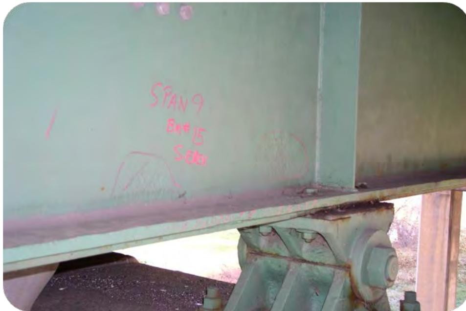
**Figure 6.6.6.3.1-1 Bearing Stiffener on I-Girder Web**
