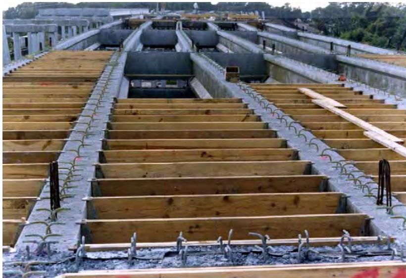
**Figure 2.3.3.4-1 Lumber Joists to Support Plywood Formwork**
