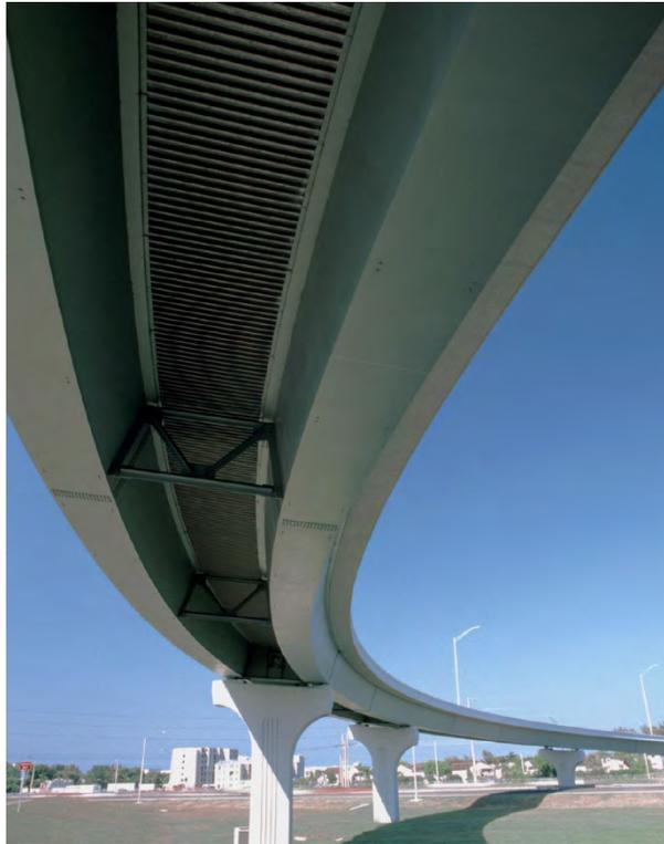
**Figure 6.3.2.11.2-1 Curved Steel Box-Girder Bridge**
