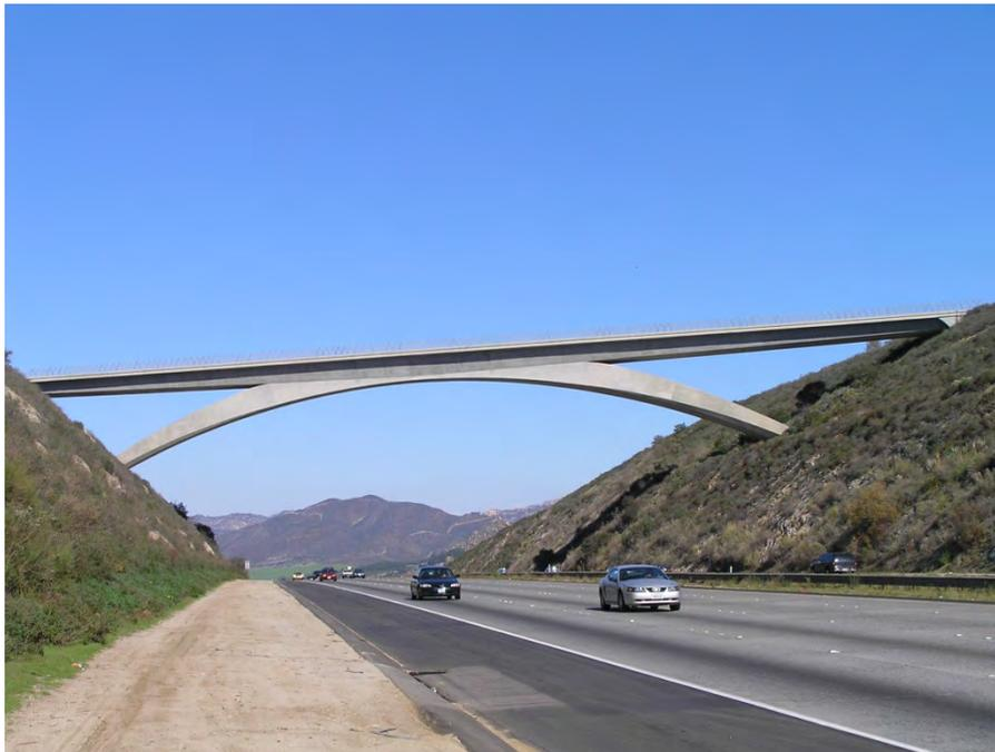
**Figure 2.3.5.2-1 Slenderness Improves the Aesthetic Quality of a Bridge**
