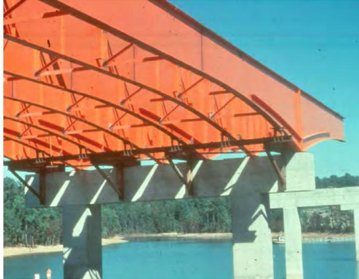
**Figure 6.3.3.2.2-2 Haunched I-Girders with a Parabolic Haunch and Longitudinal Web Stiffeners**
