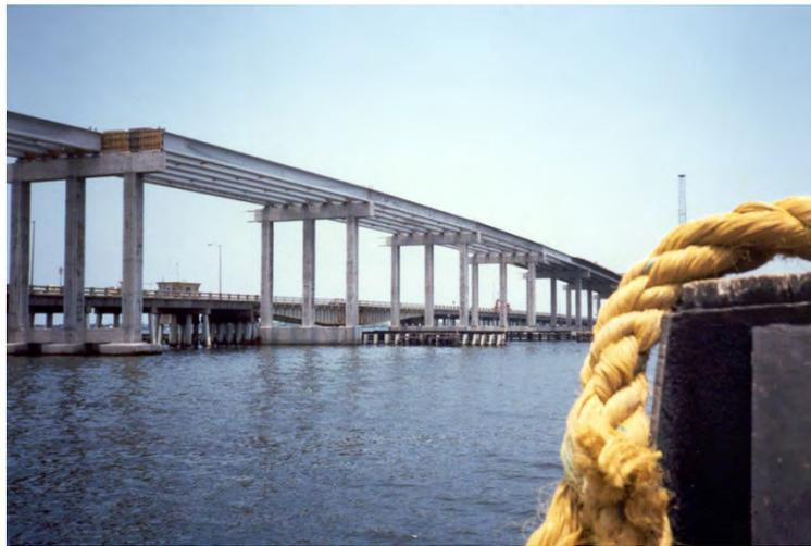
**Figure 5.10.4.2-1 Four-Span Constant Depth Spliced I-Girder**
