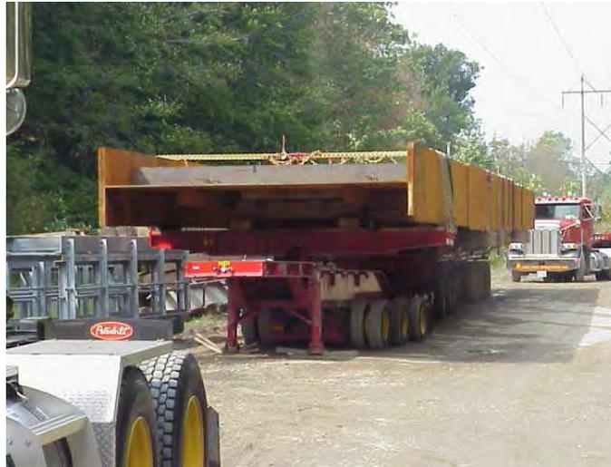
**Figure 6.3.2.4.2-1 Steel I-Girder Transported in the Horizontal Position**
