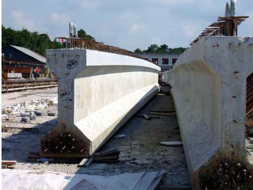
**Figure 5.5.8.1-1 Residual, Upward Deflection from Prestress and Self-weight**
