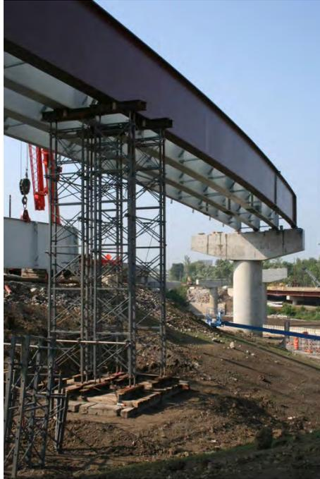
**Figure 6.4.9.4-4 Temporary Supports on Curved I-Girder Bridge**
