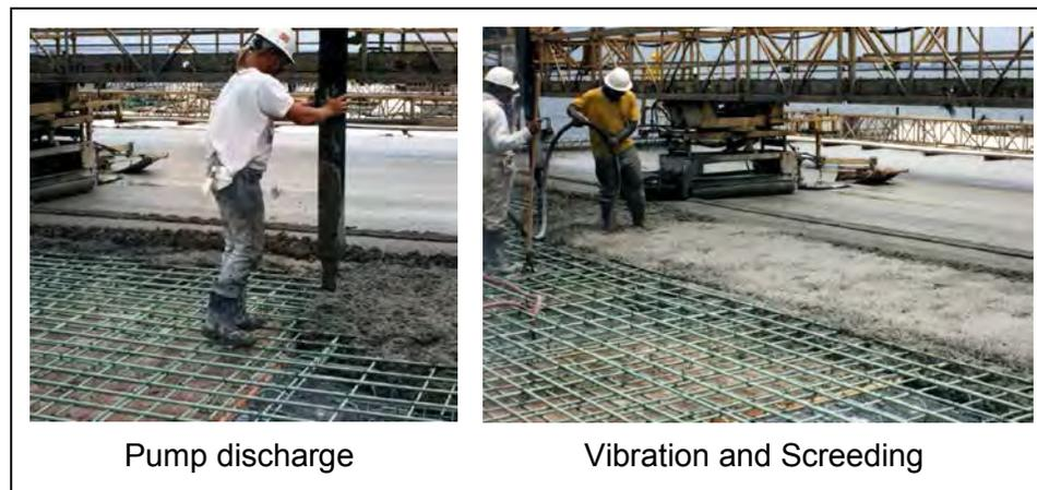
**Figure 2.3.3.6-1 Placing, Consolidating, and Screeding a Concrete Slab**
