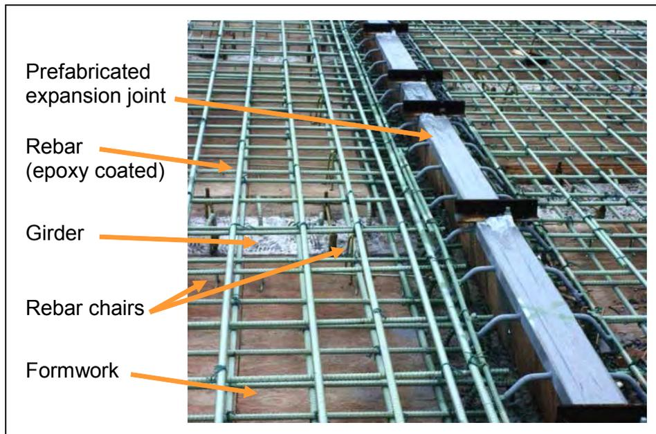
**Figure 2.3.3.5-1 Installation of Deck Slab Reinforcing Steel**
