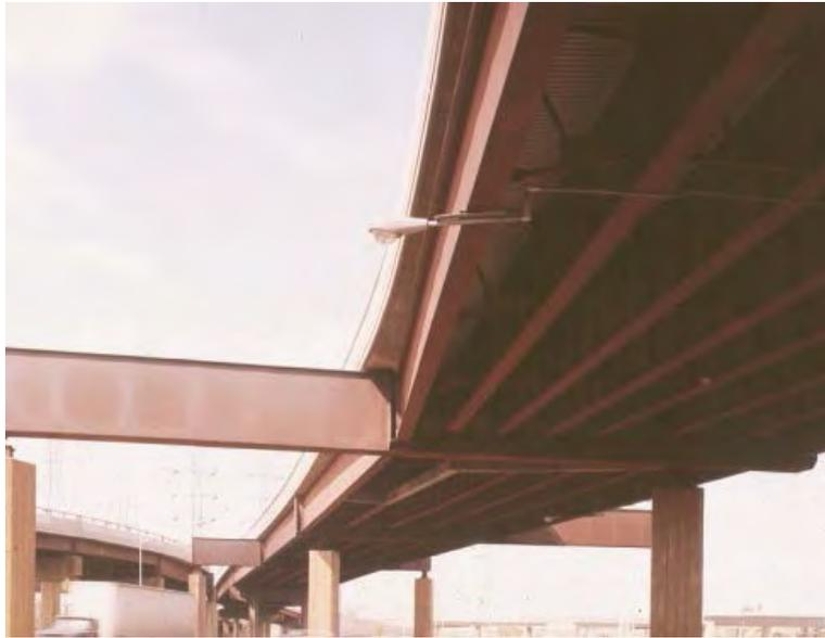
**Figure 6.4.9.2-3 Segmented Curved I-Girder Bridge**
