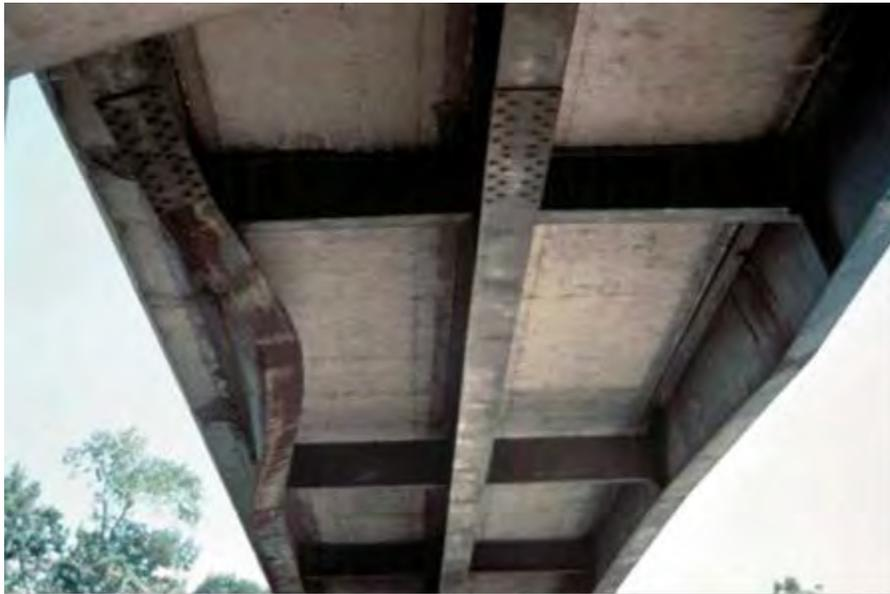
**Figure 2.2.3.2-1 Violation of Vertical Clearance Requirement**
