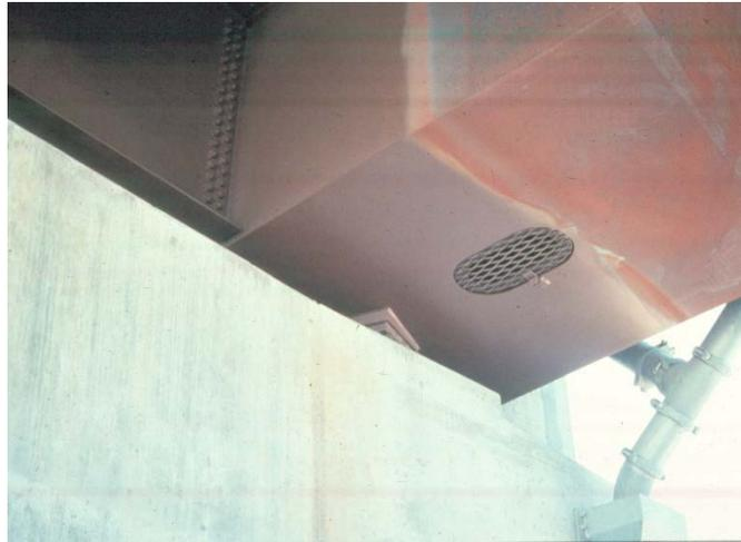
**Figure 6.4.2.3.2.3-2 Inspection Manhole in Box Girder Bottom Flange**
