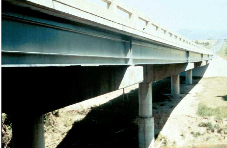
**Figure 6.6.6.4.1-1 Longitudinal Web Stiffeners on an I-Girder**
