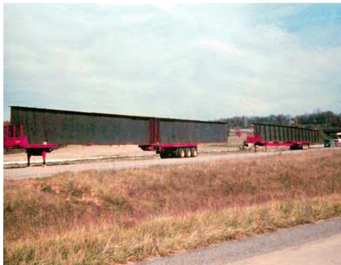
**Figure 6.3.2.4.2.1-1 Transporting Steel Bridge Girders by Truck**
