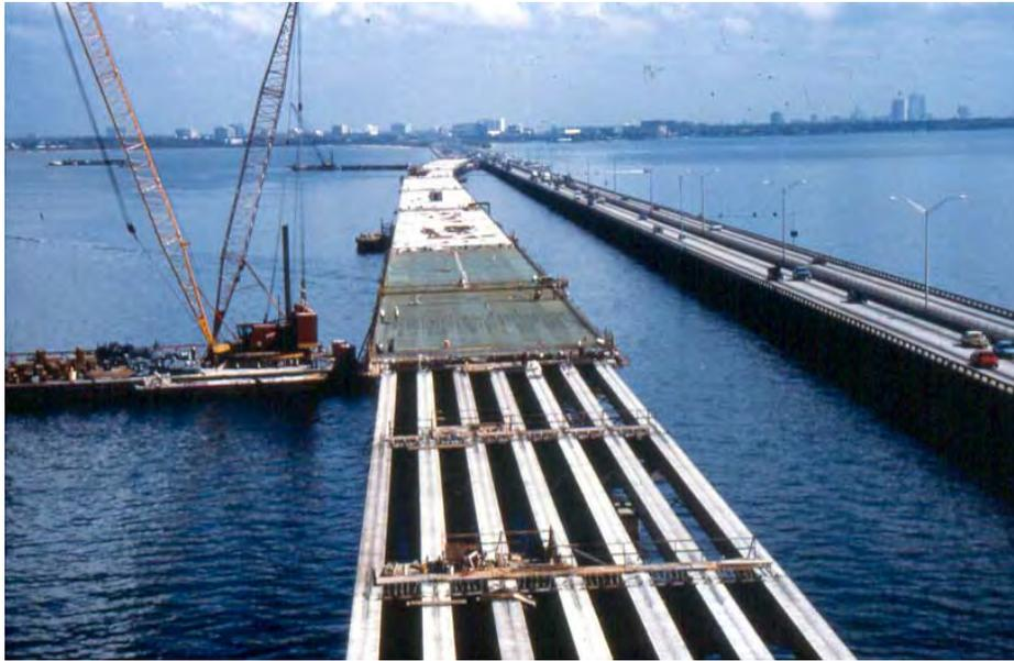
**Figure 2.3.3.1-2 Crane on Barge**
