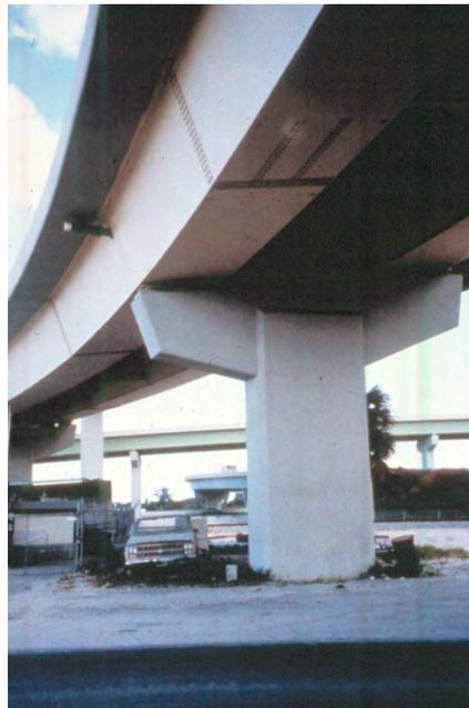
**Figure 6.4.9.5.2-1 Underside of a Two-Tub Curved Box-Girder Bridge**
