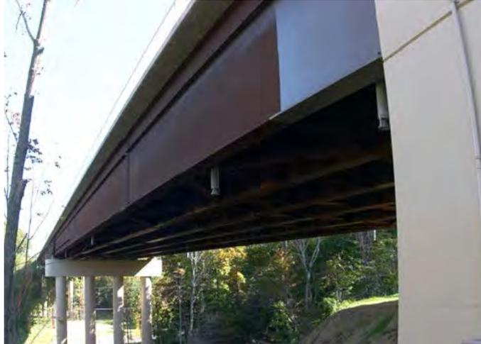
**Figure 6.4.5.5.2.2-1 I-Girder with Longitudinal Web Stiffeners**
