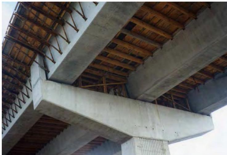
**Figure 2.3.3.4-4 Lumber Form System for Widely Spaced U-Beams**
