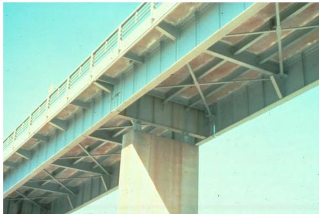
**Figure 6.3.2.5.8-1 Deck-Type Two-Girder System**
