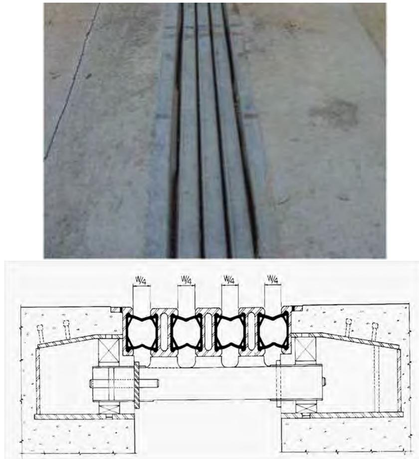
**Figure 8.3.2.3-1 Modular Bridge Joint System**
