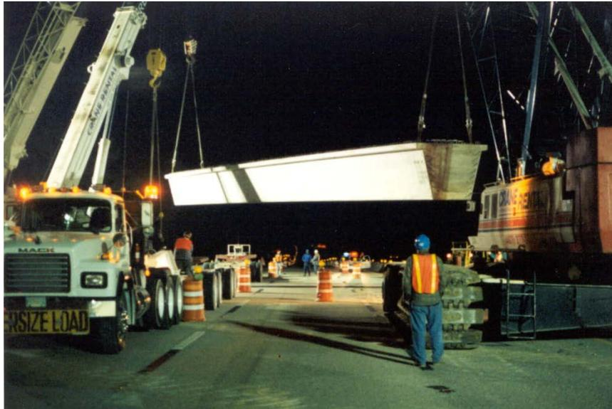
**Figure 2.3.3.1-1 Erection using Two Cranes**
