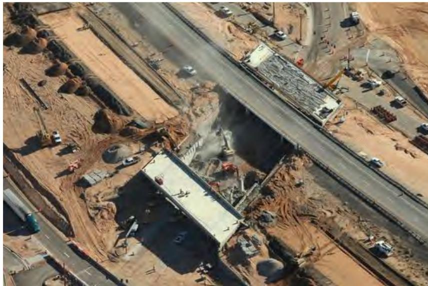
**Figure 2.4.1-1 Overhead View of a Slide-In Bridge Construction Project
