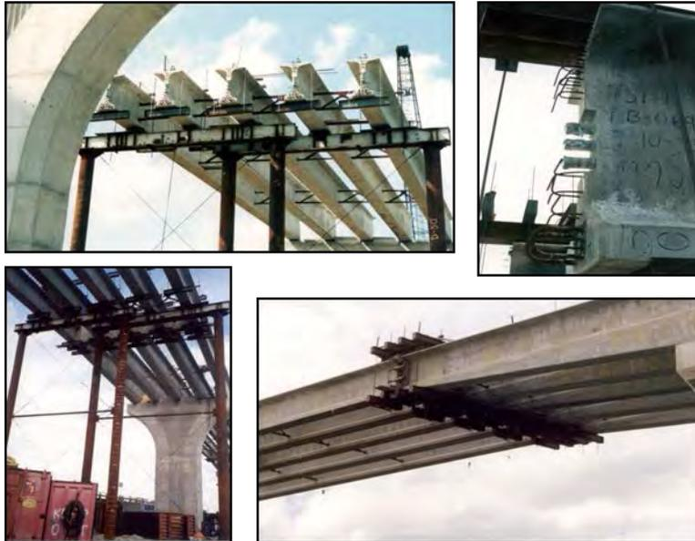
**Figure 5.10.4.2-2 Three-Span Haunched I-Girder**
