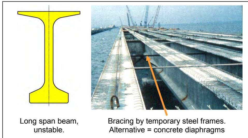
**Figure 5.10.3.1.3-4 Temporary Bracing for Construction Stability**
