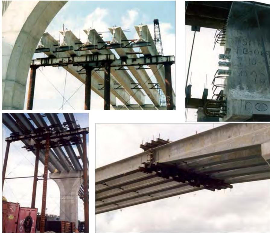
**Figure 5.4.1-4 Temporary Falsework for Spliced Girder Construction**
