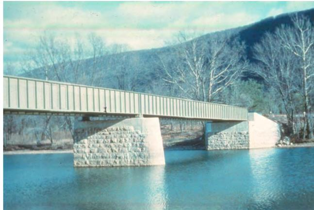
**Figure 6.3.2.5.8-2 Through-Type Two-Girder System**
