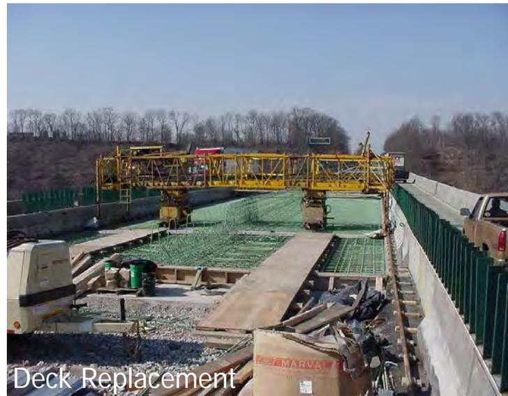
**Figure 6.3.2.5.3-1 Staged Redecking Under Traffic**
