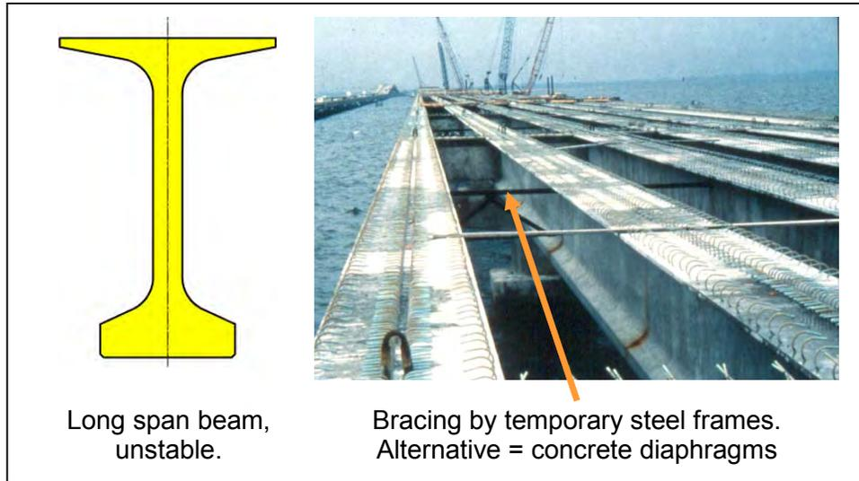
**Figure 2.3.3.3-1 Temporary Bracing for Construction Stability**
