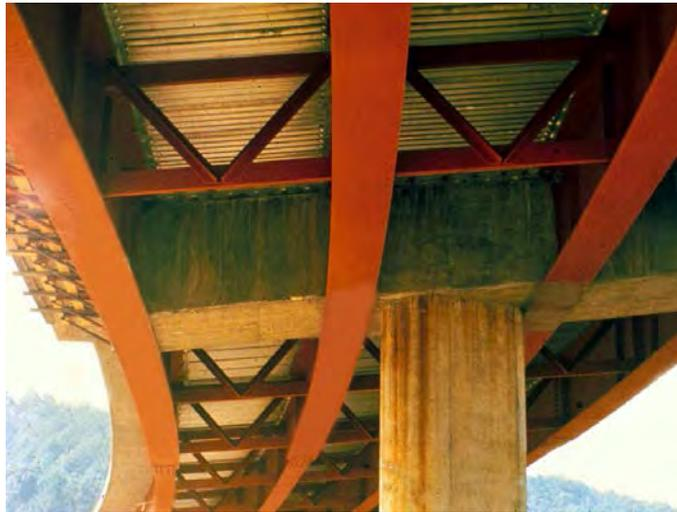
**Figure 6.3.2.9.5.1-3 K-Type Cross-Frames in an I-Girder Bridge**
