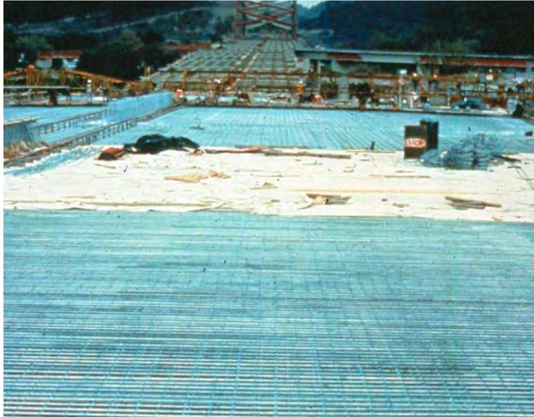
**Figure 6.5.3.3.1-1 Bridge Deck Under Construction in Sequential Stages**
