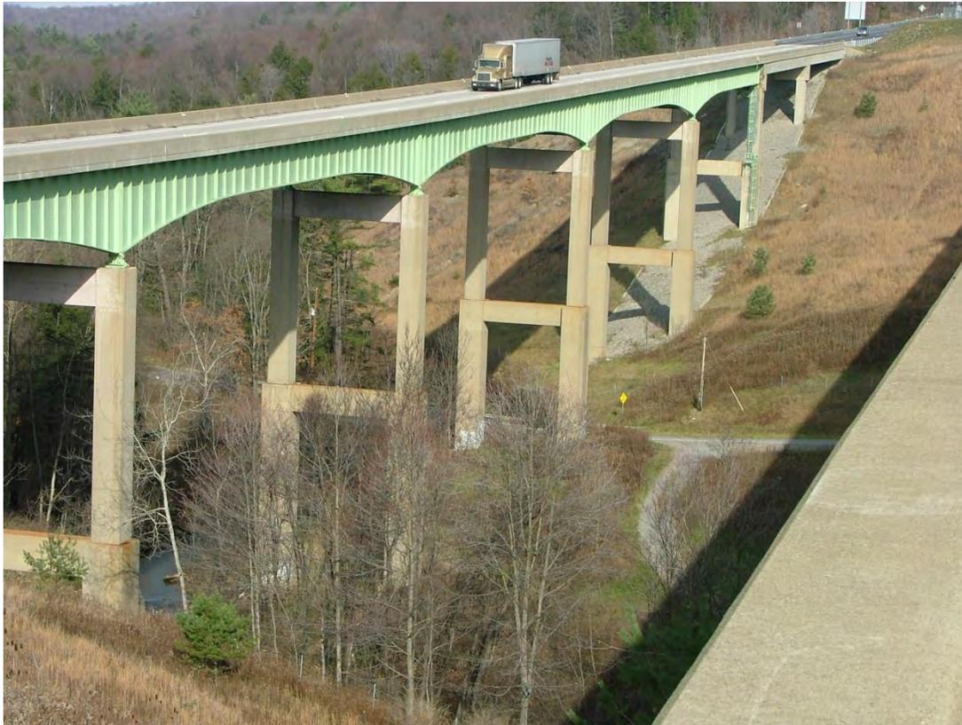
**Figure 2.3.5.5-1 Haunched Girders Can Improve the Aesthetics of the Bridge**
