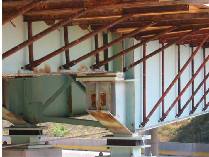
**Figure 6.3.2.6-1 Cantilevered Deck Overhang Brackets**
