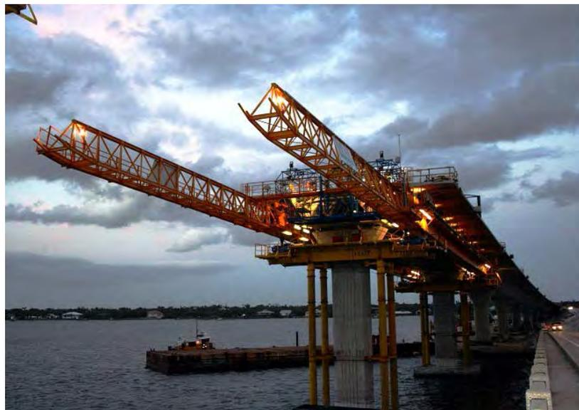
**Figure 5.4.1-5 Span-by-Span Construction using Erection Trusses**
