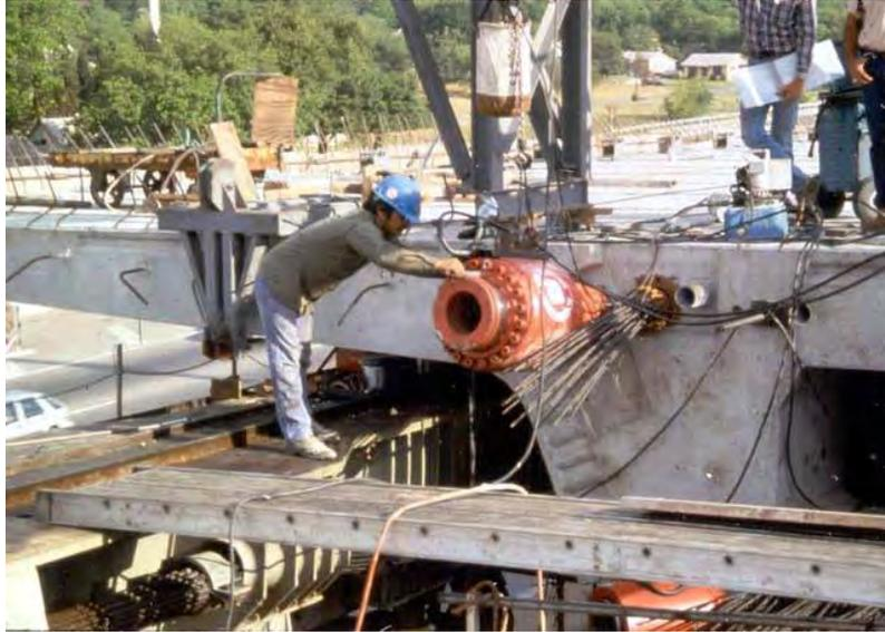
**Figure 5.3.2-3 Jacking of Post-Tensioning Tendon**
