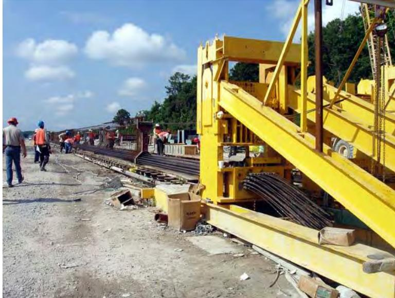
**Figure 5.3.2-2 Casting Bed for Pretensioned Girders**
