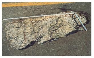
Figure 133. Typical deck spall with exposed rebar. Locations 3 and 4.
