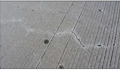
Figure 163. Closer view of cracking in wearing surface for Bridge Number 15558X.
