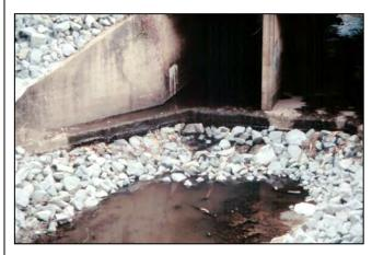
Defects: Scour and damage Severity: Moderate Extent: Widespread
