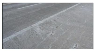
Figure 162. Longitudinal cracking in wearing surface for Bridge Number 15558X.
