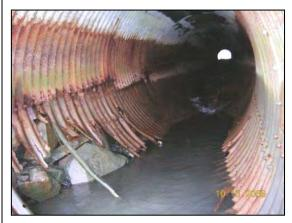
Figure 141. Corroded pipe culvert invert. Location 1 and 3. (Source: Alaska DOT)
