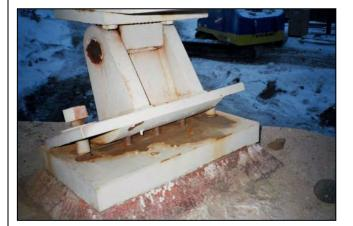
Defect: Alignment and connection Severity: Major Extent: 8 bearings (widespread)
