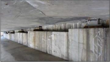
Figure 168. Cracking in south RC abutment for Bridge Number 15558X.
