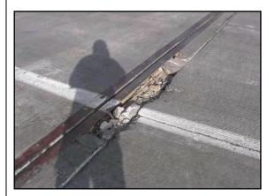
Defect: Adjacent deck or header Severity: Moderate Extent: 6' of one joint (isolated)
