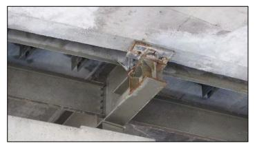
Figure 165. Surface corrosion on cantilever steel beam ends for Bridge Number 15558X.
