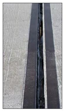
Figure 177. Strip seal ripped and punctured completely through for Bridge Number 15558X.
