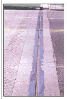
Defect: Debris impaction Severity: Minor Extent: All joints (widespread)
