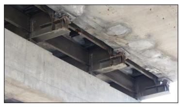
Figure 174. Typical pot bearings with surface rust for Bridge Number 15558X.
