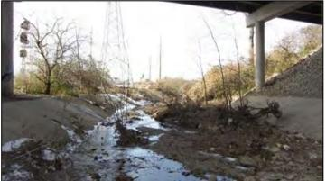
Figure 178. RC lined channel with debris and vegetation for Bridge Number 15558X.
