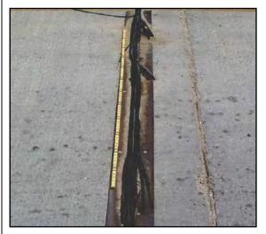
Defect: Seal damage Severity: Moderate Extent: All joints (widespread)
