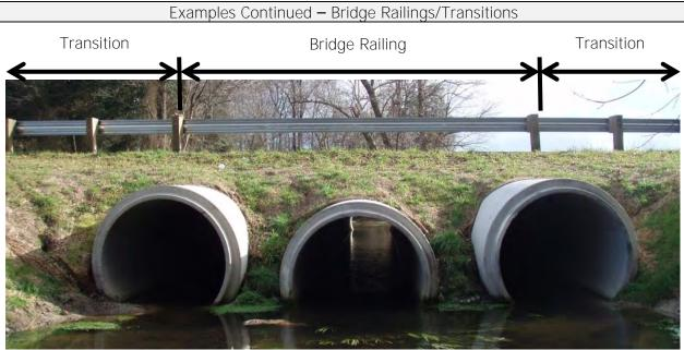
Figure 12. Metal bridge railing and transition for long-span application. (Source: Delaware DOT)
