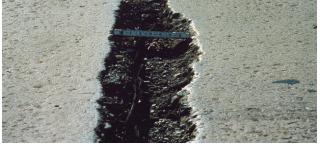
Figure 132. Deck spalling along joint. Location 2.
