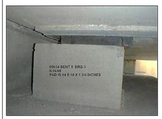
Defect: Loss of bearing area Severity: Moderate Extent: 20% of bearings (some)
