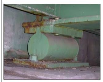
Defect: Corrosion Severity: Minor Extent: All bearings
