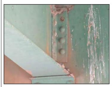
Figure 136. Missing rivets in stringer-to-floor-beam connection. Location 4. (Source: Colorado DOT)
