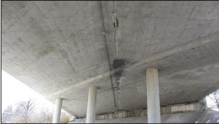
Figure 166. Spalls with exposed rebar on underside of RC voided slab for Bridge Number 15558X.
