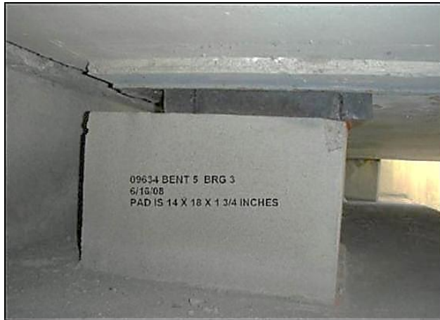
Figure 144. Loss of bearing area for elastomeric bearing. (Source: Oregon DOT)
