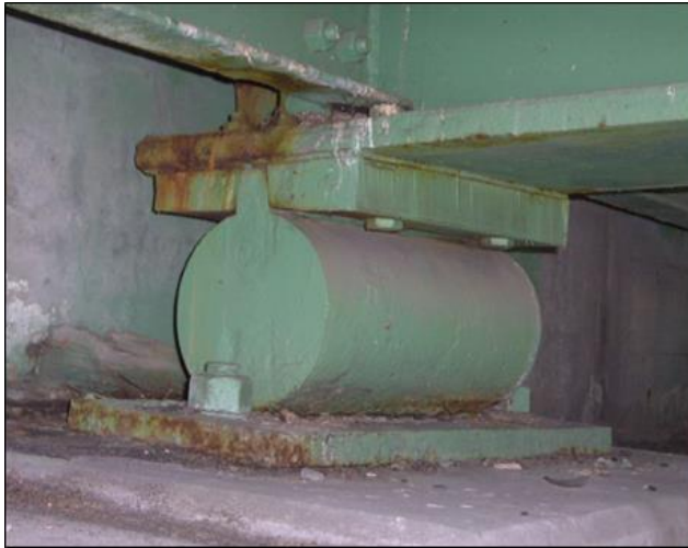
Figure 146. Surface rust on moveable bearing.
