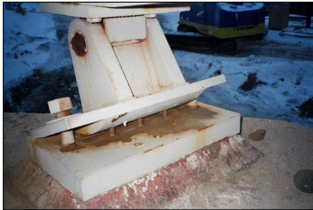
Figure 145. Misaligned rocker bearing. (Source: Alaska DOT)
