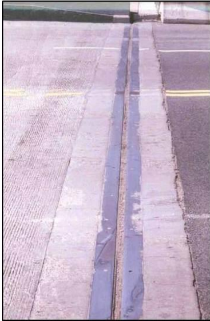
Figure 147. Joint partially filled with debris.
