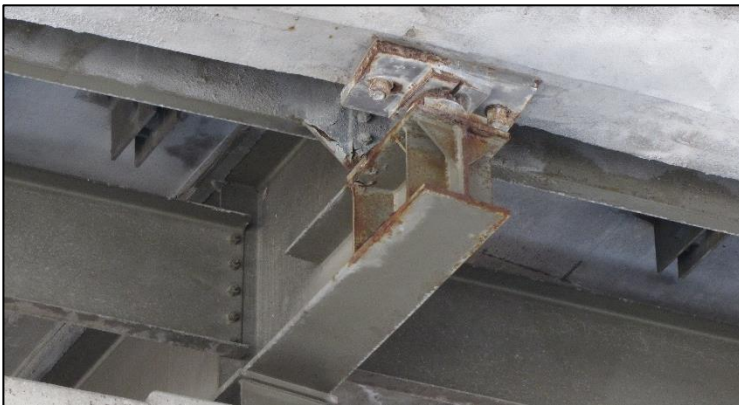
Figure 175. Closer view of typical pot bearings with surface rust for Bridge Number 15558X.
