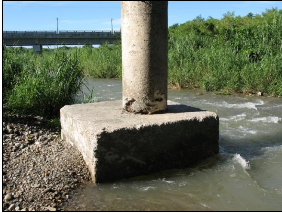
Figure 153. Exposed column footing in stream.
