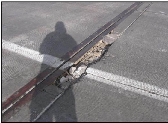
Figure 148. Spall in joint header. (Source: Colorado DOT)
