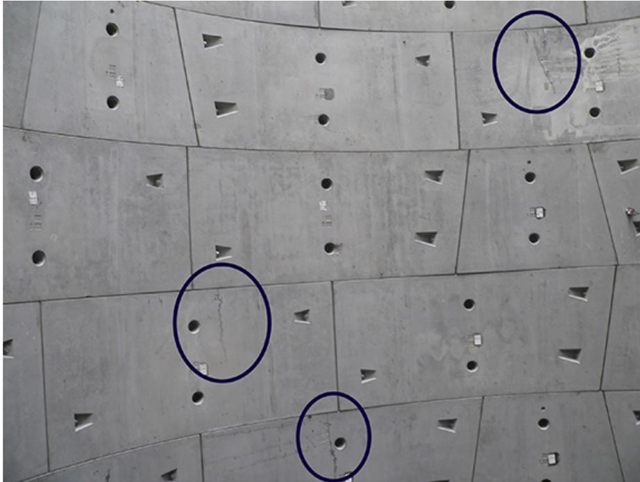
**Figure 1-6: Observed segment cracking in precast segmental lining.**
