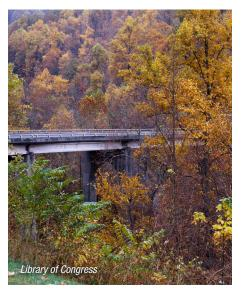
Linn Cove Viaduct (left) was the first precast concrete segmental structure to be built with the progressive placement erection method in the United States. It contains nearly every type of highway construction within its length. With its superelevation of up to 10 degrees and its tight horizontal and spiral curves, it was the most complicated bridge of its type built up to that time.
