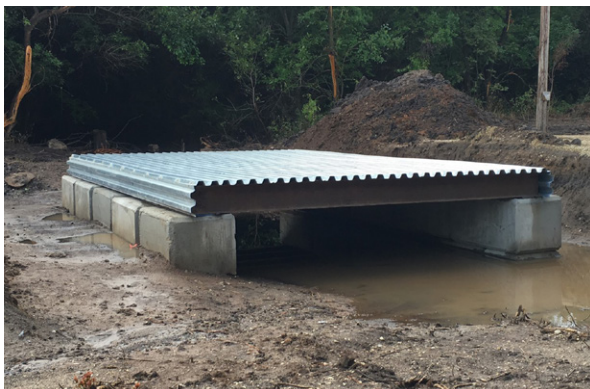
© 2021 Saline County Road and Bridge, Kansas
