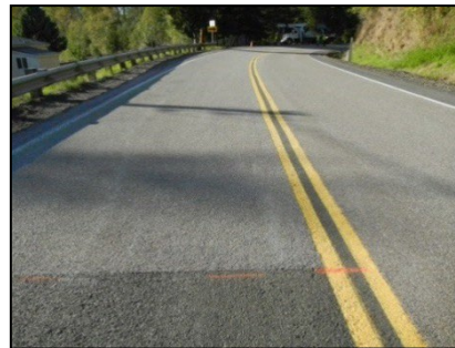
Figure 12: Completed High Friction Surface Treatment on Winoossee at Milepost 1.4 Source: National Park Service
