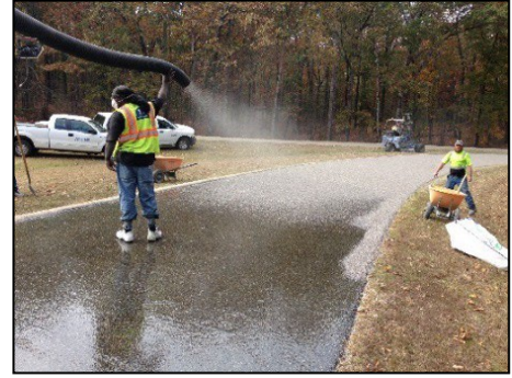
Figure 16: Applying the Aggregate
