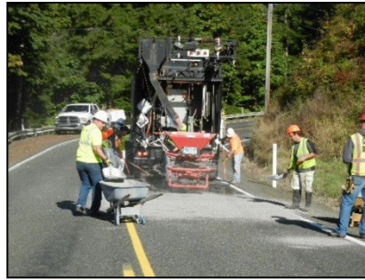
Figure 10: Distributing Aggregate Source: National Park Service
