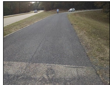
Figure 12: Completed High Friction Surface Treatment on Natchez Trace
