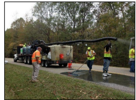
Figure 14: Semi-Mechanical High Friction Surface Treatment Application
