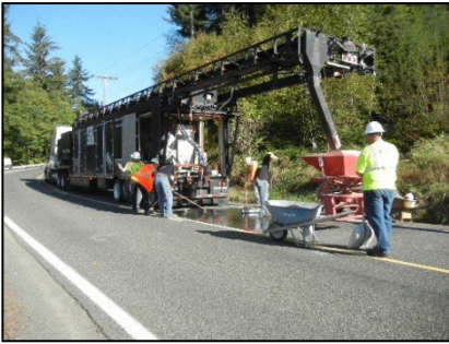
Figure 9: High Friction Surface Treatment Mechanical Application Truck Source: National Park Service
