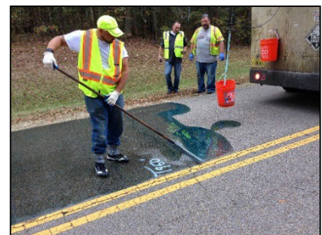
Figure 15: Spreading the Binder
