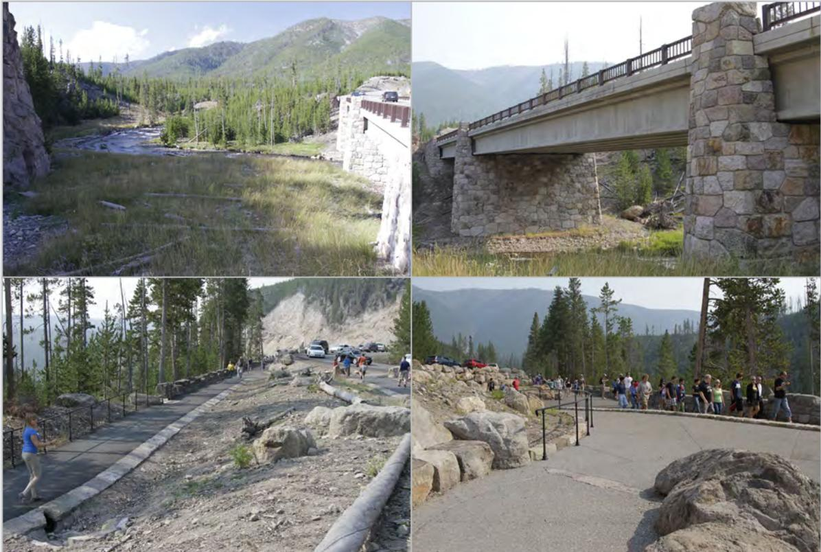
**Top left:** Little evidence exists of the former roadway alignment along the Gibbon River. **Top right:** New alignment with retaining walls of native stone and bridge over the Gibbon River. **Bottom left and right:** An expanded parking area and pedestrian pathways provide access to the falls viewing area.
