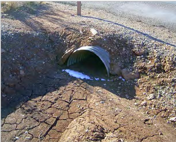
*Figure 4-2: Example of a culvert clogged by sediment
