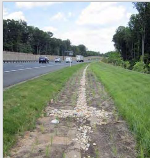
*Infiltration swale after construction*
