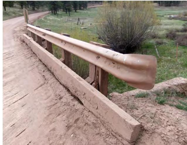
*Figure 4-3: Example of a guardrail not meeting safety requirements
