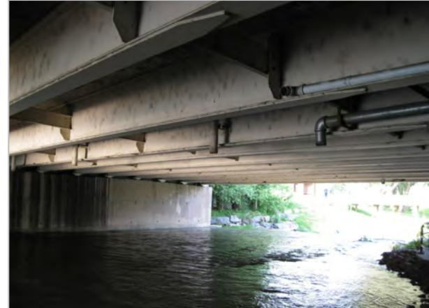
Figure 3-17: Drainage directly into a creek without treatment/infiltration strategies
