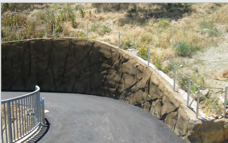
*Soil-nail wall system as constructed*
