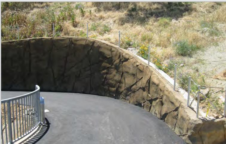
*Soil-nail wall system as constructed*
