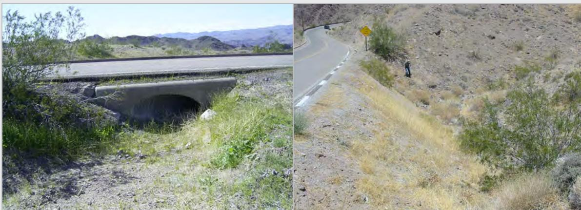
*Left: culvert entrances located within clear zone, creating a hazard for motorists. Right: steep side slopes without guardrails.*
