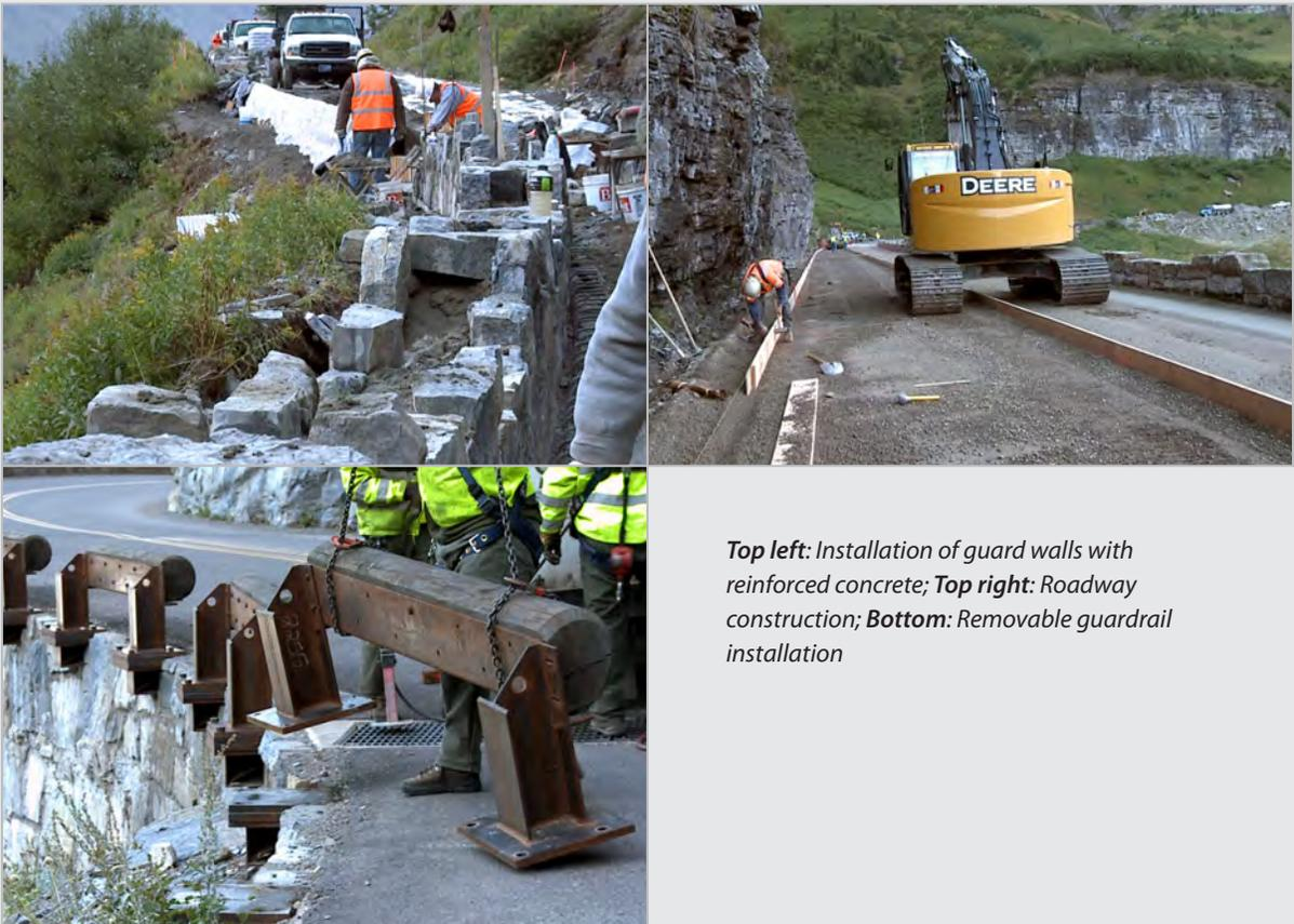
*Top left: Installation of guard walls with reinforced concrete; Top right: Roadway construction; Bottom: Removable guardrail installation*
