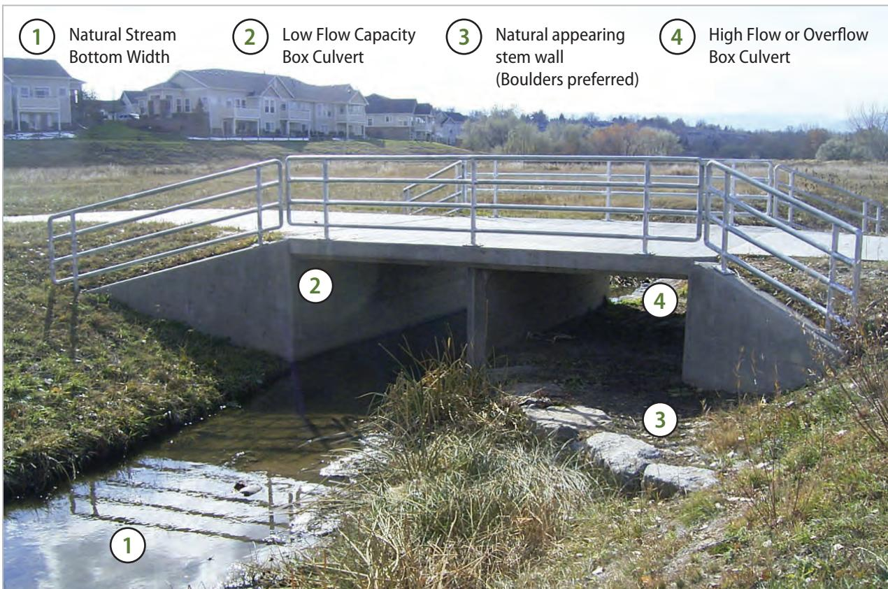
Figure 3-21: Multi-cell box culvert
