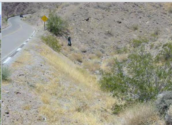
*Left: culvert entrances located within clear zone, creating a hazard for motorists. Right: steep side slopes without guardrails.*
