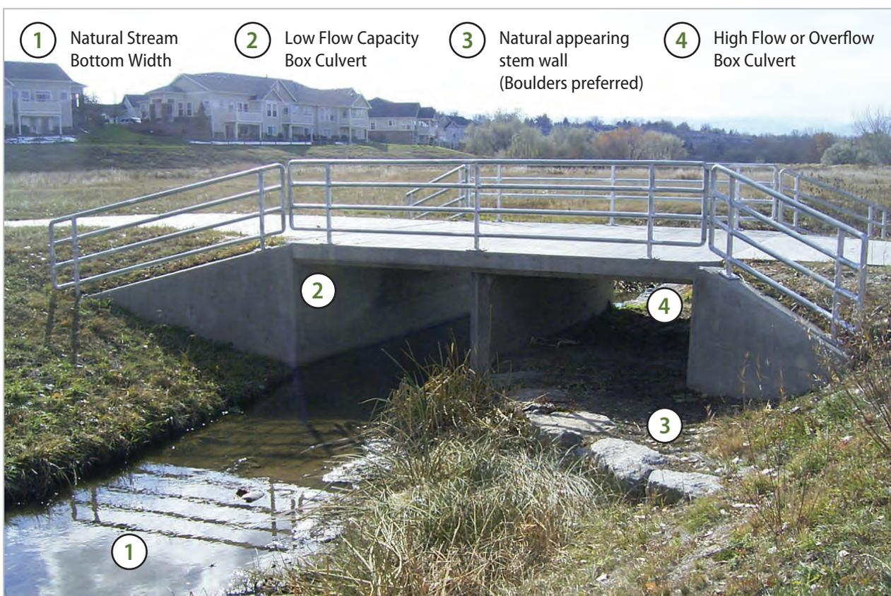
**Figure 3-21: Multi-cell box culvert**
