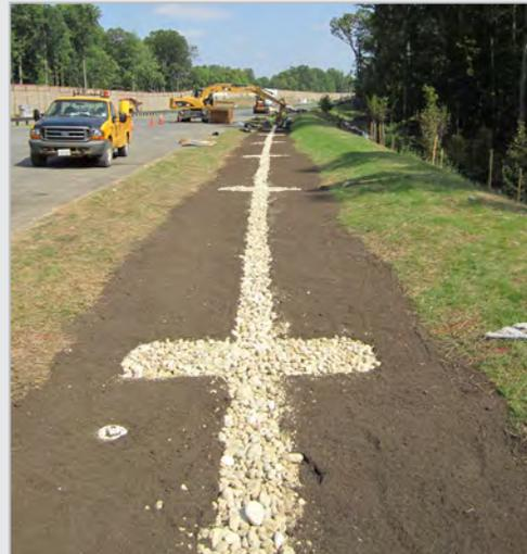
*Infiltration swale during construction*
