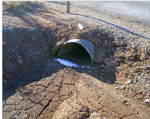
[Figure 4-2: Example of a culvert clogged by sediment](#)
