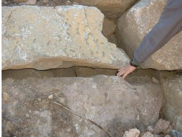
**Figure 68. Photograph. Example of an unacceptable rock bearing.**
