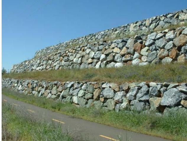
**Figure 22. Photograph. Three-tier, 9.1-m-high (30-ft-high) MSE slope with protecting rockery facing, in Folsom, California (2003).**
