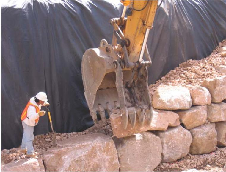
**Figure 63. Photograph. Placement of facing rocks using an excavator with a “thumb.”**
