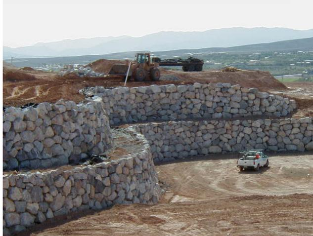
**Figure 20. Photograph. “Protecting” rockery used as a facing for a 9.1-m-high (30-ft-high) MSE wall with a 5.5-m (18-ft) maximum tier height in Henderson, Nevada (2001).**
