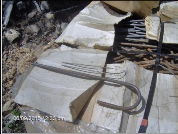
7. Anchor TRM to ground with stakes or rebar
