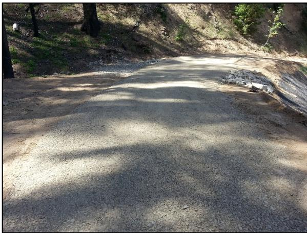
9. Surface the road dip and place riprap at outlet
