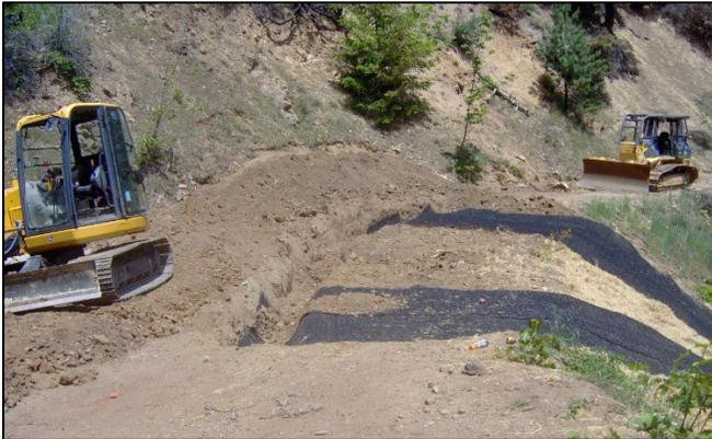
4. Backfill/compact anchor trench
