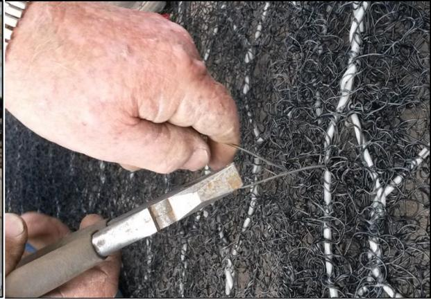
8. Tie TRM panels together with wire ties or gabion clips
