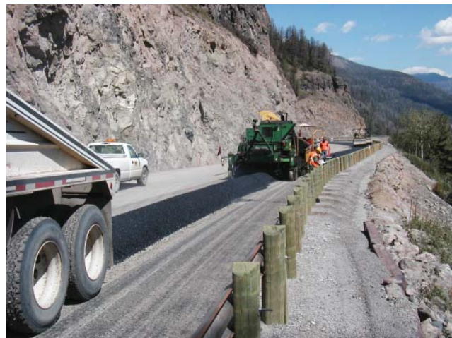
Figure 7 ~ Advera WMA deposited in windrow.
