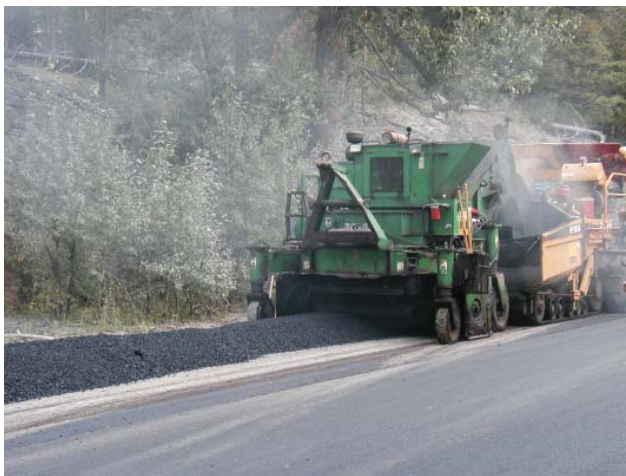
Figure 2 ~ Control mix placement.
