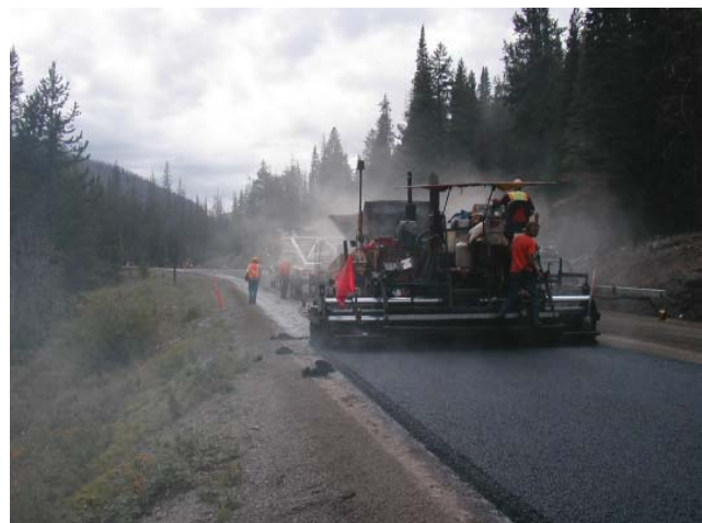
Figure 5 ~ Control mix laydown.
