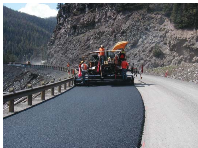
Figure 8 ~ Advera laydown operation.
