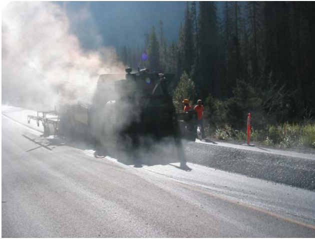
Figure 4 ~ Control mix paving operation.
