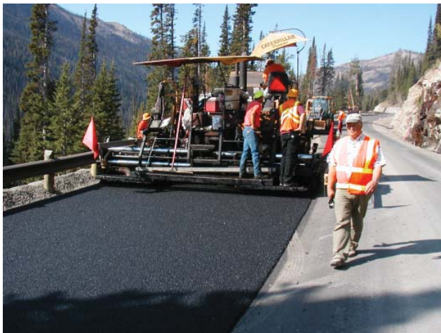
Figure 10 ~ Sasobit laydown operation.
