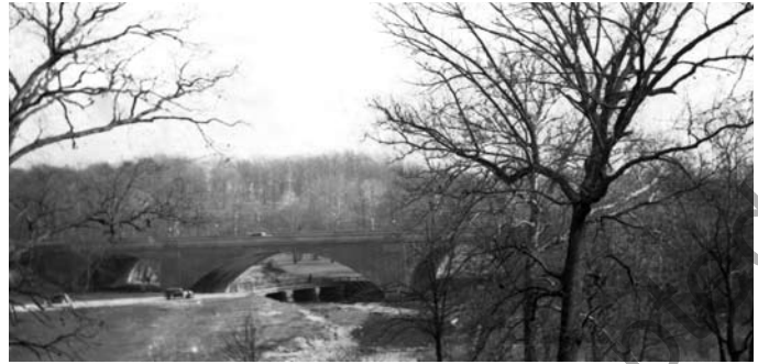
Harford Road Bridge, 1938.
