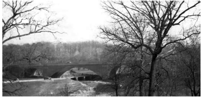
Harford Road Bridge, 1938.
