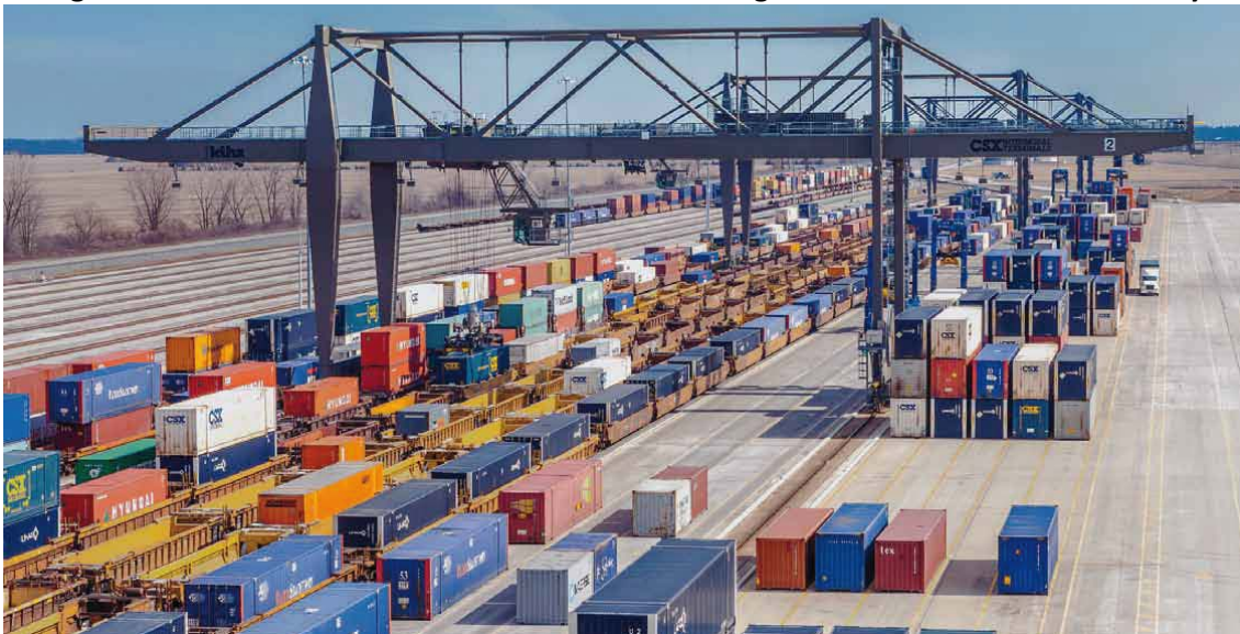
Figure 3: Kuenz of Germany RMG Crane at CSX's Northwest Ohio Intermodal Terminal
