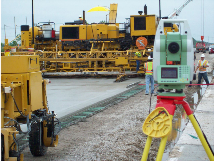
Figure 1. Concrete paving operation with AMG using special provision 12SP-824A-03.
