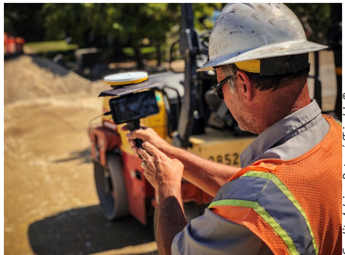
Figure 4: A hand-held augmented reality device in use on the 9000 South project.
