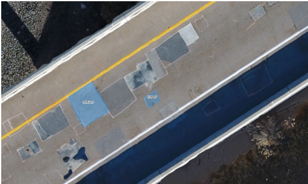
Figure 3. Location of delamination areas and structures can be documented using imagery GPS coordinates. Source: UDOT
