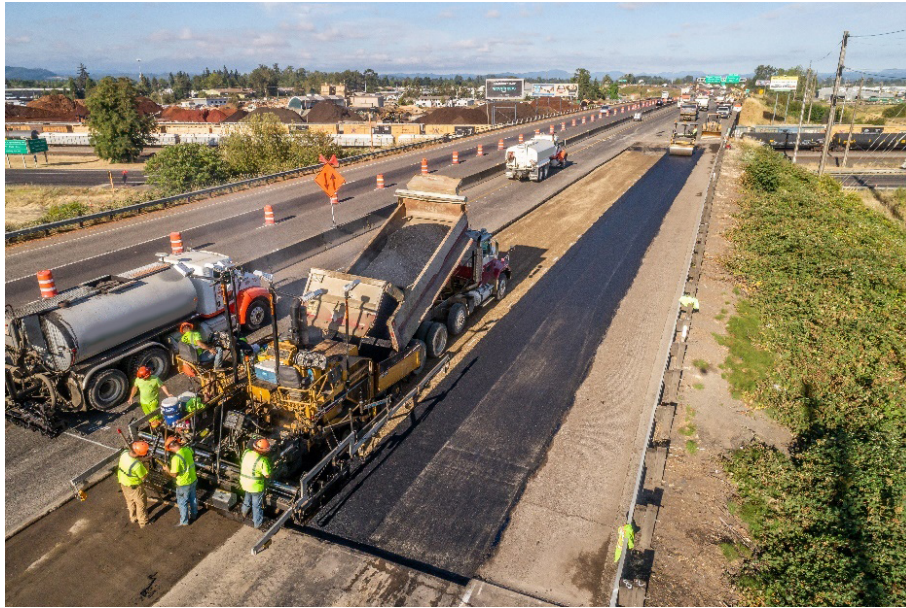
Figure 5. UAS mission to monitor construction progress. Source: ODOT
