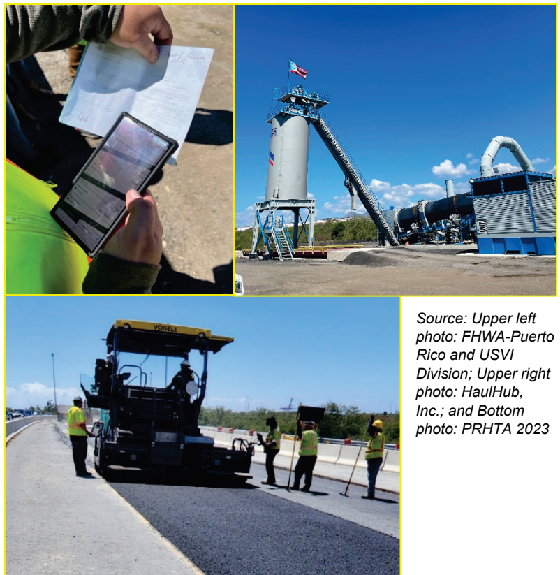
Figure 14. e-Ticketing process applied to the design, delivery, and compaction of Warm Mix Asphalt in Puerto Rico
