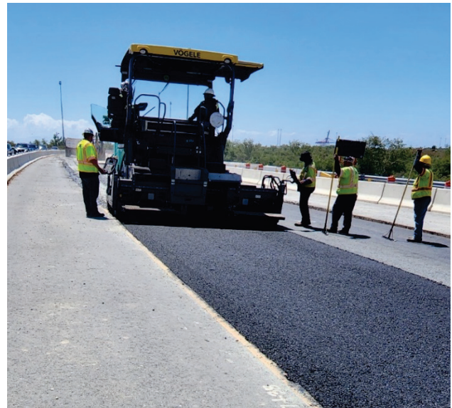
Figure 5. Placement of Asphalt Mix in PR-52, Ponce, Puerto Rico
