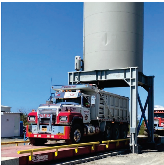
Figure 4. Truck loading at the Super Asphalt Pavement Corporation Plant, Peñuelas, Puerto Rico
