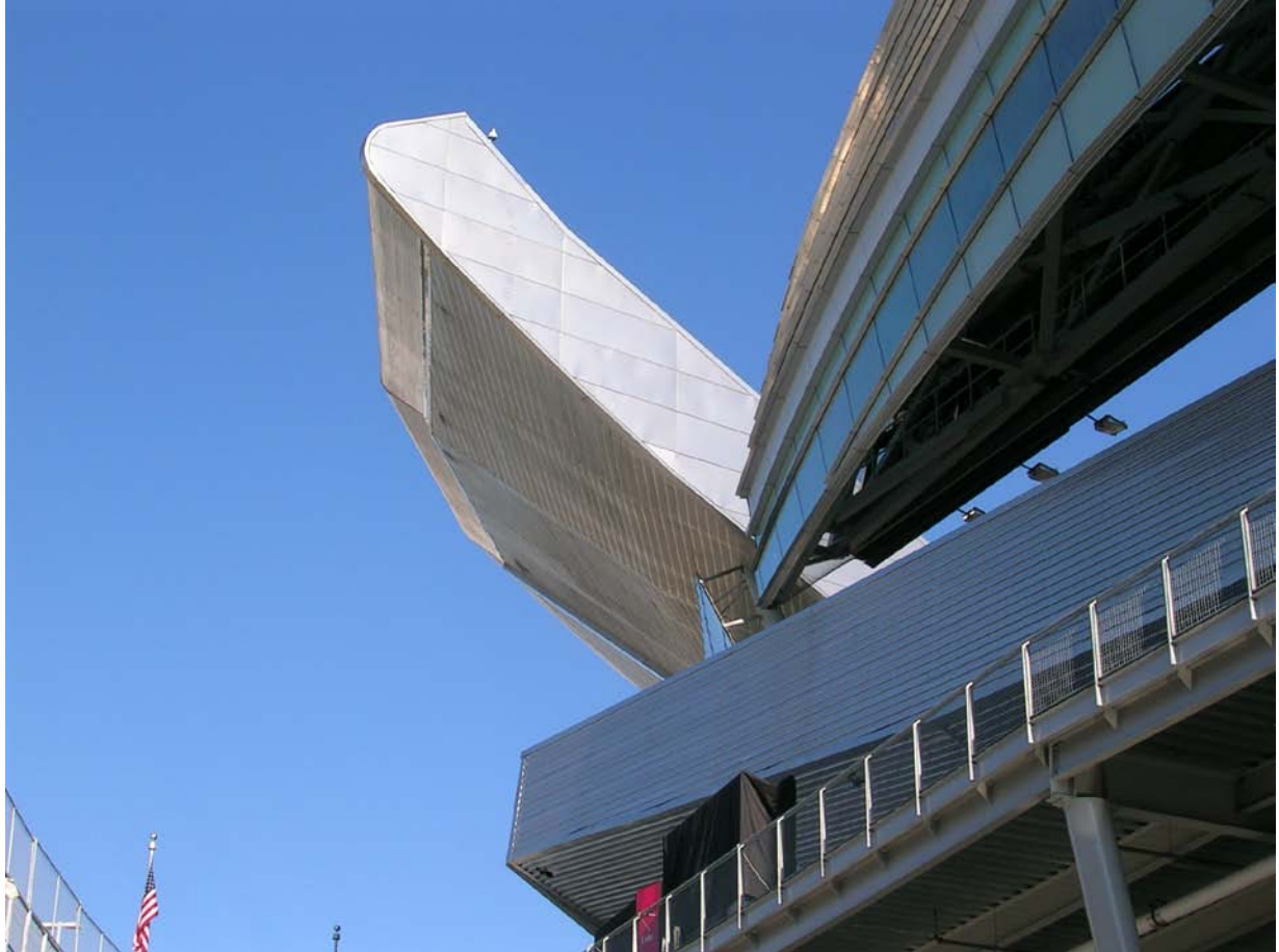
Cantilevered seating, Soldier Field Stadium
