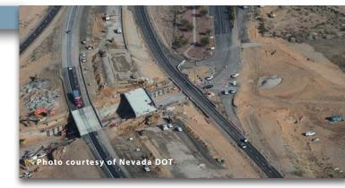
One common method used for SIBC is to push or pull the bridge superstructure across a smooth horizontal surface on pads, rollers, or rails using a hydraulic jack. In some cases, a new bridge superstructure has been pulled into place using cables attached to an electric drum or threaded bars. The decision to use jacks or cables to push or pull the bridge depends on a number of factors including terrain, bridge design, and contractor preference.
