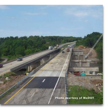
**Quality**. The use of a pre-constructed superstructure can improve quality by eliminating deck construction joints and girder camber problems associated with phased construction. In addition, it is possible to get a better concrete cure when the superstructure is constructed off-line.
