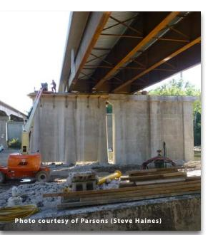
Pads are a simple and low-cost solution that allows the use of an unguided system that will not bind if the ends of the bridge move at different rates. Continual lubrication of the pads is critical during the slide, and a variety of biodegradable lubricants are available; an often-used substance is common dish soap.
