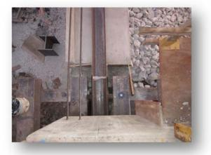
To ensure the proper jacks will be supplied to the project, the engineer must make a good estimation of the friction forces during the slide. These forces should be verified during the rehearsal slide.
