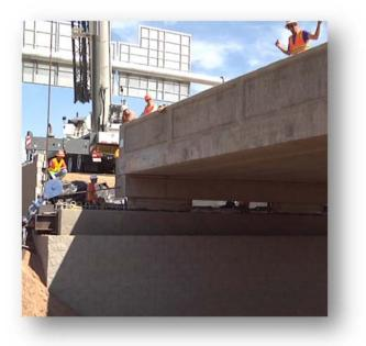
Slide-in bridge construction, and ABC in general, is primarily used for bridge replacement projects where the impacts to mobility are significant.
