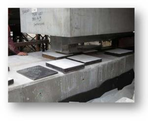
One slide mechanism is PTFE coated bearing pads with stainless steel slide shoes. Each pad is coated with dishwashing soap to further decrease the frictional forces; it is available, cheap, and effective.
