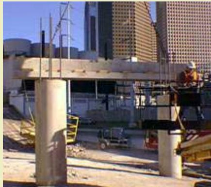
designers opted to speed construction by using precast bent caps on the existing columns. The bridge consists of twin structures, one northbound and one southbound, and each structure was completed in 95 days, a total of 226 spans
