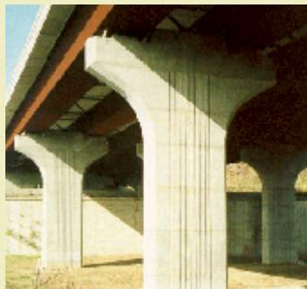
York State Department of Transportation accepted the contractor's value-engineering proposal to incorporate precast segmental voided pier sections for each of the 42 piers, which consisted of 8-foot match-cast segments vertically post-tensioned together and to the footings. It also changed the cast-in-place deck to 10-foot-long by 9-inch-thick precast panels, 42 to 50 feet wide to match longitudinal construction stages, supported on pairs of multi-span continuous steel tub girders.
