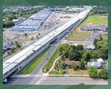
surroundings. The alignment was shifted, avoiding all commercial establishments, but remained viable to the business district. The project features include permanent count stations and a remote weather information system as well as an automatic anti-icing system on a ramp.
