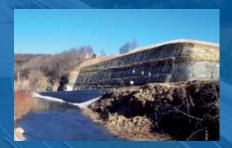
he Mae West Bend Project improved a sharp bend on Route 8 in Etna, PA. Due to its urban setting, the contractor was presented with a number of design and construction challenges including the restriction of blasting and realigning a road between a 100-foot high rock slope and a trout-stocked recreational stream in a commercial setting. Using a T-Wall (an interlocking retaining wall system), the contractor was able to minimize cost and time. This project met or exceeded all of PennDOT's needs,
