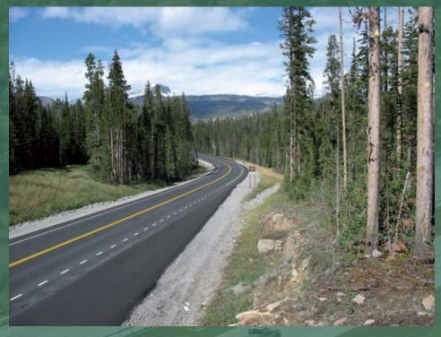
inconsistent and dangerous roadway geometry; and insufficient roadway width. The challenges were complex due to hydrologic, geologic, and climatic issues combined with high elevations and a short construction season. The new drainage structures were not designed for normal hydrology due to the previous forest fires, but instead were designed to accommodate heavy debris flow such as logs and
