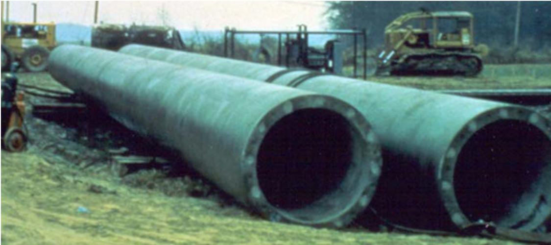
Figure 6-23 Concrete cylinder pile.
