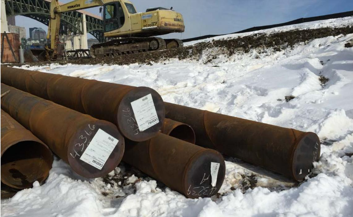
Figure 6-11 Typical 16 inch closed end pipe pile.
