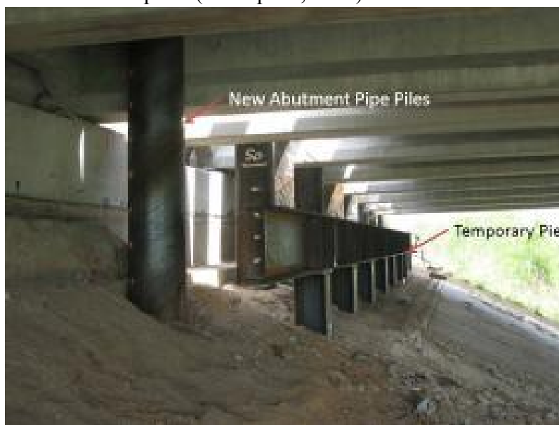
Figure A-18: Repairs and New Foundations (DeStephen, 2015)
