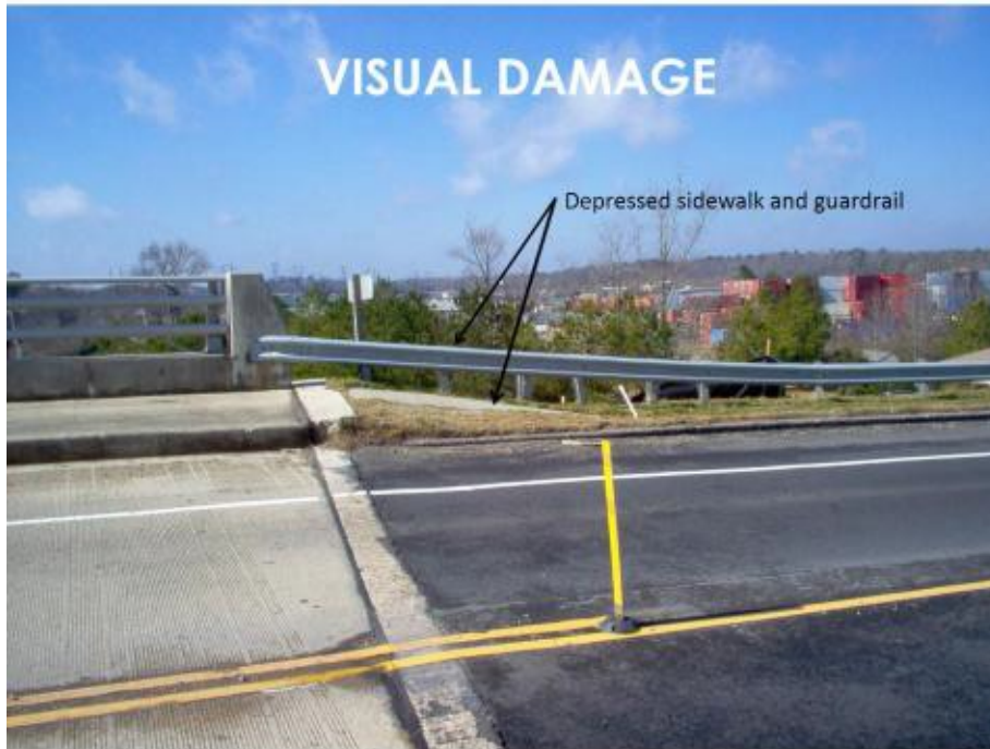
Figure A-16: Damage from Settlements (DeStephen, 2015)
