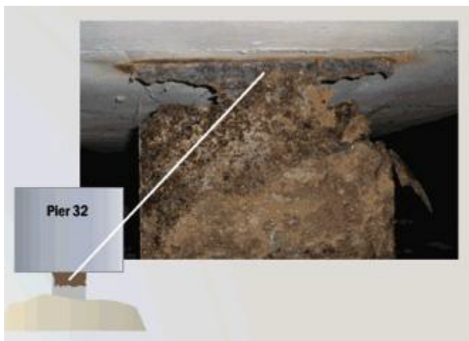
Figure A-14: Pile corrosion under Pier 32 (Paint Square, 2013)
